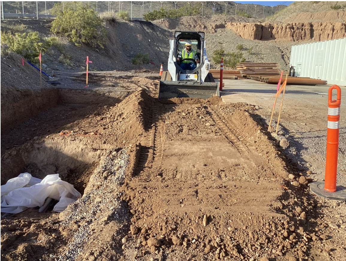
Photo showing backfill at Electrical Node 1.
