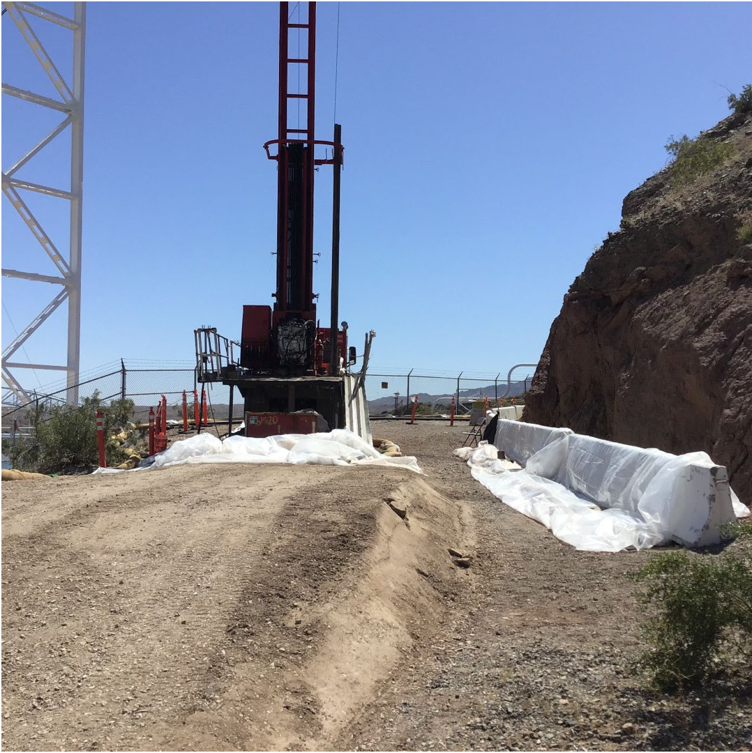
Photo showing drill rig on an earthen pad at ER-3.
