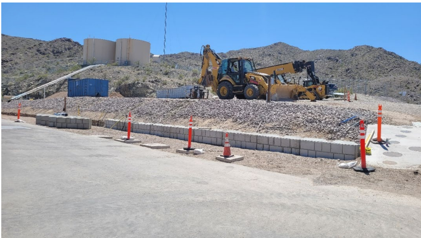
Photo showing installation of the concrete ecology block wall.
