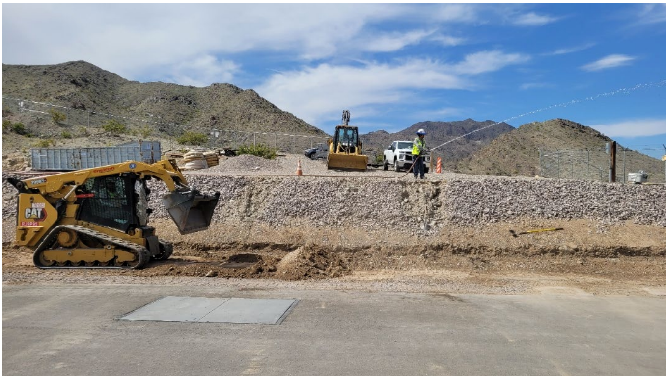
Photo showing excavation for the installation of a concrete ecology block wall south of TCS. This block wall replaces the wall removed during remedy construction in this area.
