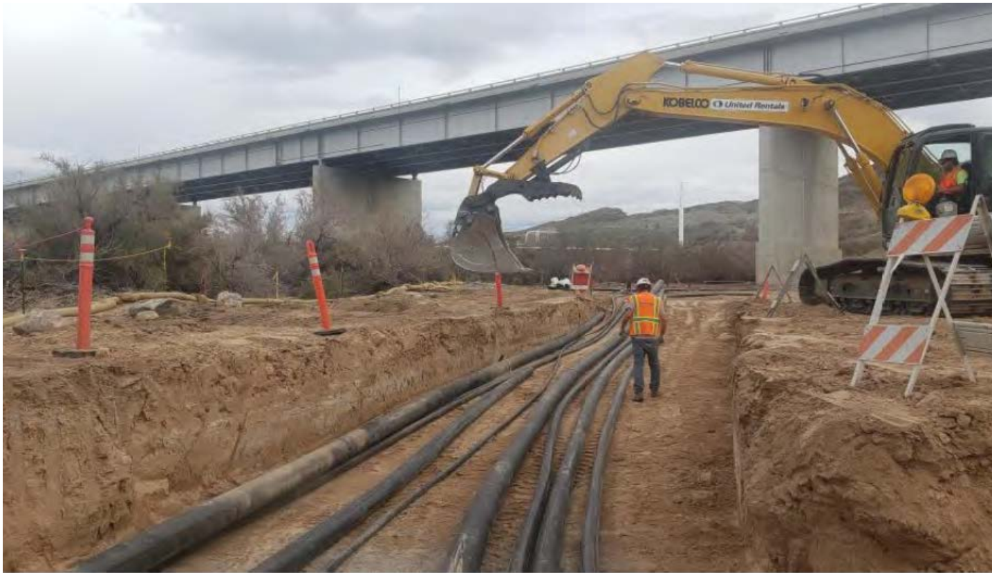
Photo showing pipe placement at C8 in the floodplain
