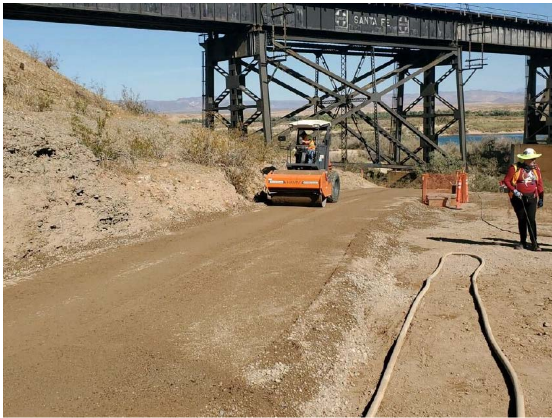
Photo showing compaction of access road on top of Pipeline C14
