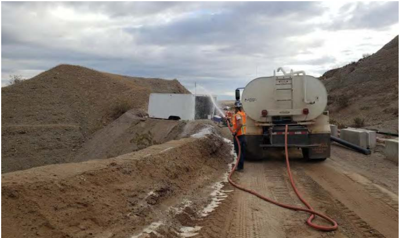
Photo showing application of SoilTac (a soil binder used for dust suppression) along Pipeline B
