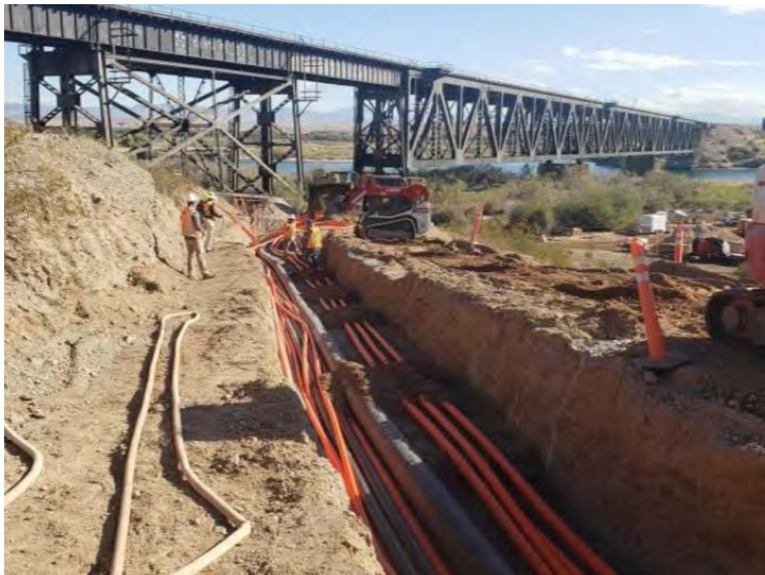
Photo showing sand shading and stacking of conduits along Pipeline C14
