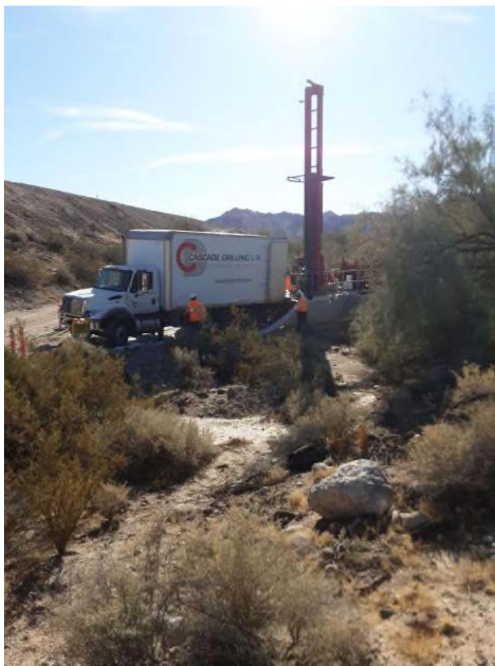
Photo showing drill rig at Hydro-6 drill site
