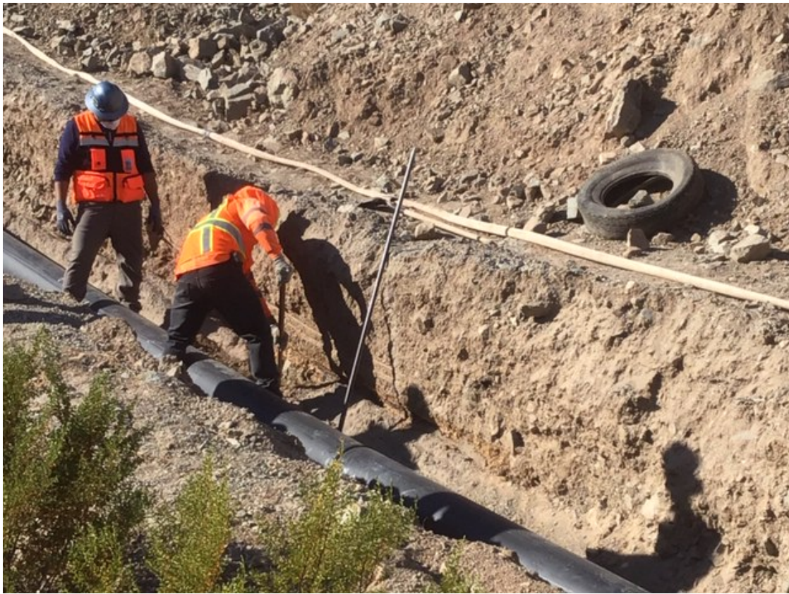
Photo showing preparation for sampling of stained soil encountered in the westernmost reach of Pipeline B
