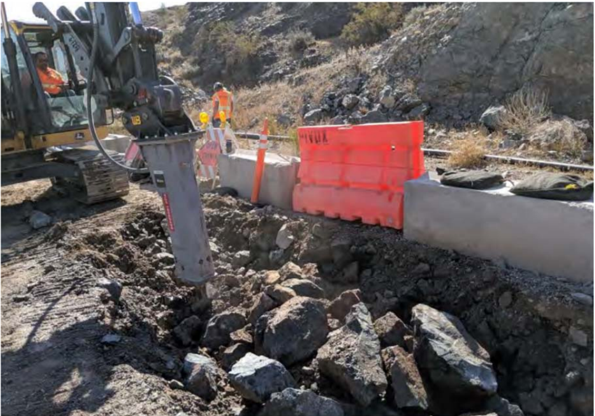
Rock breaking at Pipeline B
