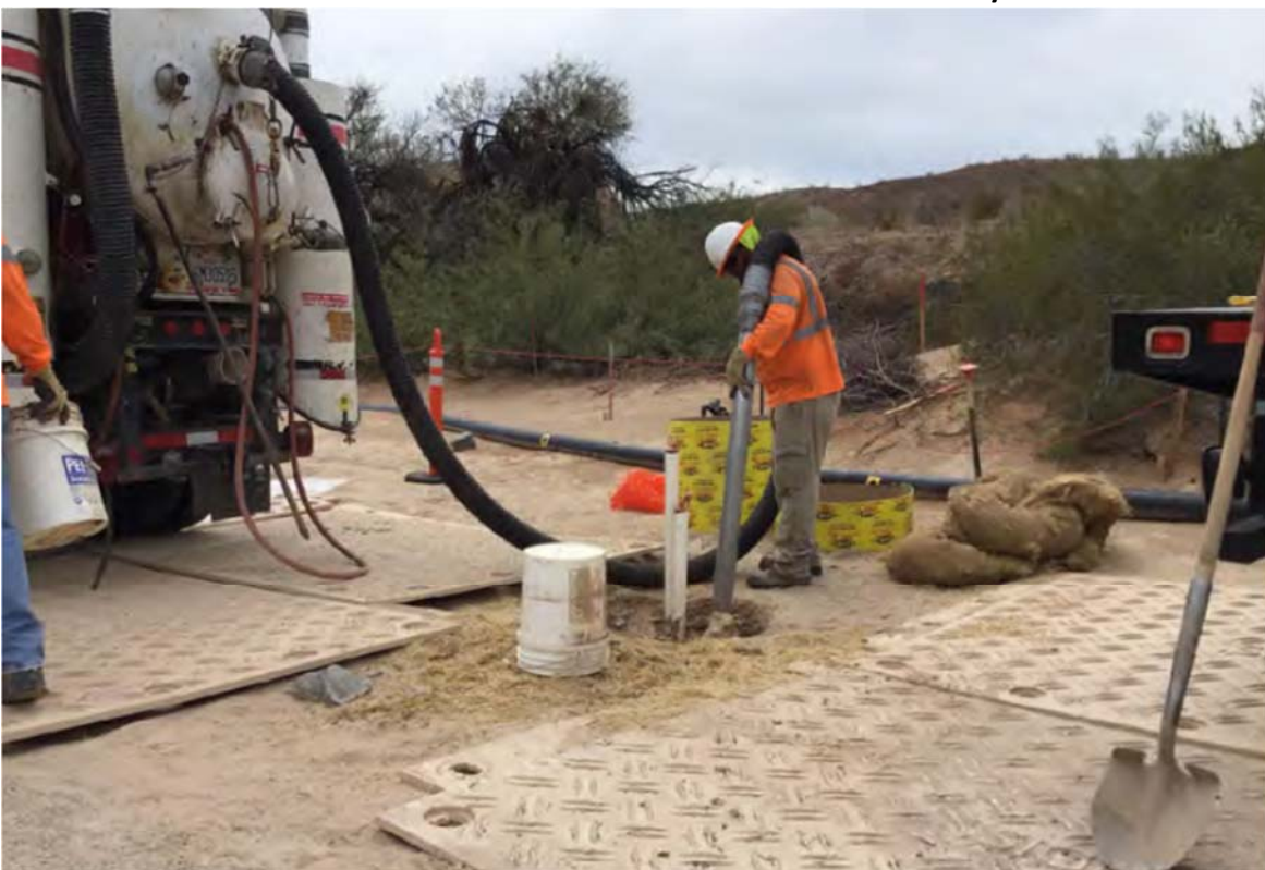
MW-C – Airvac of borehole
