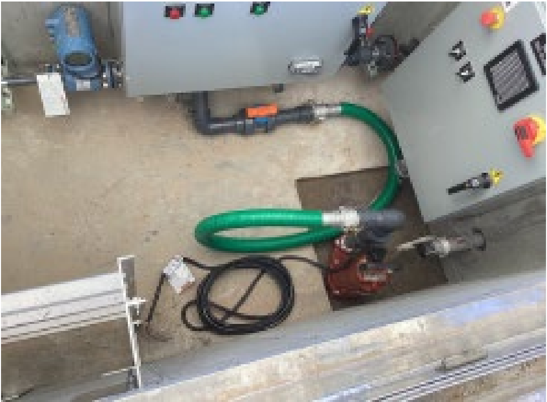
Photo showing sump pump installation in vault RB-5.
