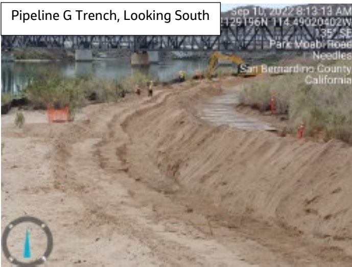
Installation of HDPE piping and conduits in Pipeline G Trench
