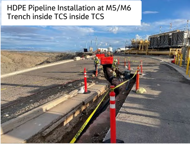
Sand Bedding Placement in Pipeline M6
