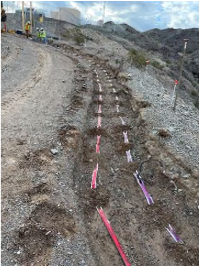
Backfill at Pipeline L inside TCS
