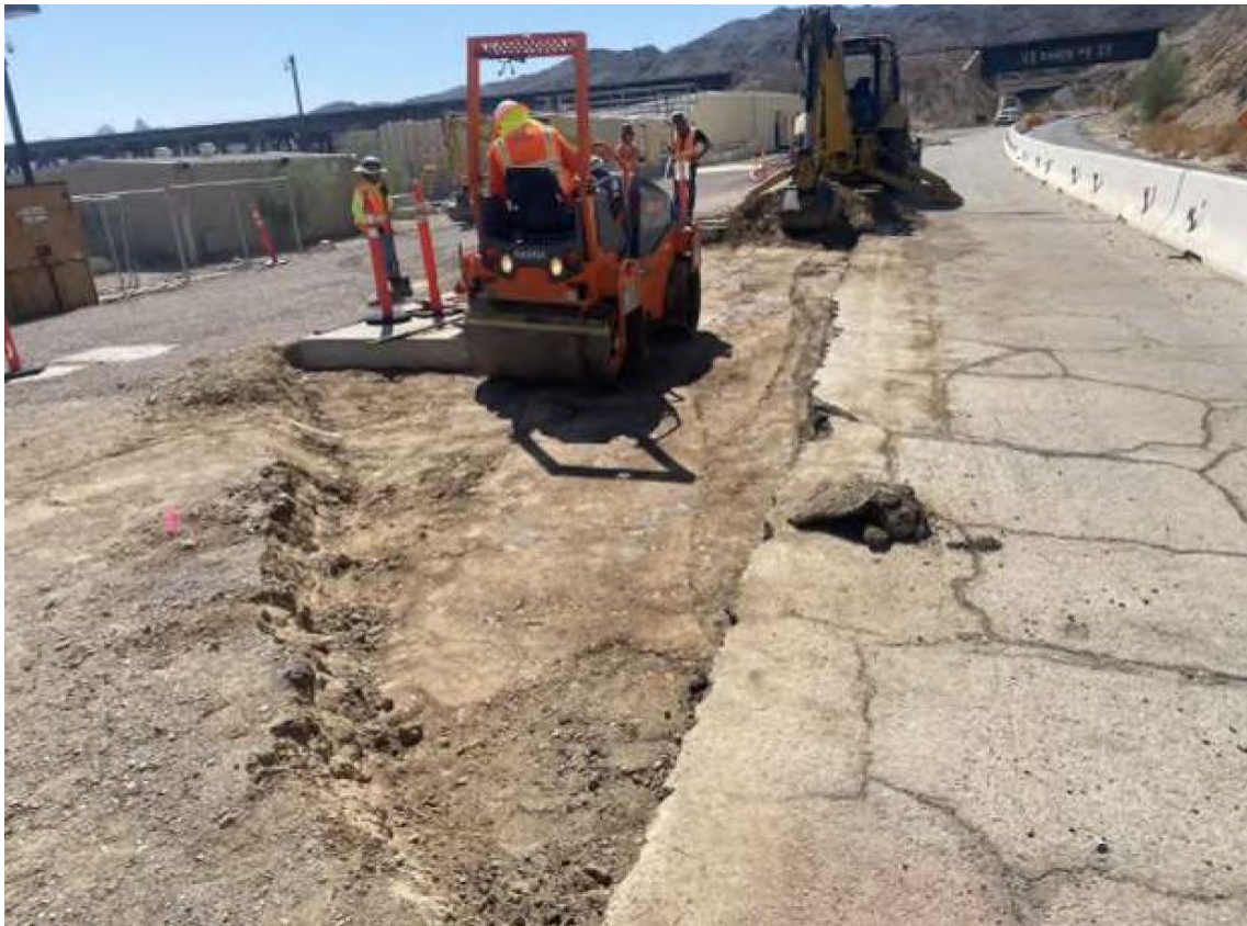
Photo showing excavation around IRZ-21 well vault in preparation for the asphalt paving.
