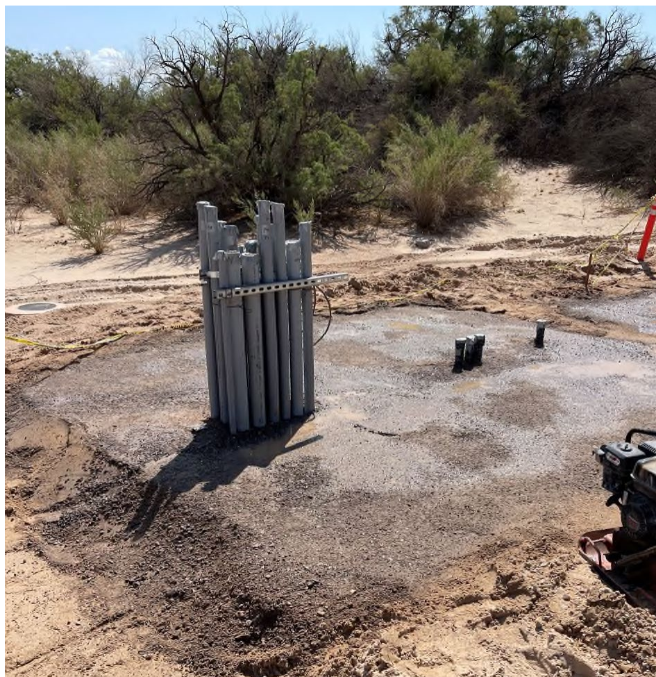
Photo showing concrete pad preparation at Electrical Node 4.
