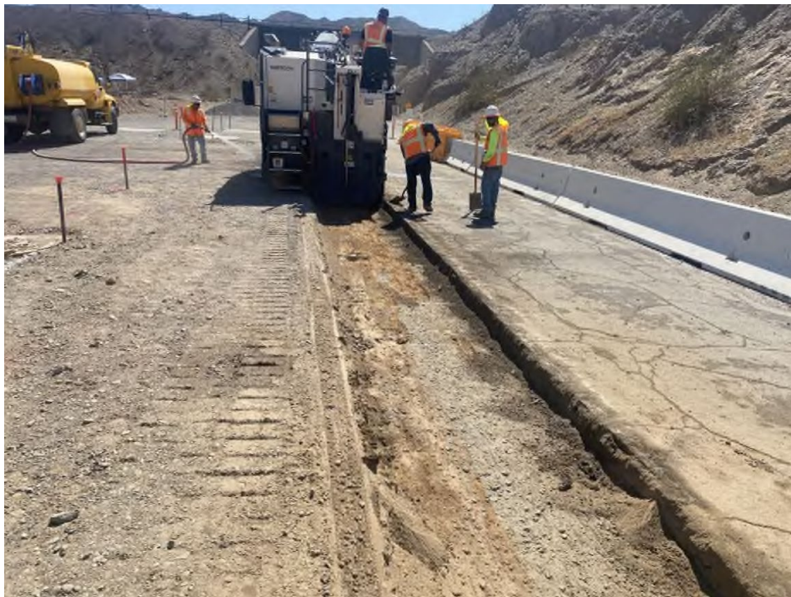
Photo showing milling existing asphalt at MW-20 Bench.
