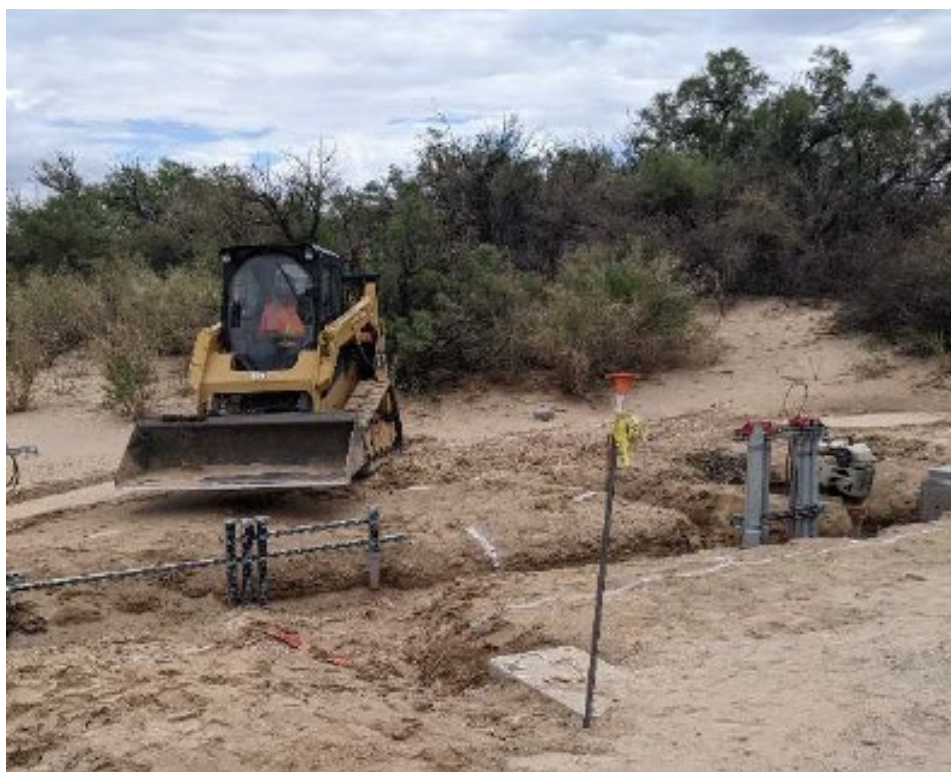
Photo showing grading in preparation for concrete pad installation at Electrical Node 4.
