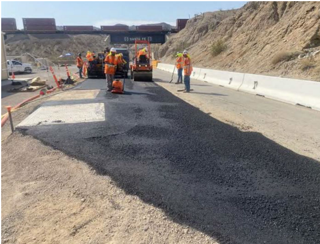
Photo showing asphalt installation around vaults.
