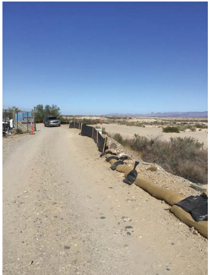
Construction Stormwater pollution prevention measures at MW-20 Bench
