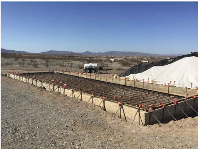
Truck containment pad at TCS ponds
