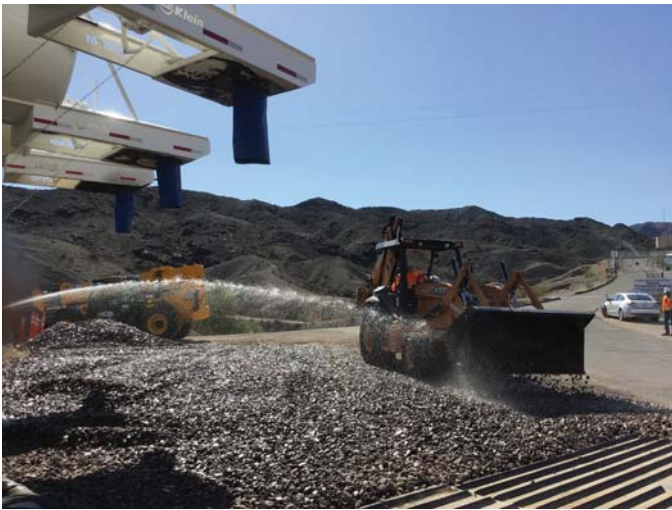
Dust control by watering
