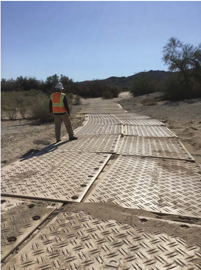
Soil stabilization mats in the floodplain to facilitate access
