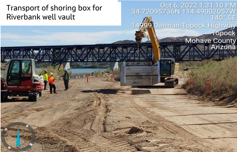
Shoring box placed at well RB-4
