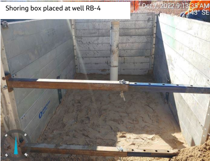
Completed excavated bottom ready for fabric and gravel placement
