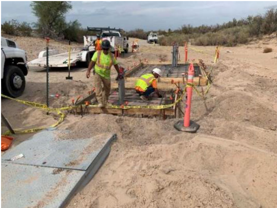
Photos showing rebar placement and tie at Electrical Nodes 4 (top) and 2 (bottom).
