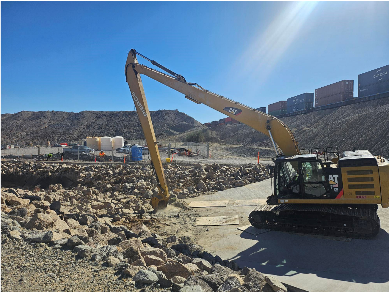
Photo showing maintenance repair of riprap at the Construction Headquarters (CHQ).
