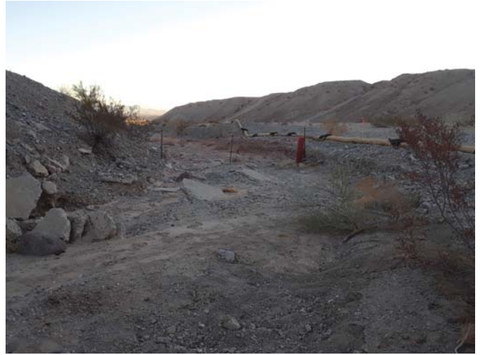
Installation of snow fence to delineate the maximum construction footprint in the jurisdictional water (wash) at the CHQ
