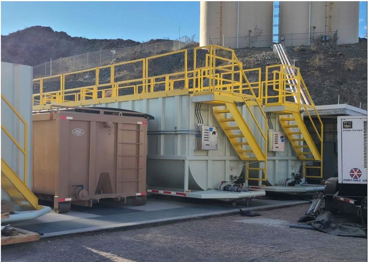
Photo showing the remedy-produced water conditioning (RPWC) system tank farm.
