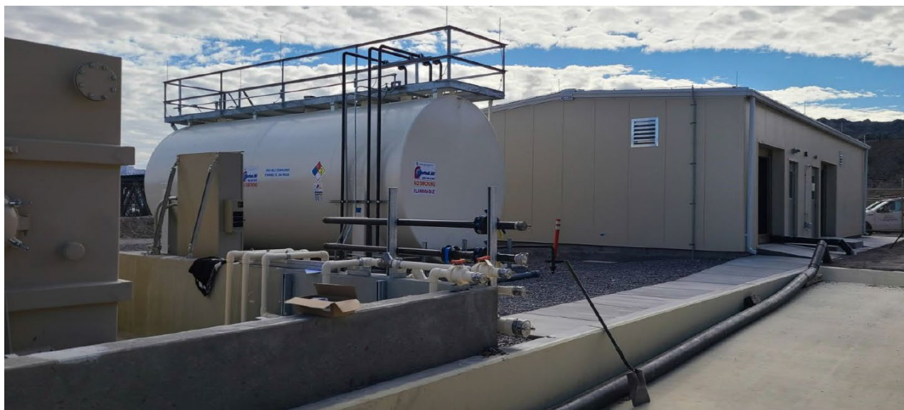
Photo showing the ethanol storage tank and Carbon Amendment Building on the MW-20 Bench.
