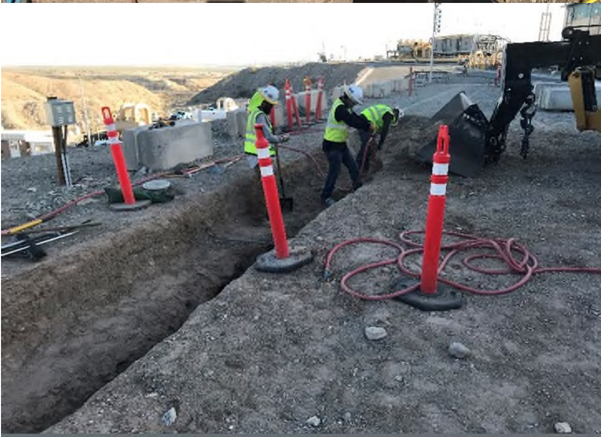
Photos showing hand excavation for installation of remedy pipelines I1 (top) and M6 (bottom) inside TCS
