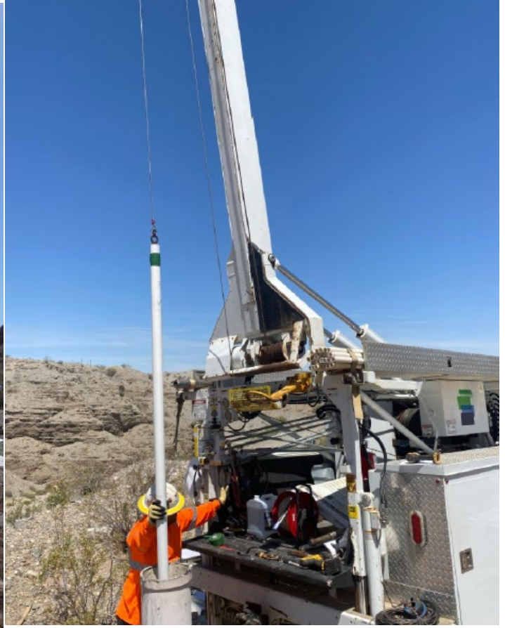
Photos showing pump being pulled at PGE-07BR
