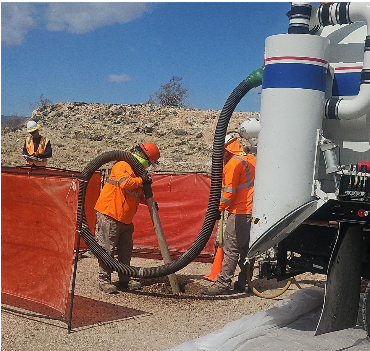
Photo showing air knifing at well IRL-3.
