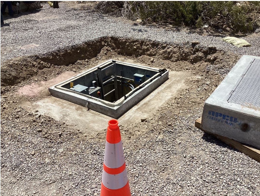
Photo showing excavation around well IRZ-18 in preparation for raising vault lid.
