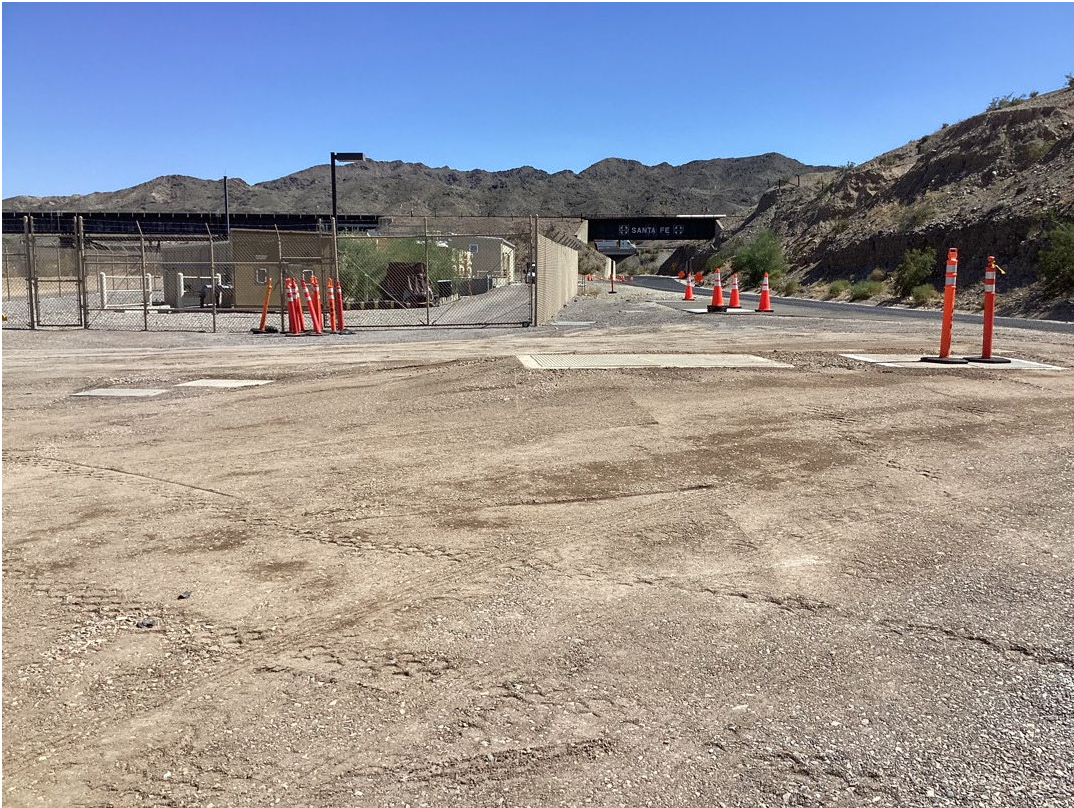
Photo showing final grade around IRZ-23 well vault after the vault lid was raised.
