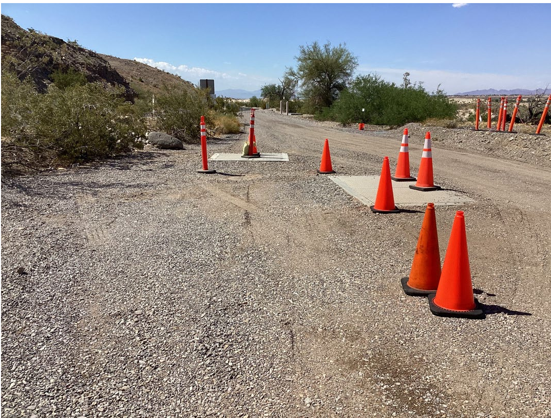
Photo showing final grade around IRZ-18 well vault after its lid was raised.
