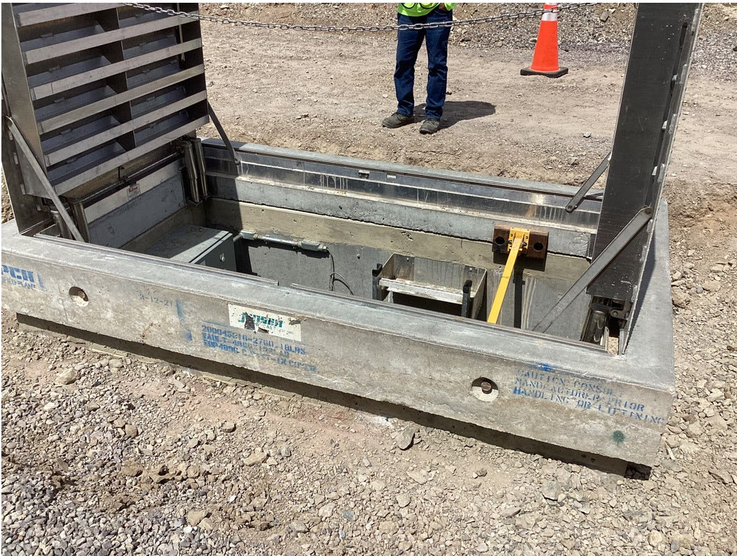
Photos showing the IRZ-18 vault lid installation
