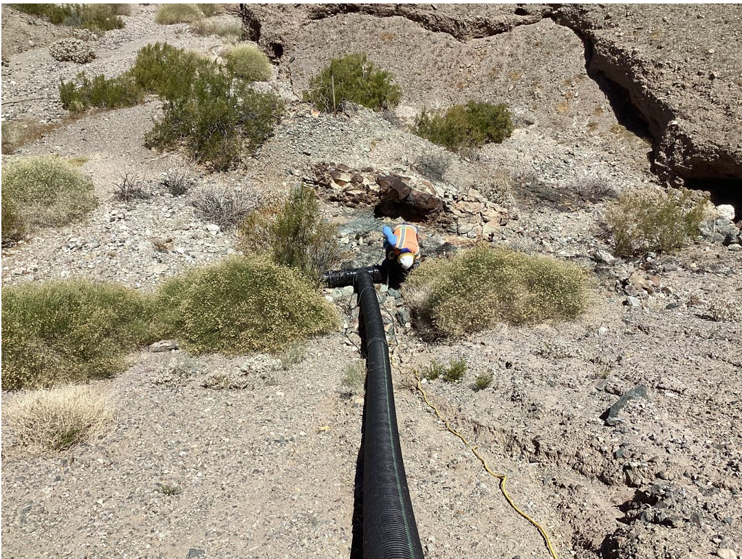
Photo showing installation of anchors to secure the drain pipe from Pipeline B access road.
