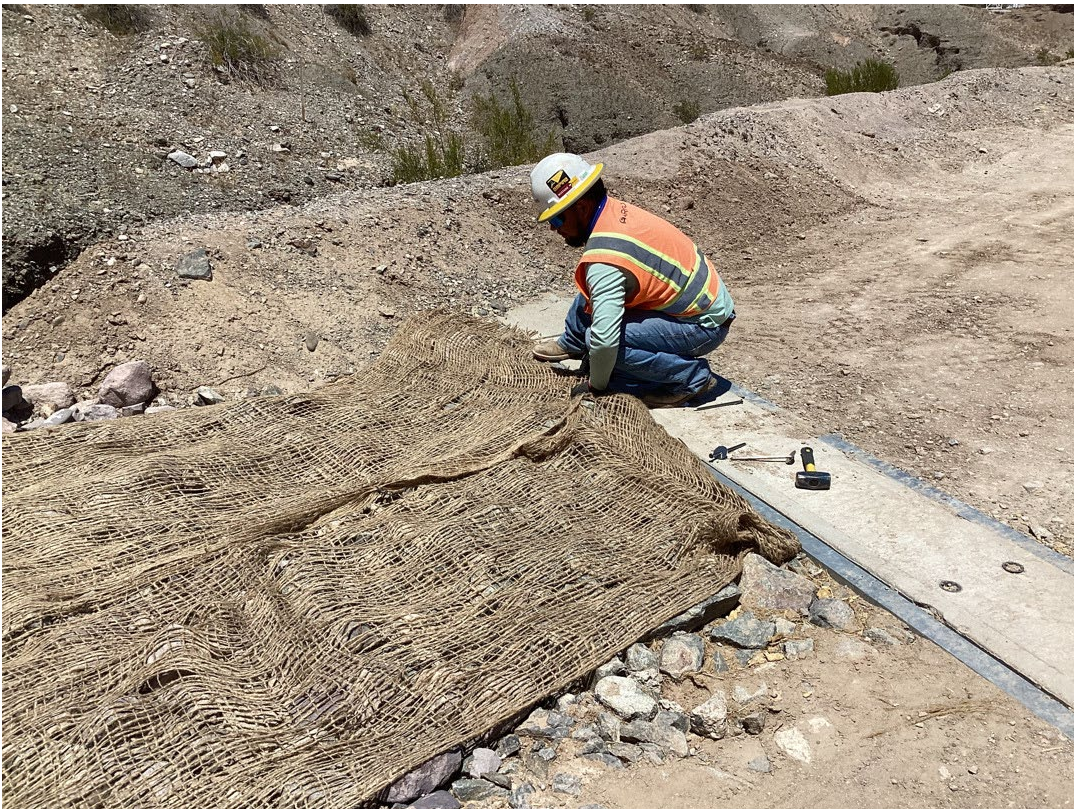
Photos showing installation of coir mats for slope erosion control.
