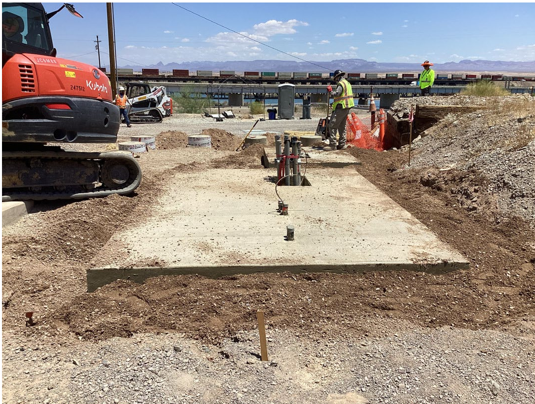
Photo showing Electrical Node 1 backfill and compaction.
