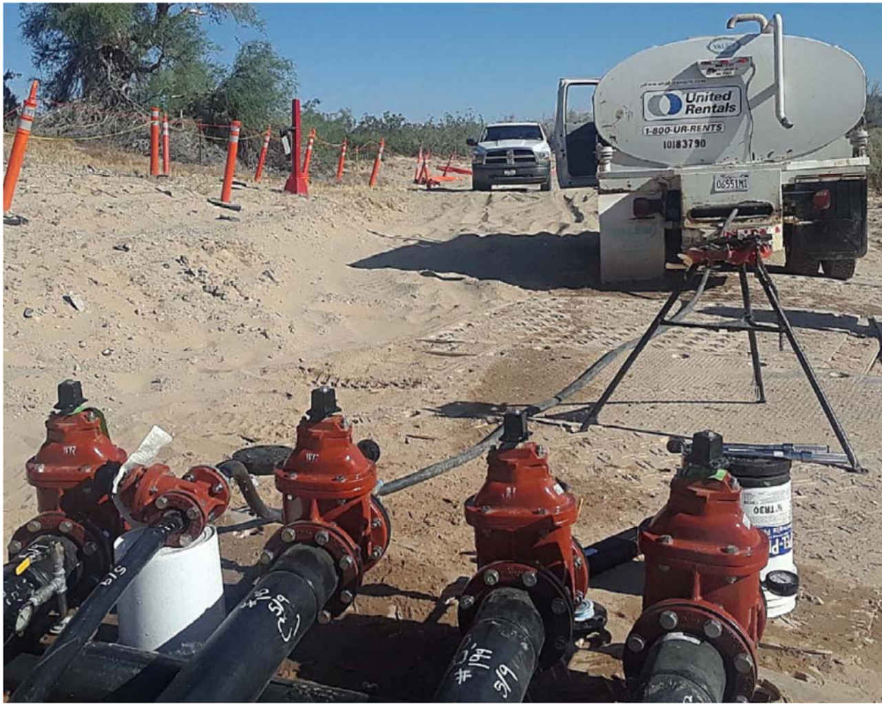
Hydrostatic testing fill point at the beginning of Pipeline C Segment C3
