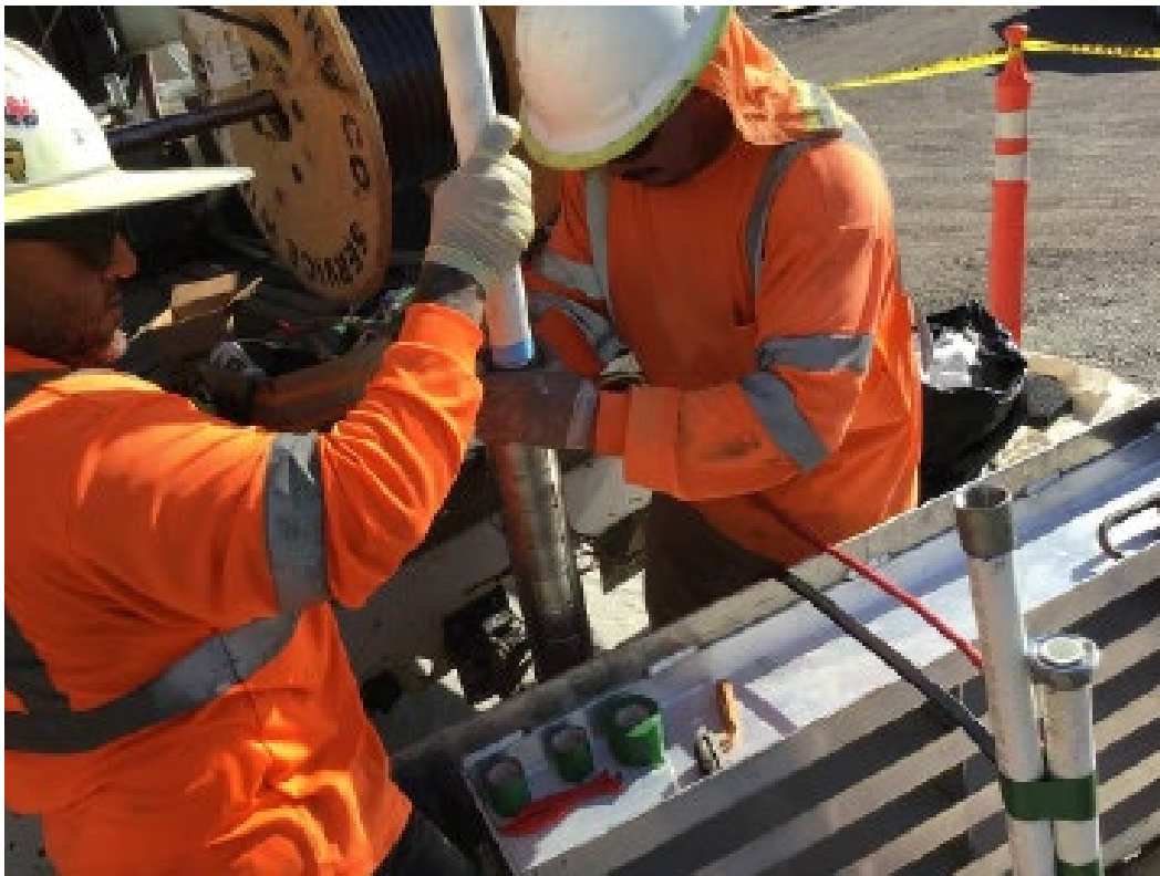
Photo showing Cascade installing shallow pump at IRZ-25.
