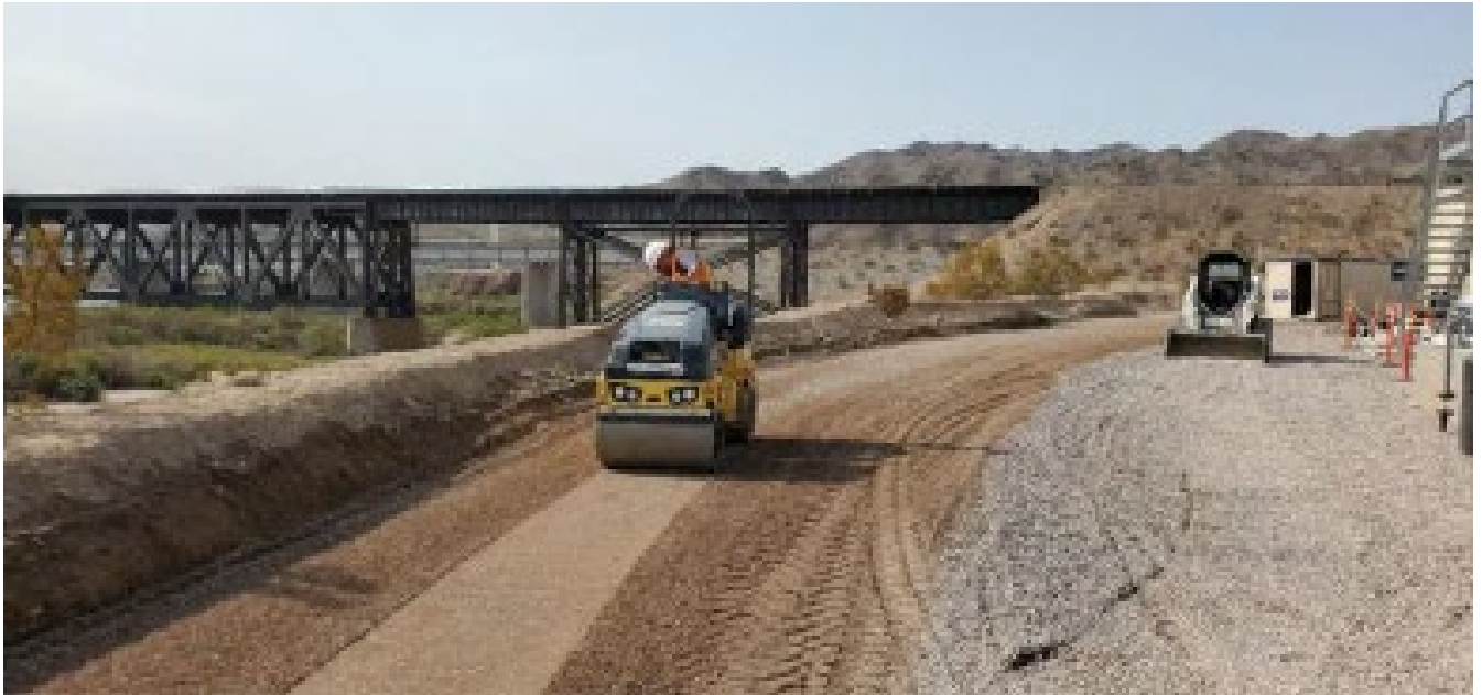
Photo showing compacting on the river side of MW-20 Bench.
