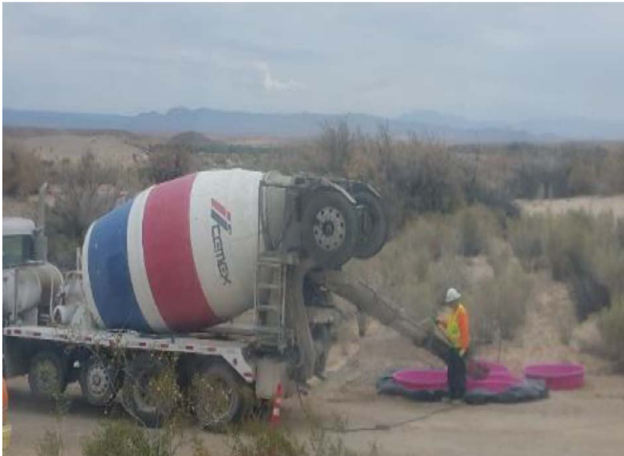
Wash out of slurry mix into the secondary containments in the floodplain
