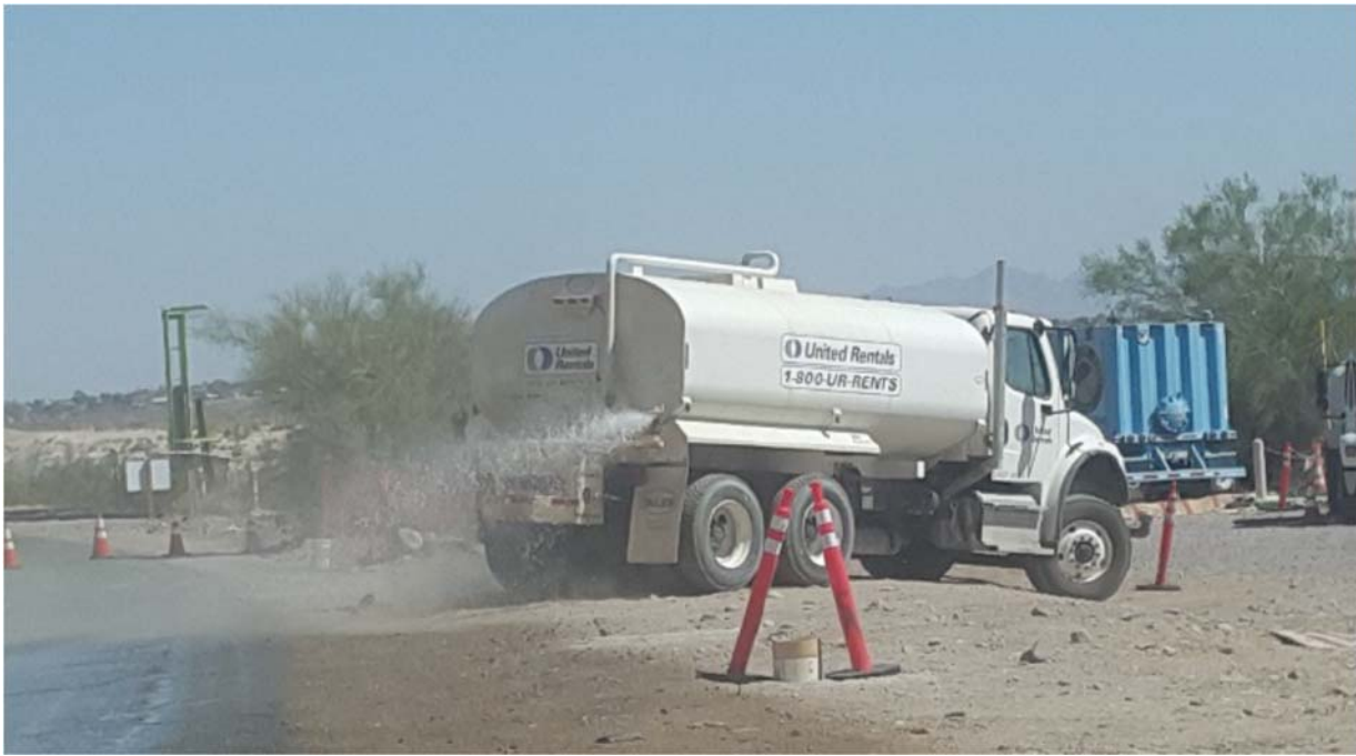
Applying water at MW-20 bench for dust control
