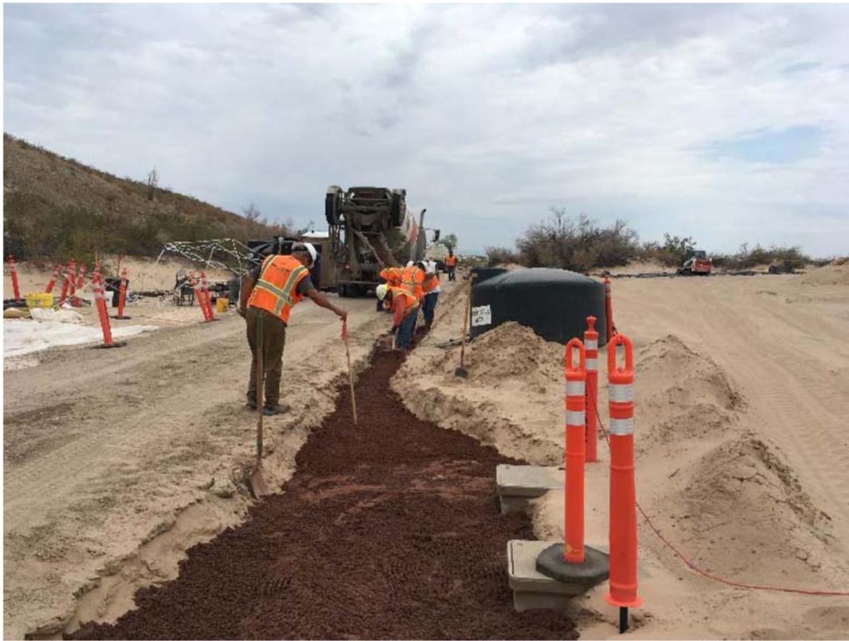
Placement of red slurry warning layer over electrical trench along Pipeline C Segment C3
