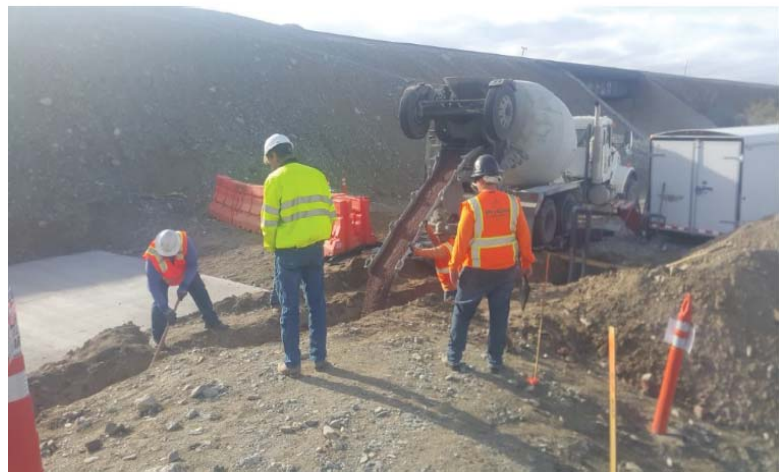
Pour slurry concrete at CHQ access road (photo taken on 1/7/19)
