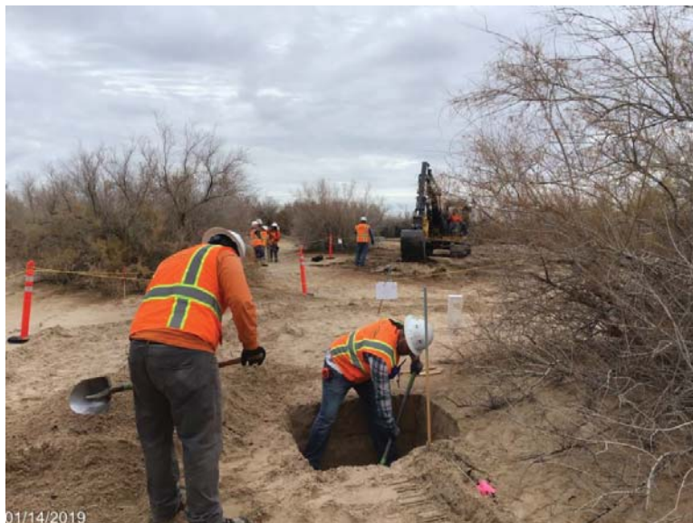
Potholing in C5 segment (photo taken on 1/14/19)
