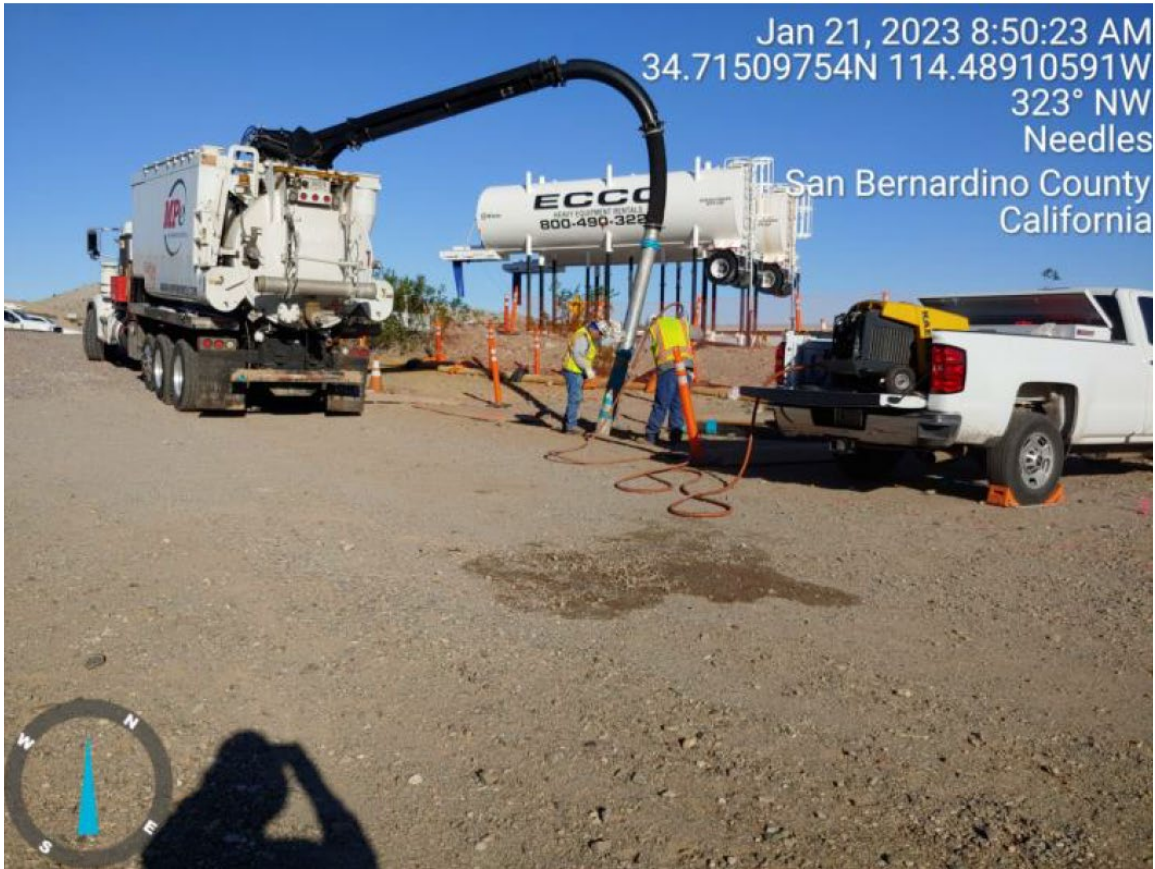
Photo showing vacuum excavation potholing for Pipeline C11 on east side of National Trails Highway
