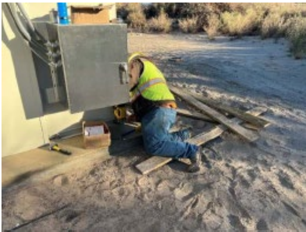
Photo showing transformer anchor installation at Electrical Node 4 in the floodplain.
