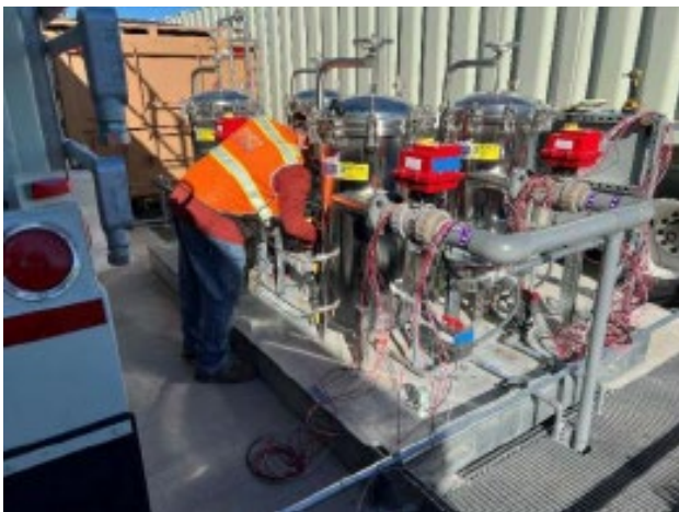
Photo showing wire termination at the Remedy-produced Water Condition (RPWC) system.
