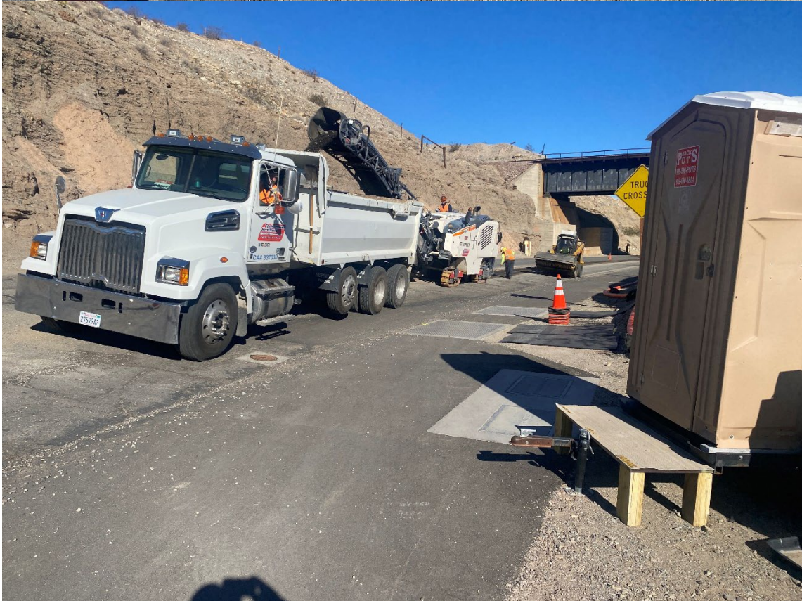
Photo showing road repair from K-rails pins strike.
