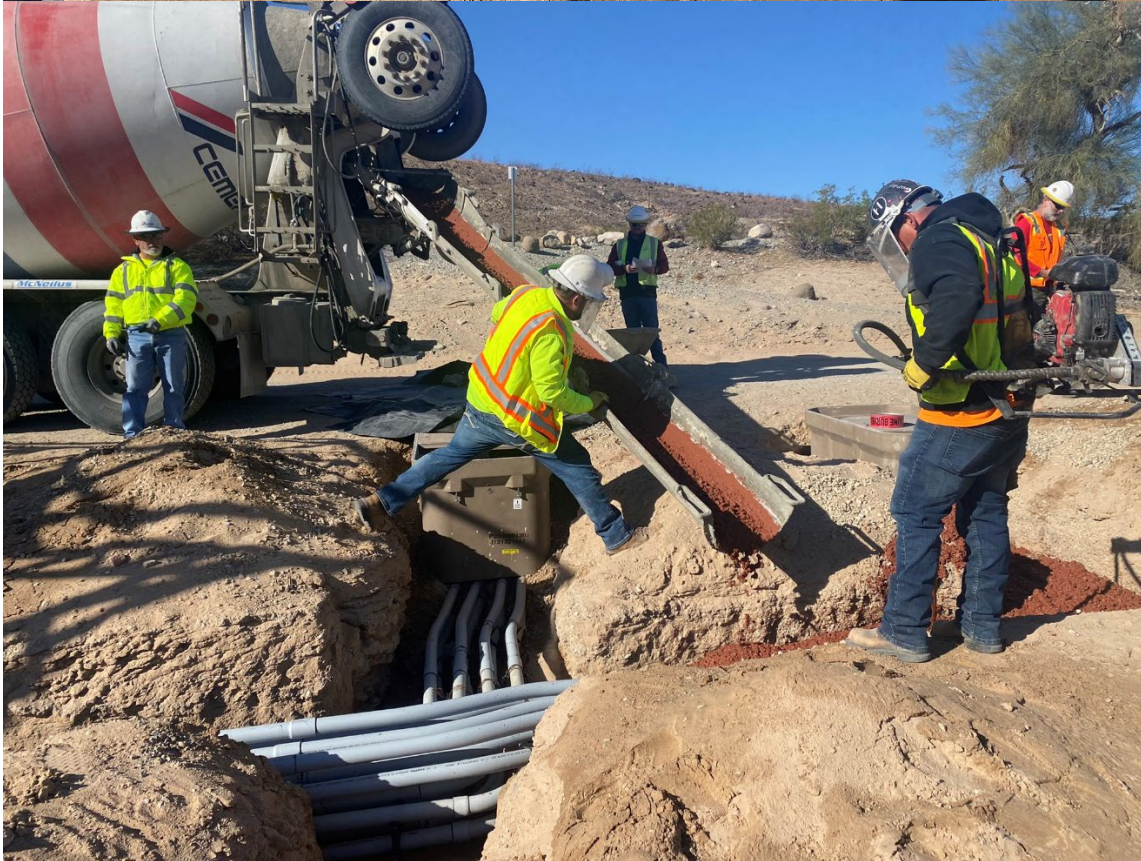
Photos showing slurry pour at Electrical Node 4 in the floodplain.
