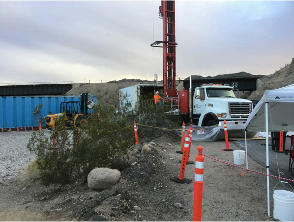
IRZ-25 sonic drilling (photo taken on 12/11/18)
