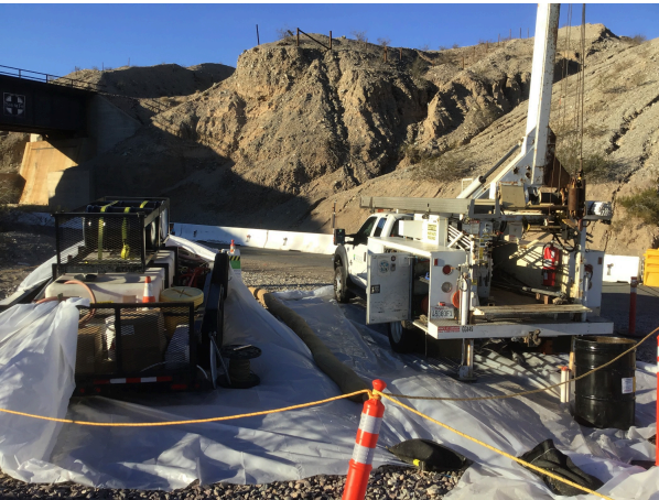
Well development at MW-E (photo taken on 12/13/18)
