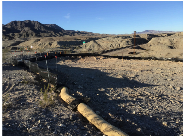
SWPPP BMPs (silt fence and fiber rolls) at MW-N well location (photo taken on 12/13/18)
