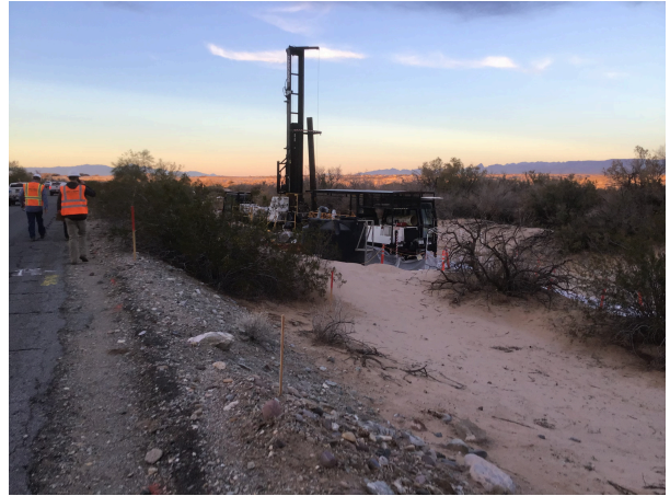
IRZ-9 sonic drilling (photo taken on 12/11/18)
