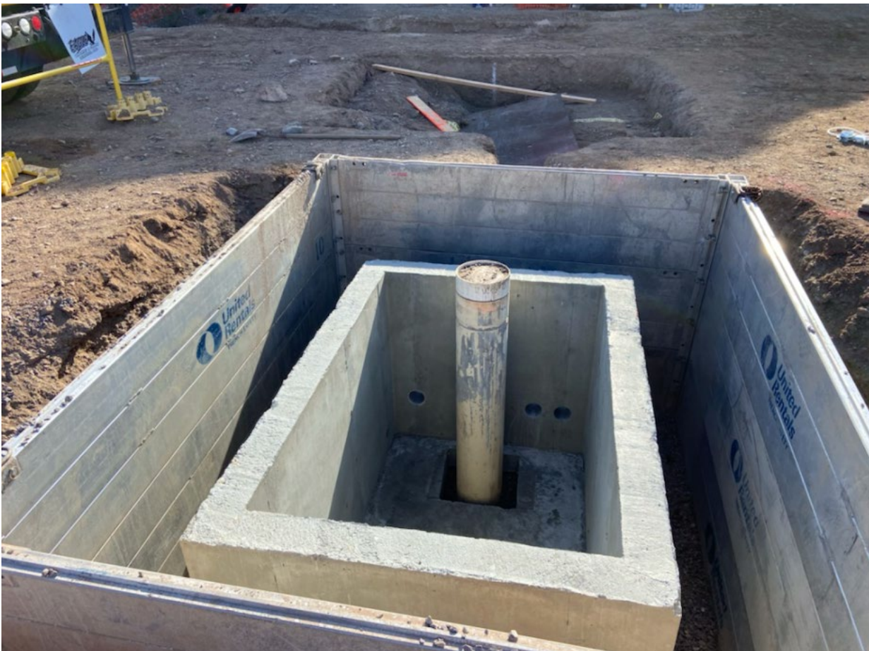
Photos showing the excavation for Installation of TWB-3 well vault
