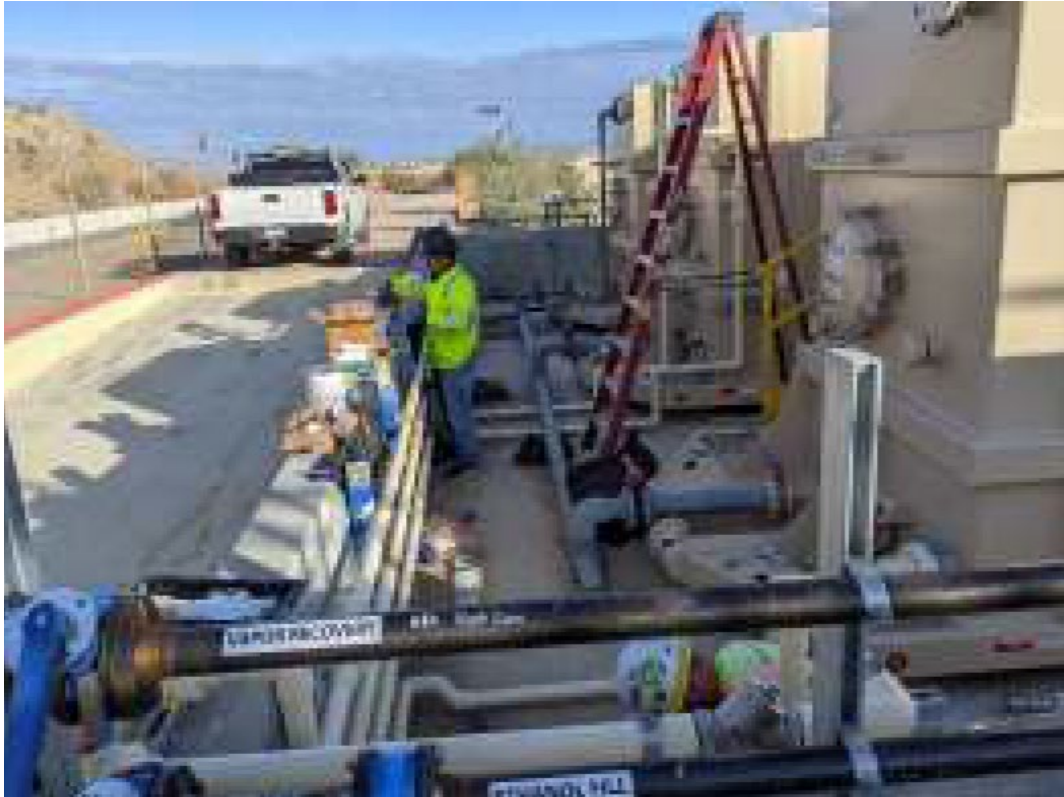
Photo showing pipe painting at the MW-20 Bench Frac Tanks
