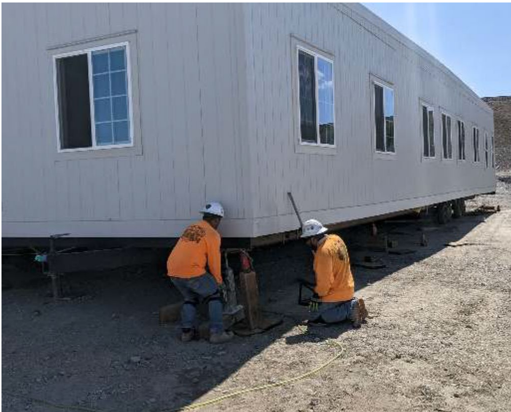
Photo showing installation of new trailer at SPY.
