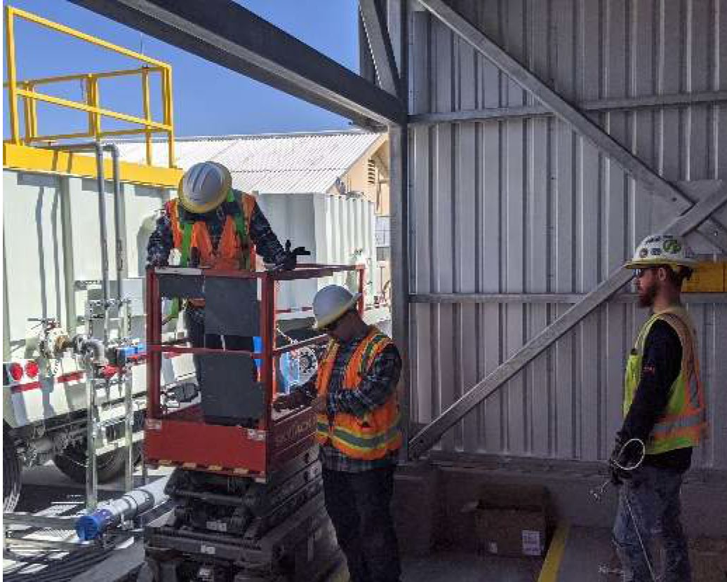
Photo showing removing front of switch gear canopy.
