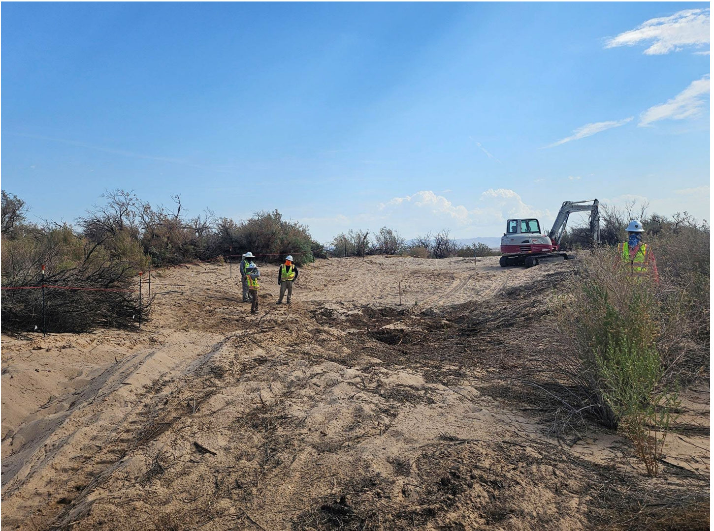
Photo showing grading and vegetation removal at MW-JJ in the floodplain.
