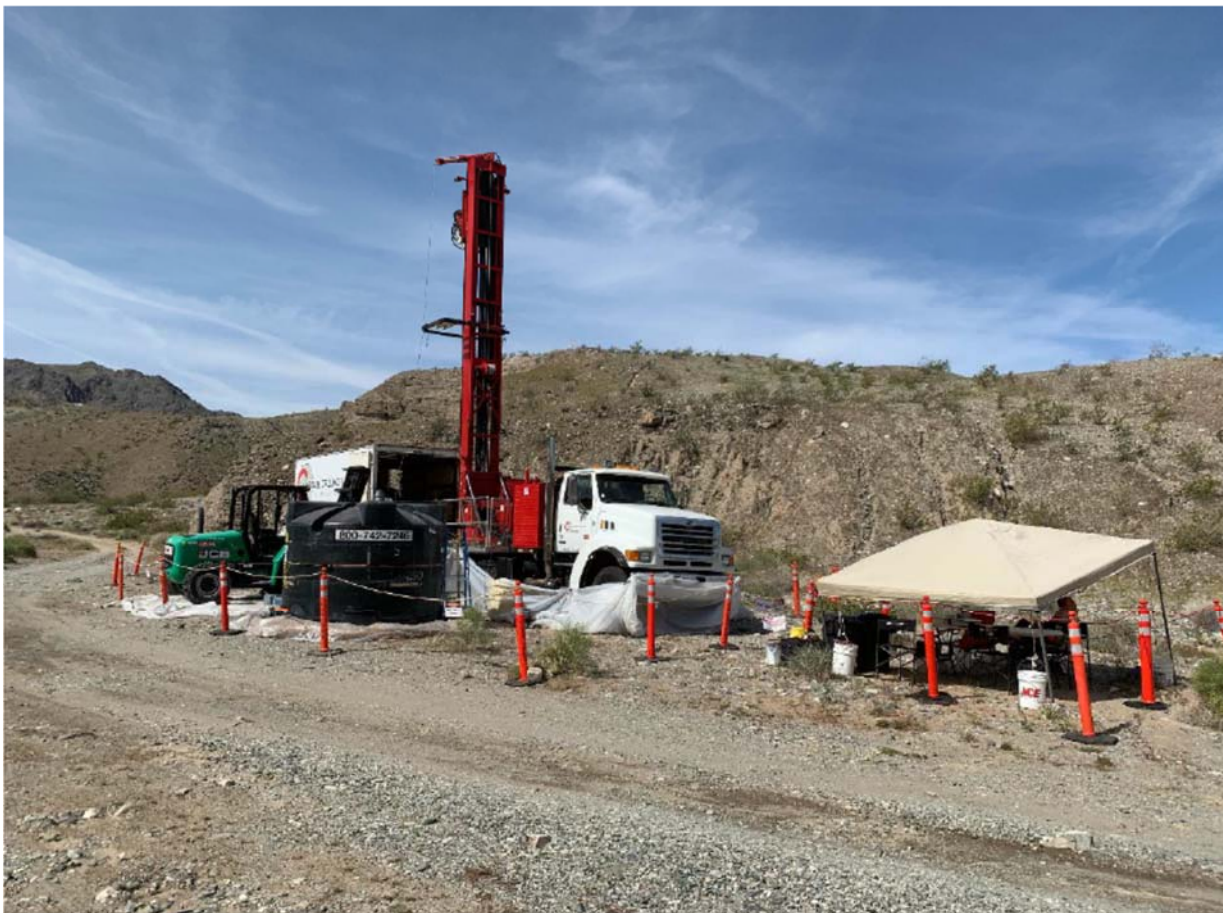
Sonic Rig at MW-10 D in Bat Cave Wash
