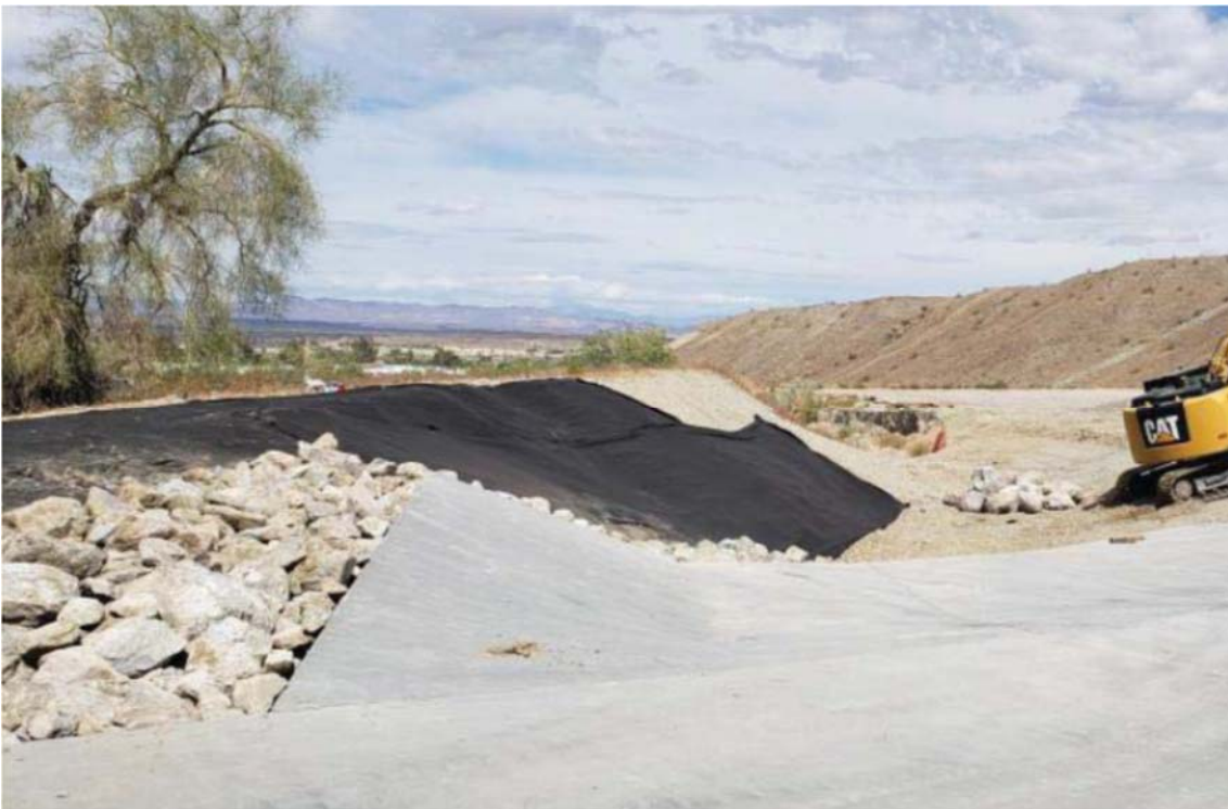
Installation of Geofabric and RipRap at the CHQ
