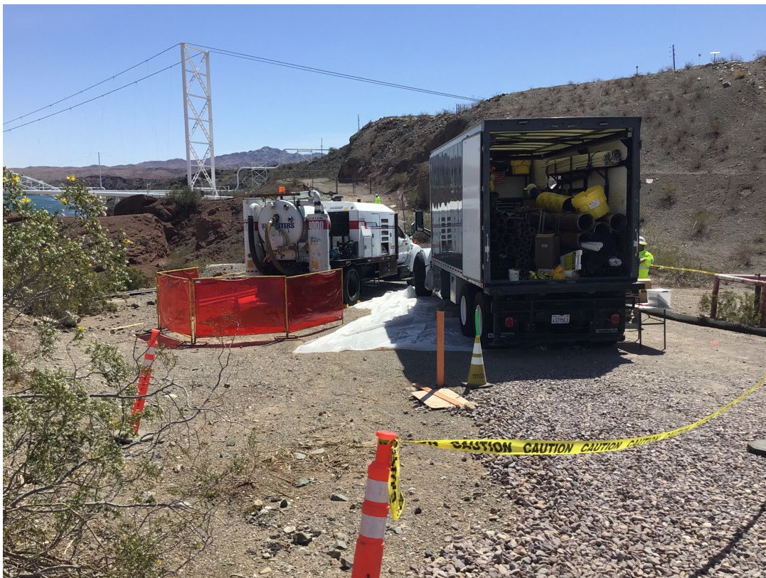
Photos showing potholing at TCS-1 and ER-1 drilling locations.
