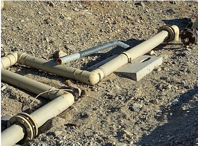
Photograph 13: Injection well control conduit removal example.
