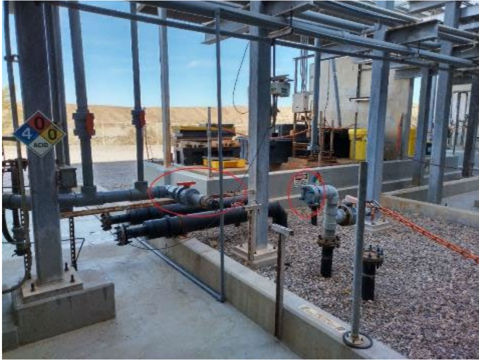
Photograph 10: Injection line isolation at IM-3 after dismantling and cleaning [facing southeast].
