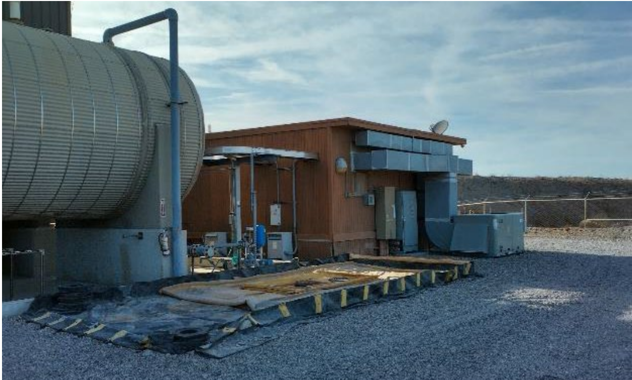
Photograph 18: Emergency diesel generator pad after generator removal.
