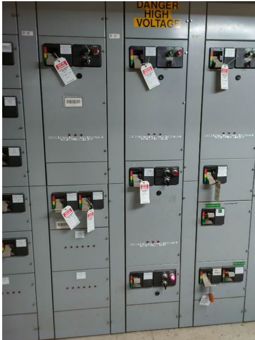
Photograph 9: Extraction Well MCC tagout.
