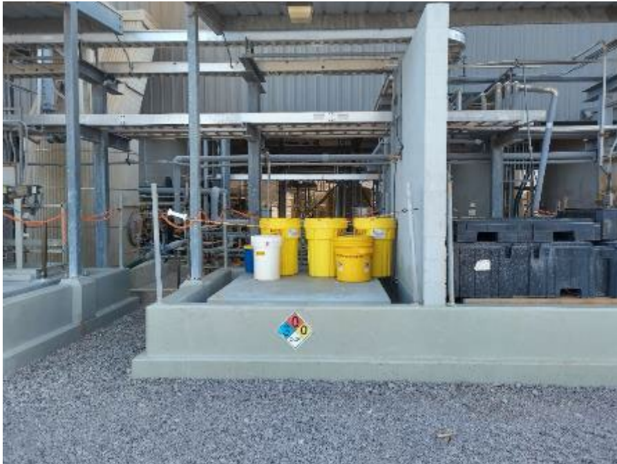
Photograph 28: Caustic Storage Area 1 after dismantling and cleaning.
