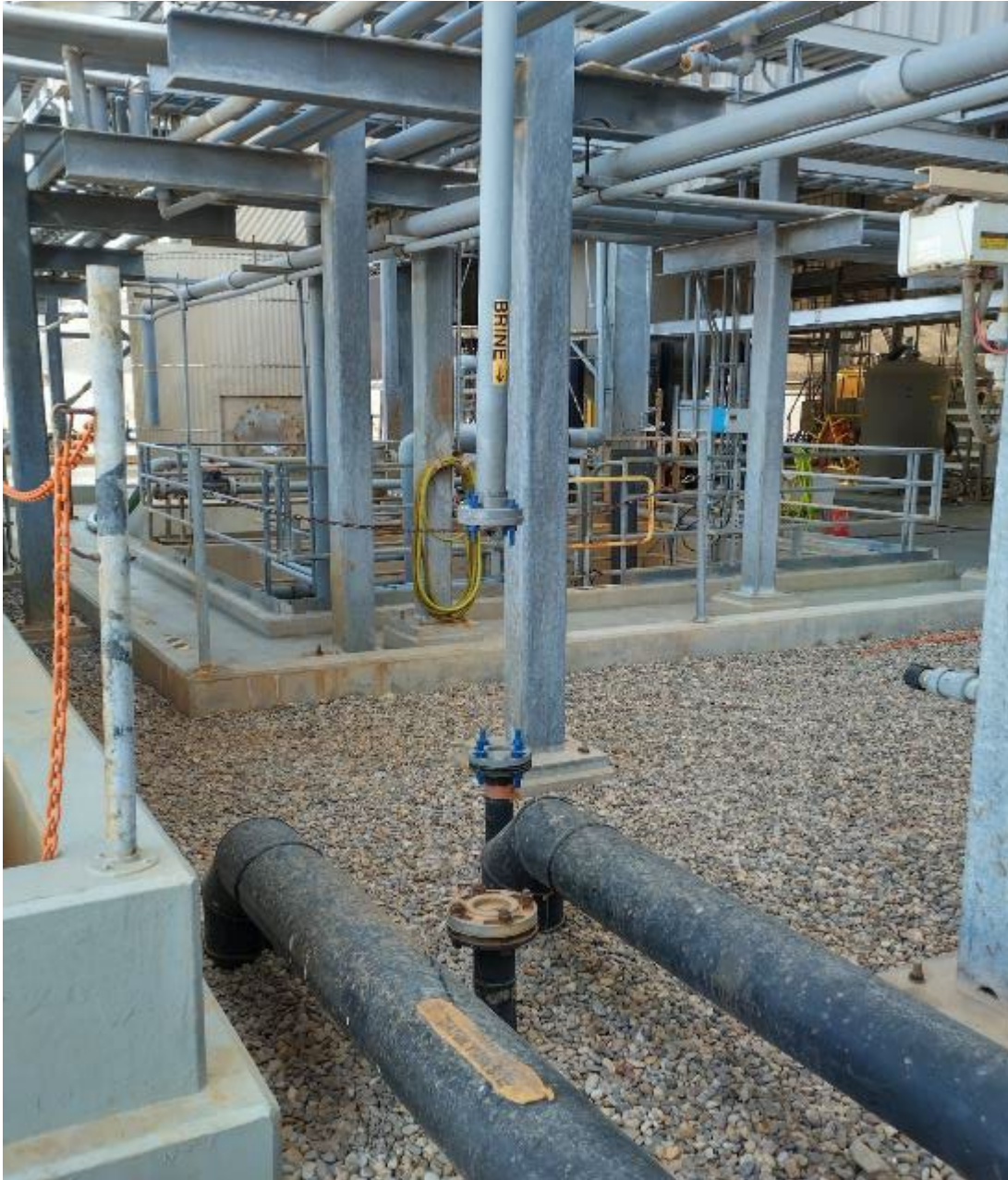
Photograph 12: Brine line isolation at IM-3 after dismantling and cleaning [facing southwest].
