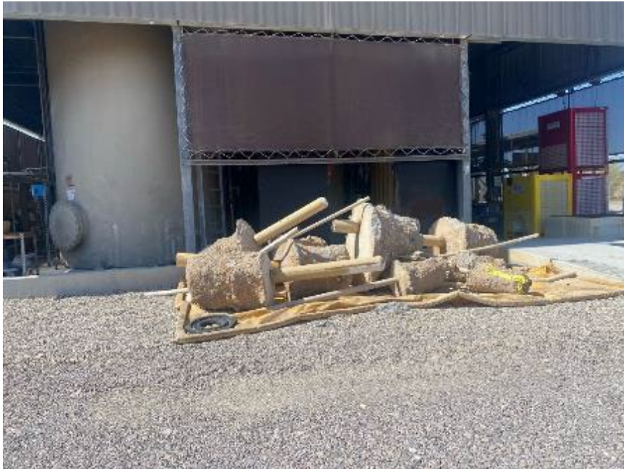
Photograph 37: Injection Well Control system bollards after removal.
