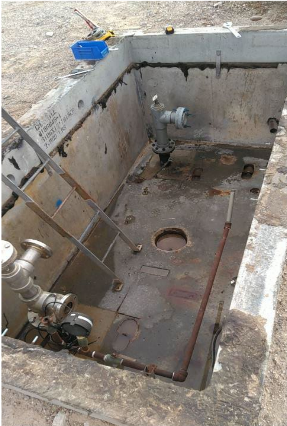
Photograph 15: Injection well vault example after line blinding and vault cleaning.
