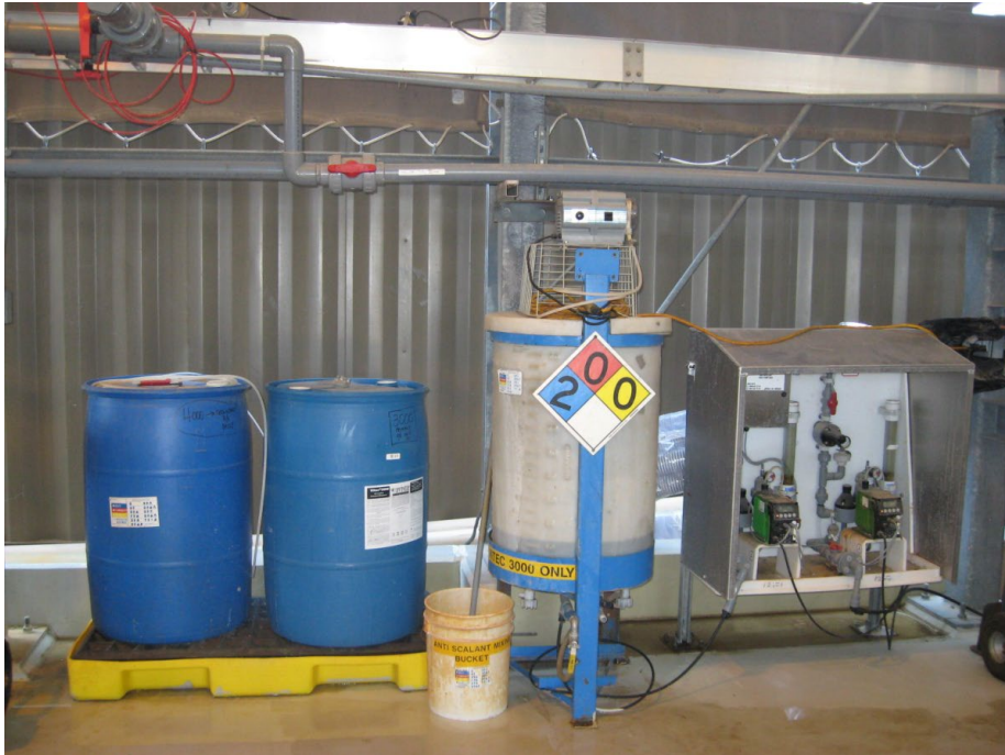
Photograph 32: RO Antiscalant Storage Area prior to dismantling and cleaning, frontal view (CH2M, 2014).
