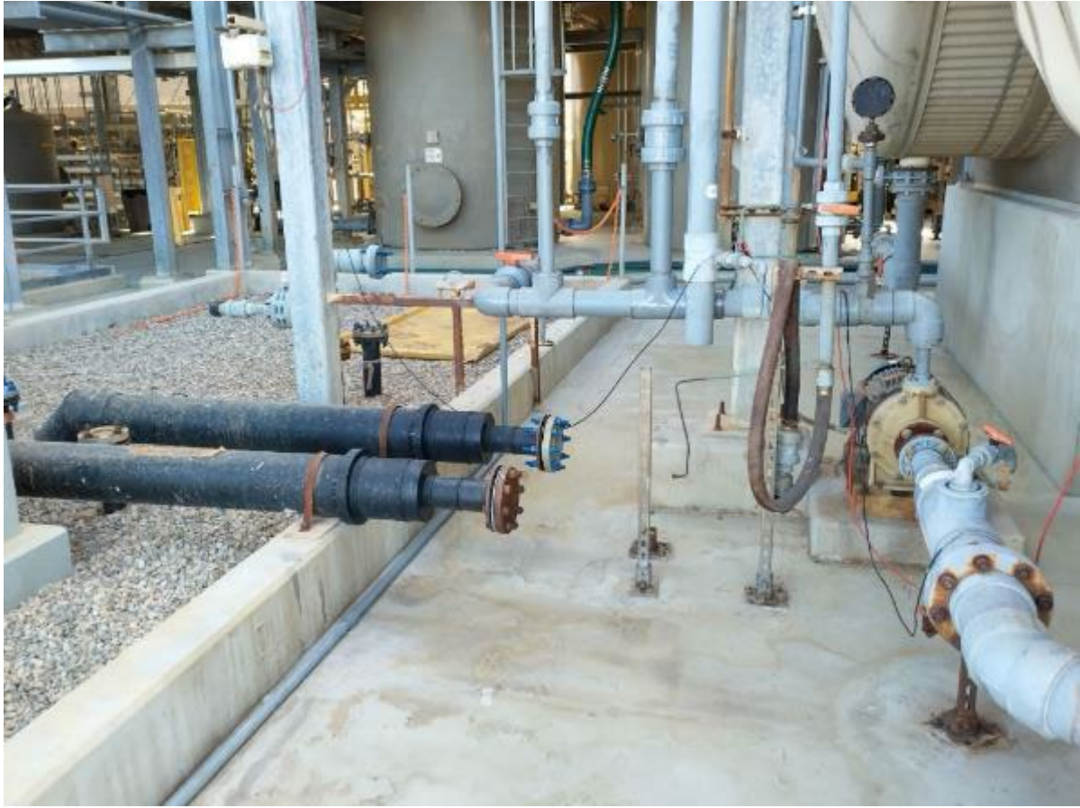
Photograph 8: Extraction Line isolation at IM-3 after dismantling and cleaning [facing west].
