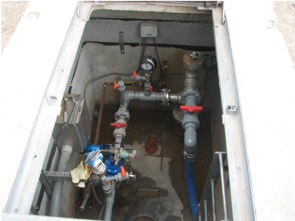
Photograph 14: Injection well vault example before dismantling and cleaning (CH2M, 2014).
