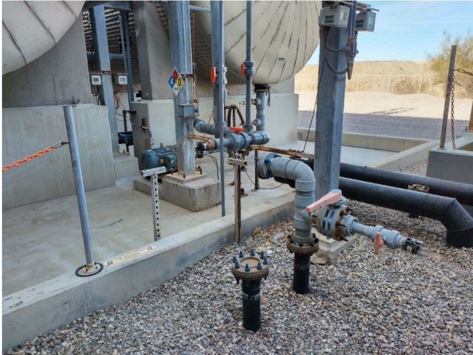
Photograph 11: Off-spec water line isolation at IM-3 after dismantling and cleaning [facing east].
