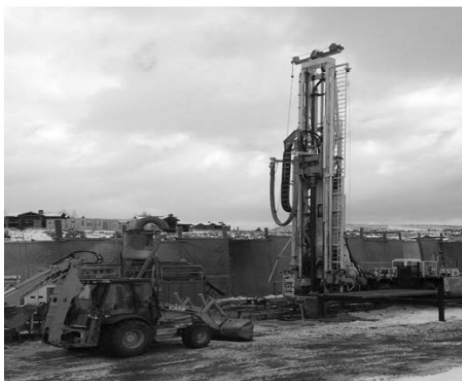
A Boart Longyear™ LR™ 175 electric/hydraulic rotary drill with a quiet genset operating the electric motor and a self-contained electric mud system was utilized in place of the typical diesel/hydraulic rotary drill.
