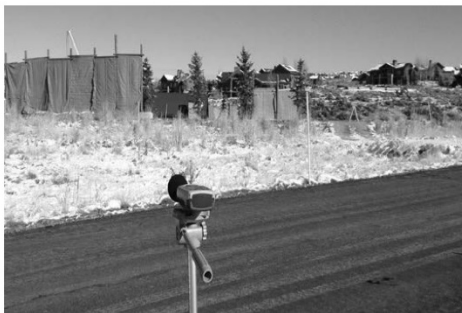
Sound attenuation curtains were constructed on three sides of the project site and mufflers were installed on the drilling rig to further reduce noise output.
