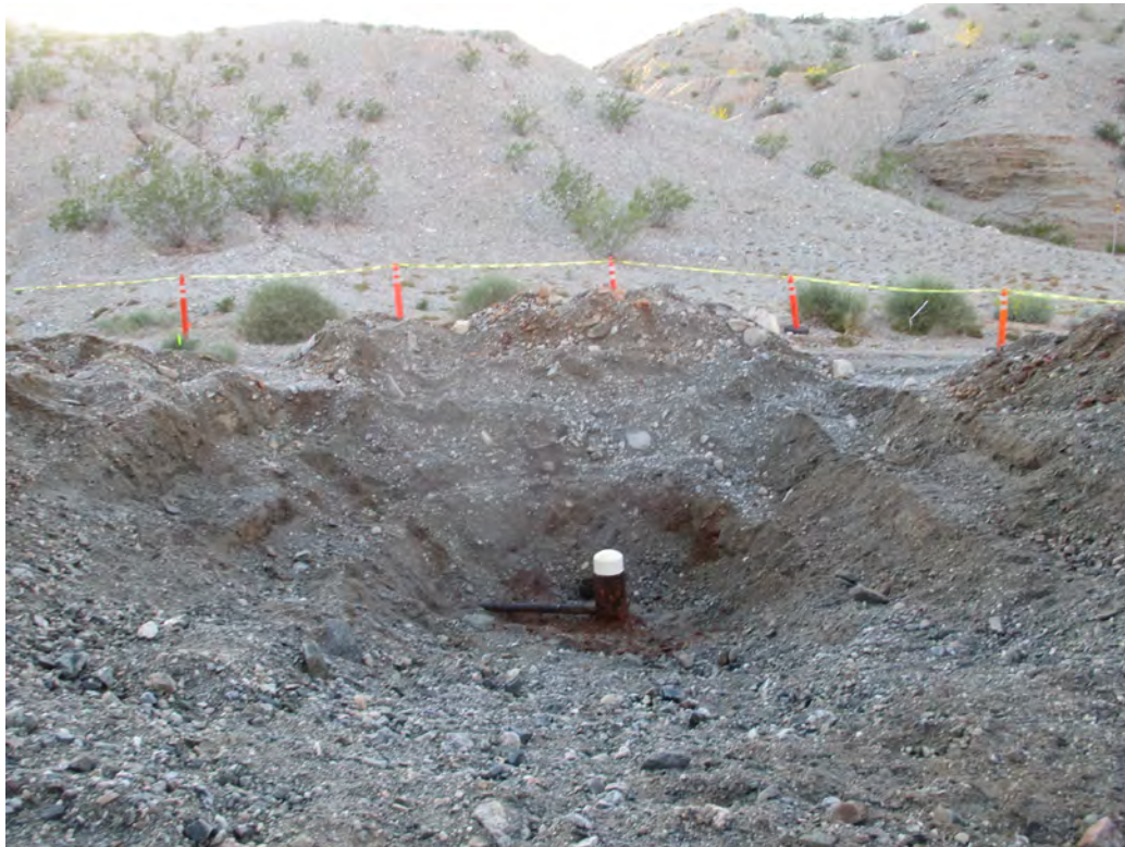
Photo 3A – TCS-4 well head exposed and PVC extension removed. Note intact injection pipe.
