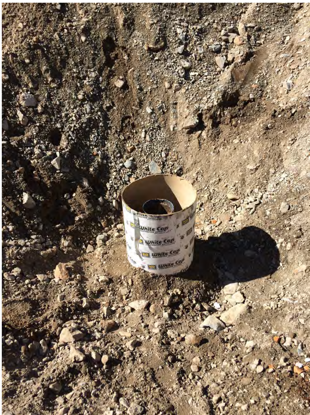
Photo 4 – Placement of 24-inch diameter form over TCS-4 well head for mushroom cap placement.
