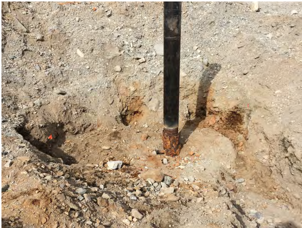
Photo 3B – TCS-4 well head with welded steel casing extension. Note removed section of injection pipe.
