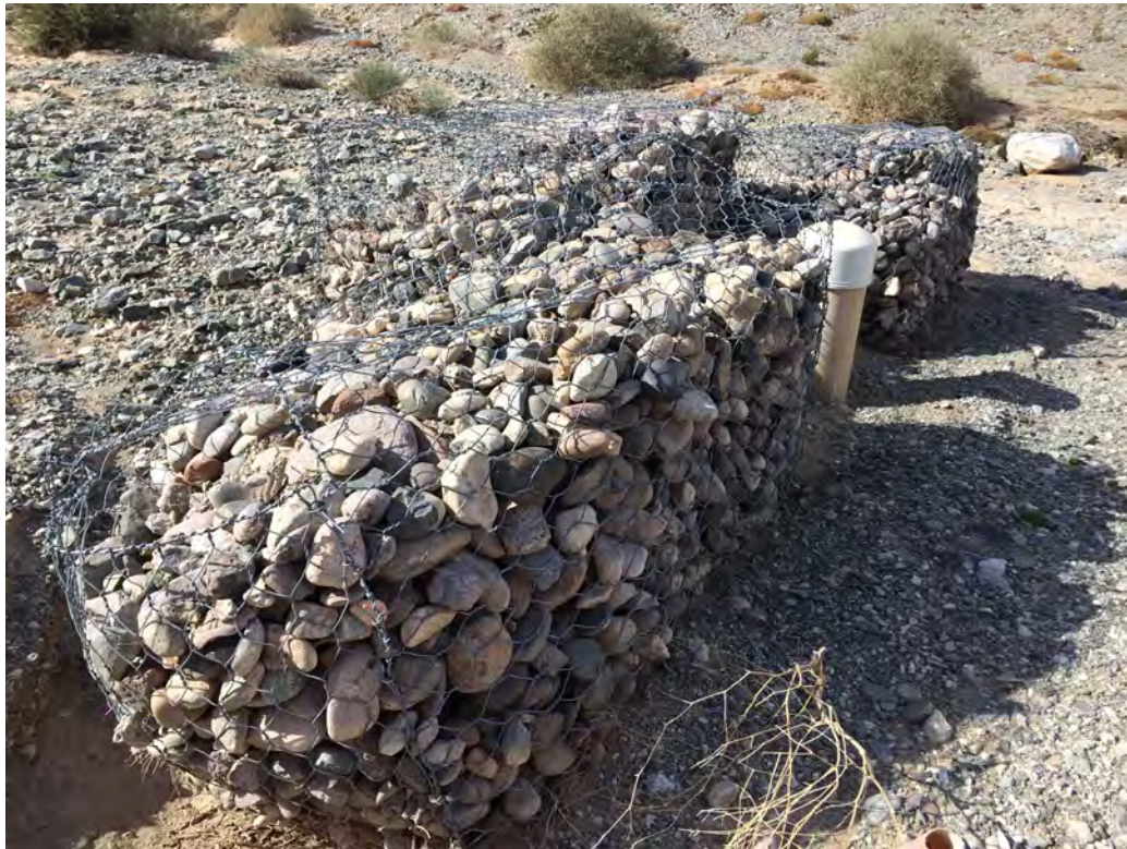
Photo 1 – Well TCS-4 with PVC extension and protective rock gabions prior to work.
