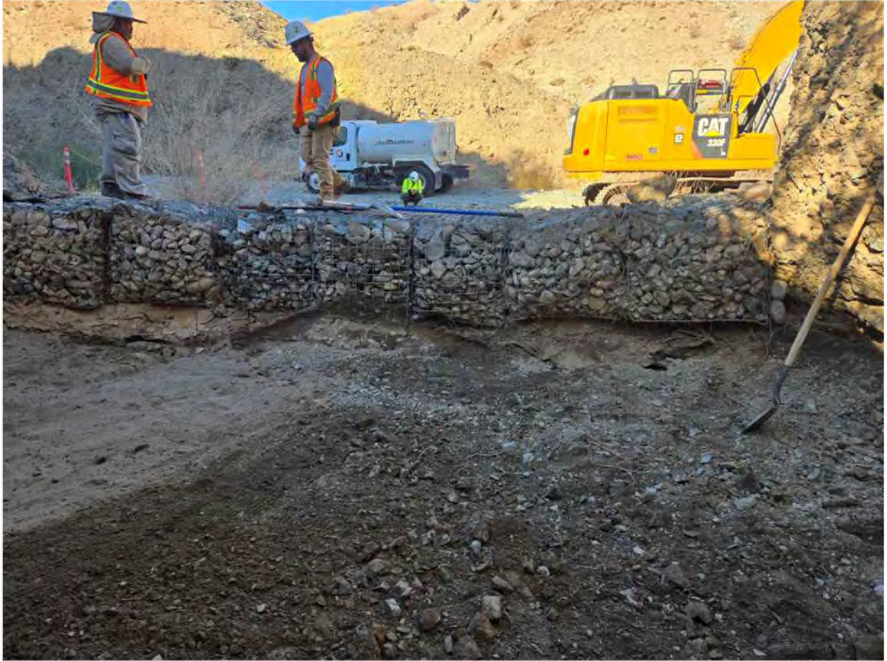
AOC 4 Gabion: Removal Area, November 15, 2024
