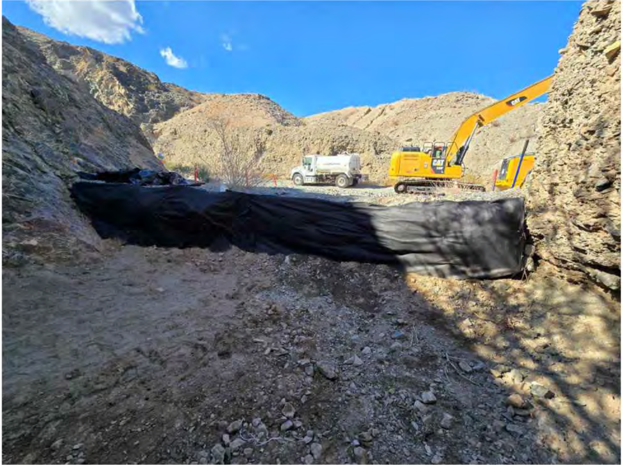
AOC 4 Gabion: Gabion Protected with Geotextile, November 15, 2024
