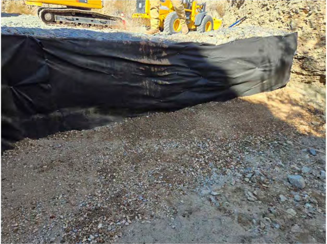
AOC 4 Gabion: Gabion Protected with Geotextile, November 15, 2024
