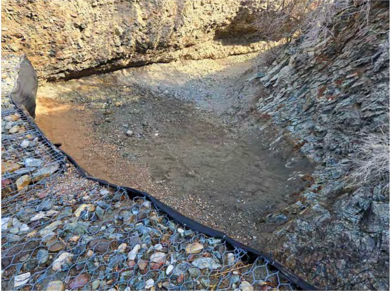
AOC 4 Gabion: Removal Area, November 15, 2024
