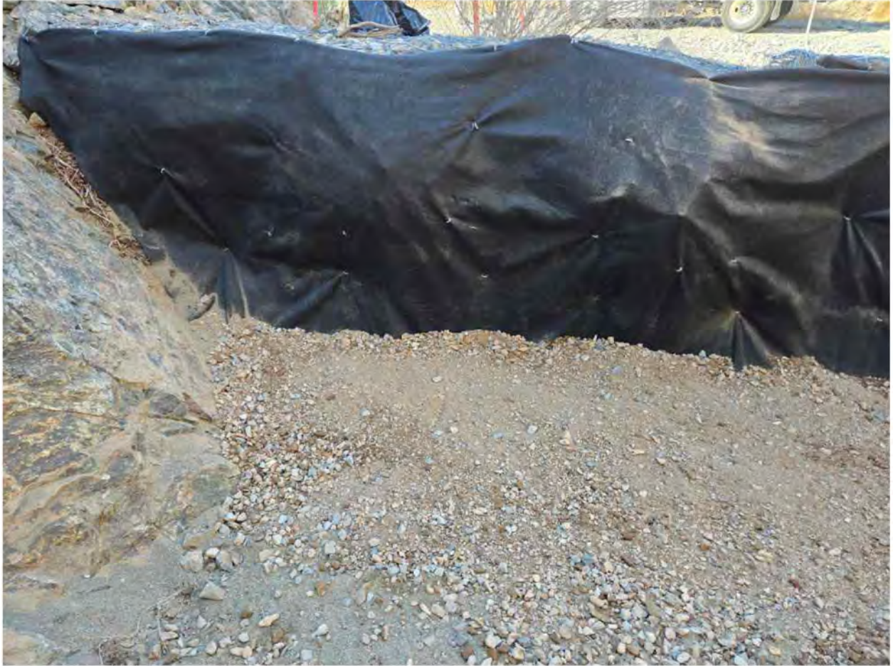
AOC 4 Gabion: Gabion Protected with Geotextile, November 15, 2024
