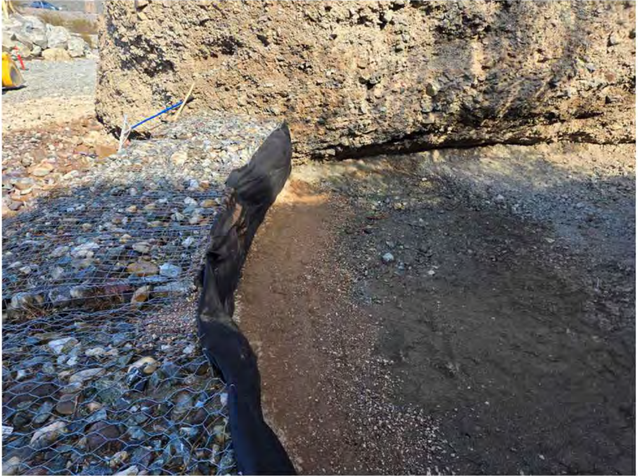
AOC 4 Gabion: Removal Area, November 15, 2024
