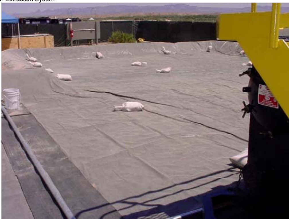
PHOTO 2 Secondary containment expansion
