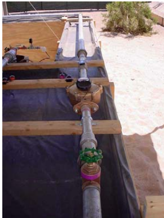
PHOTO 4 Piping, Flow Meters, and Valves from TW-2S within the secondary containment trough.
