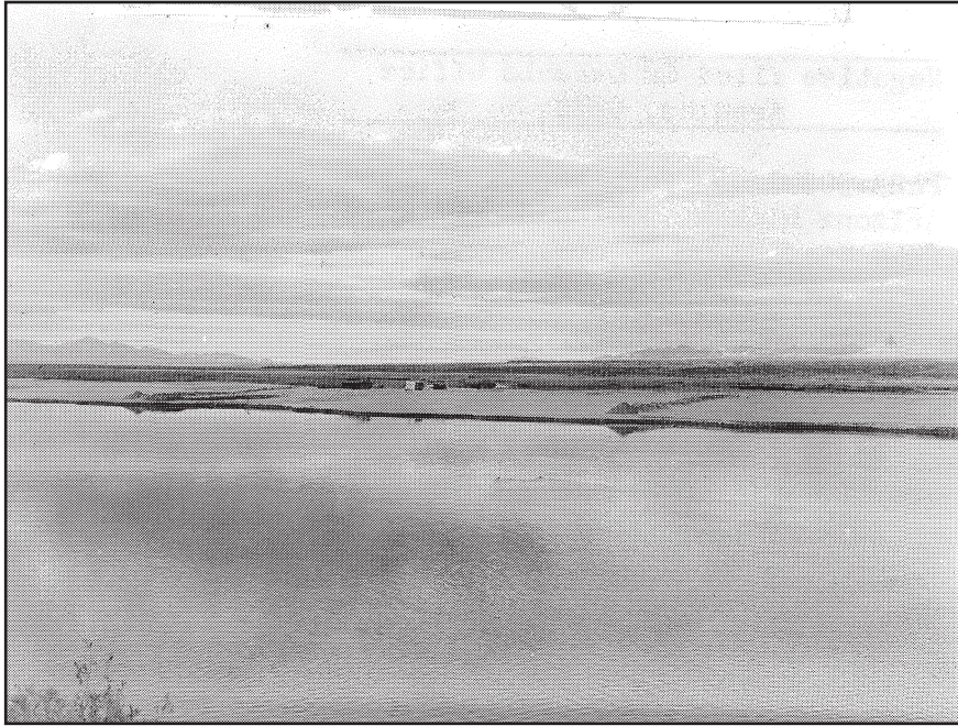
P423-306-1299A. Jetties constructed on Arizona bank at 300' and 500' intervals from Sta. 38-00 to Sta. 67-00. Jan. 31, 1956. Photo by H.B. Burress.
