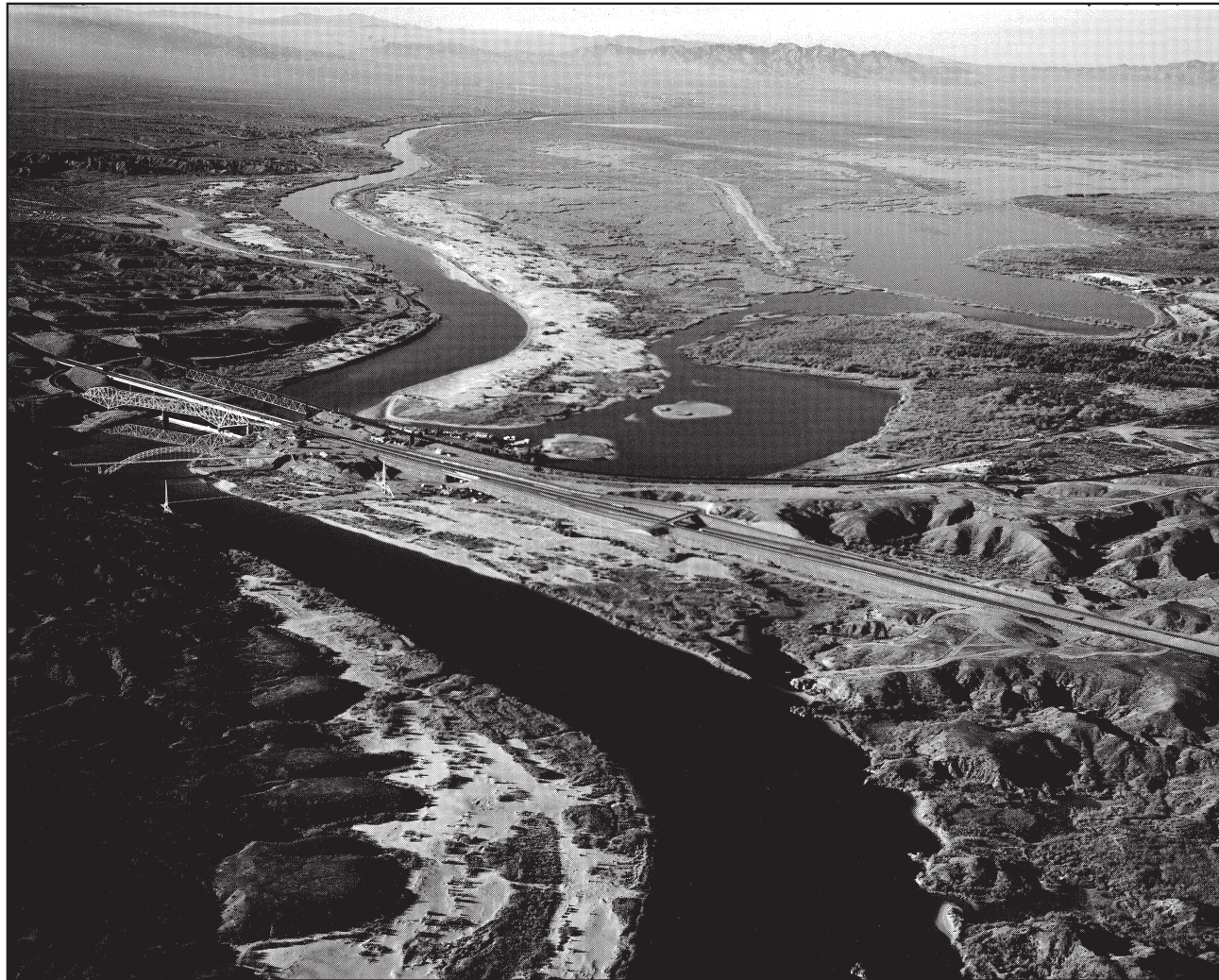
P423-300-8737 NA Topock Gorge Division – Colorado River Front Work & Levee System, Arizona-California. Looking upstream at the start of the Topock Gorge Division area. Portions of this section have been dredged prior to the time that Secretary of the Interior, Stewart Udall, suspended all work in the Topock Gorge Division pending a reevaluation of the dredging program. River Mile 465 is at the bottom of the photograph. 1/6/69 Bureau of Reclamation photo by E. E. Hertzog.
