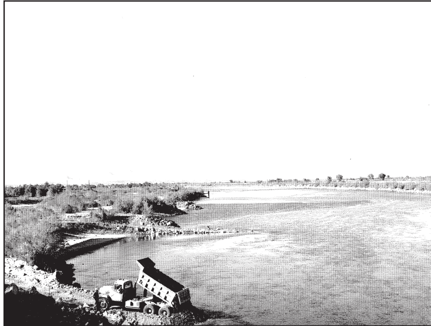
P423-306-4340 NA. Colorado River Front Work and Levee System, Region 3. Needles to Topock Division. Government forces constructing jetty to narrow the width of channel. The channel was narrowed to cause the water to scour sand bar at entrance to Topock Marsh inlet channel structure. Truck at Station 558, California bank. 12/1/65. Bureau of Reclamation photo by Fred Burley.
