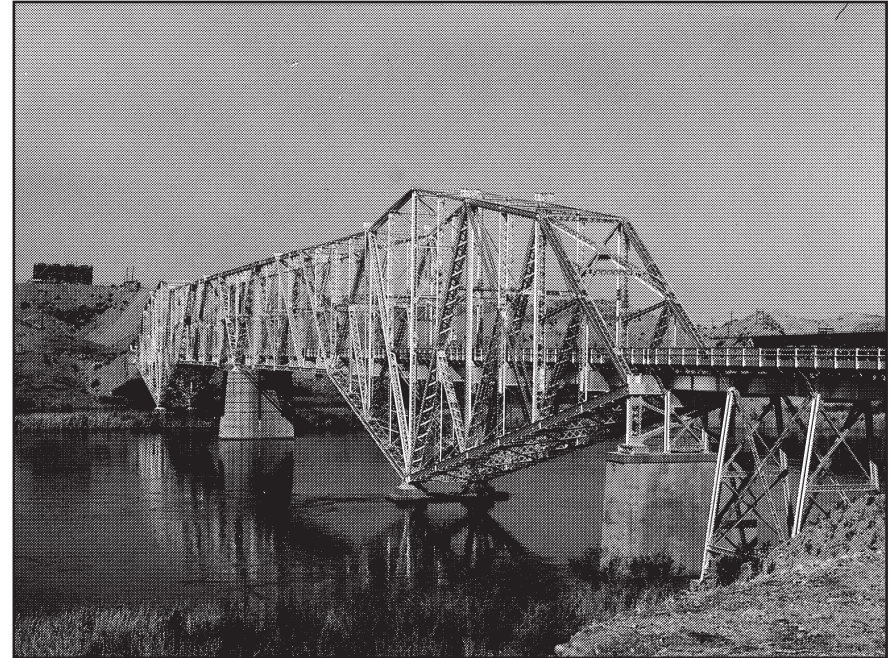
300-4385A. Colorado River Front Work & Levee System. Photograph of highway bridge across Colorado River near Topock, California, 1962. Bureau photo by R.C. Middleton.
