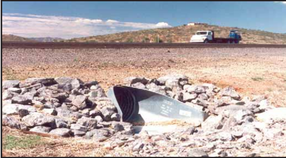
Figure 2.9 Rock rip rap at culvert
