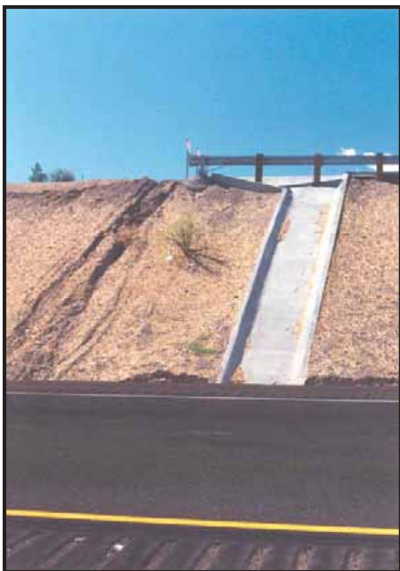
Figure 2.7 (left) Spillway (with failed temporary embankment curb)
