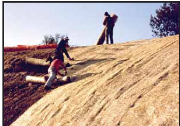
Figure 2.2 Installation of erosion control blanket
