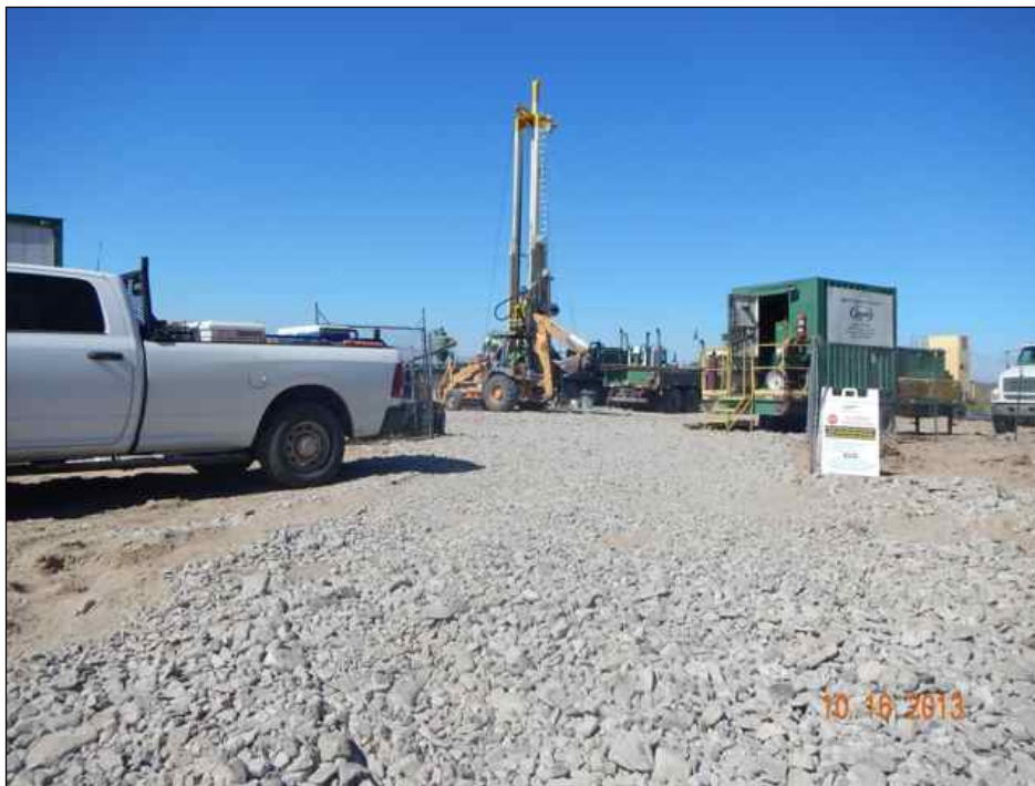
Photo 3. HNWR-1A Site: Drilling activity.
