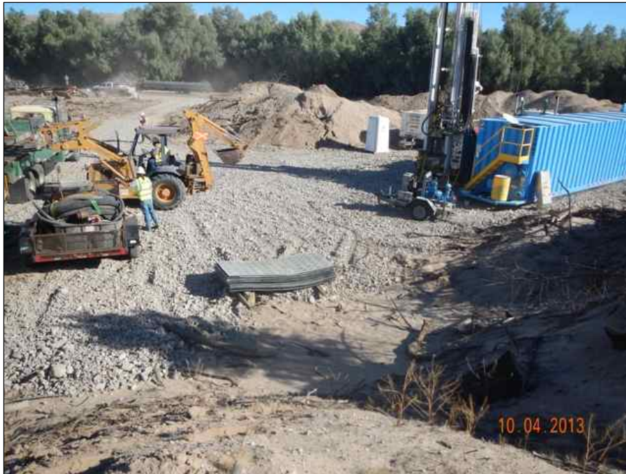
Photo 9. Site B: Drilling activity.
