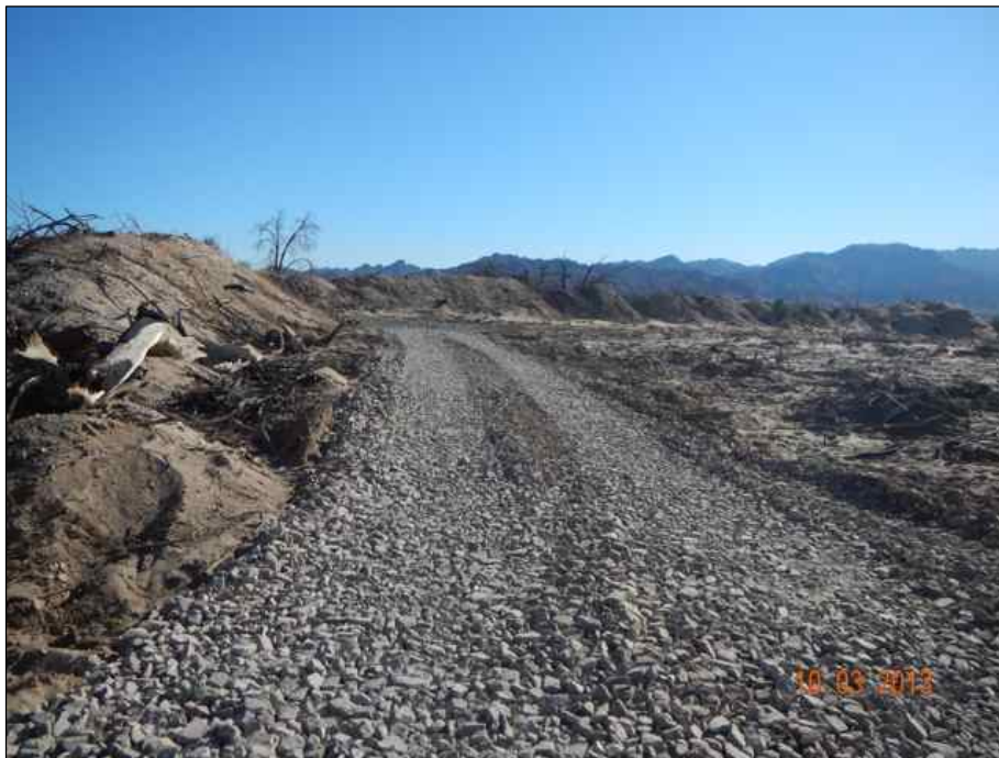
Photo 10. Site B: Gravel placed over soft soil for access.
