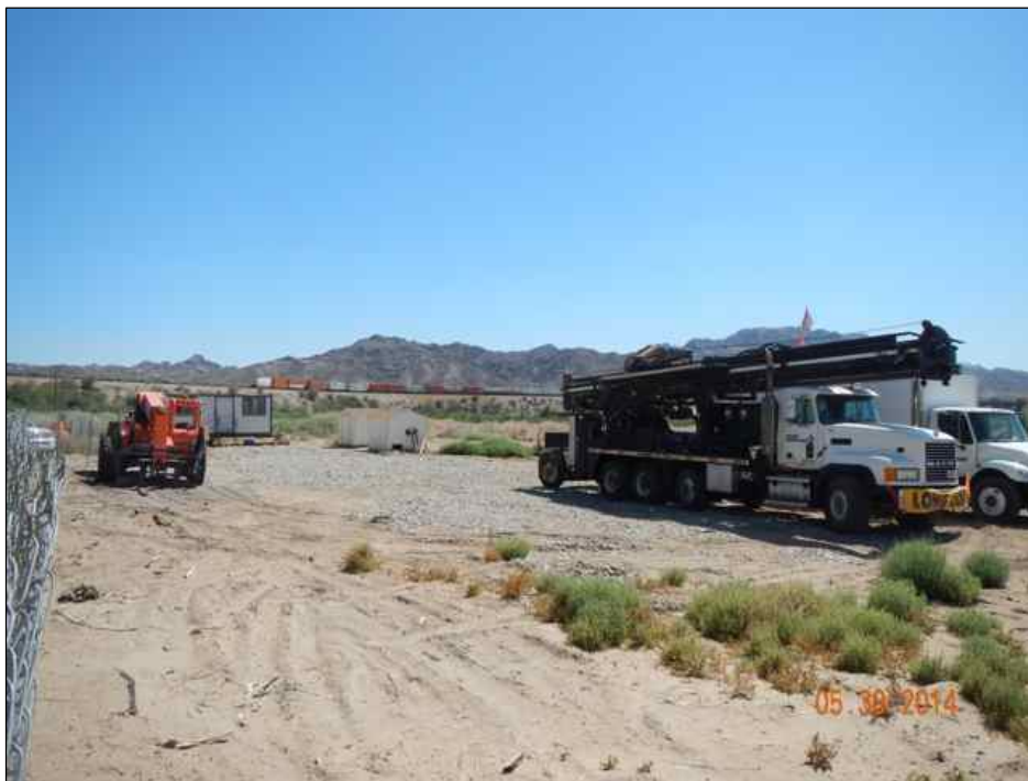
Photo 4. HNWR-1A Site: Equipment on site
