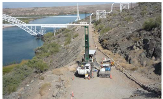
Well drilling in the East Ravine Area
