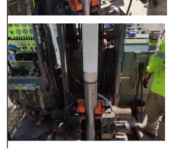
4/20/2022 – ER-01: Installing 20 slot 316L Stainless Screen and Schedule 80 PVC well casing
