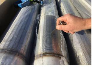
4/20/2022 - ER-01: 6" diameter Schedule 80 PVC casing, and 6-inch diameter 20 slot 316L Stainless Steel Wire Wrapped Screen
