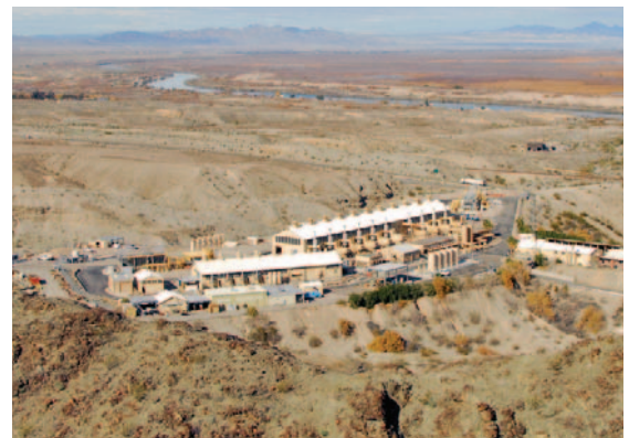
Topock Compressor Station
