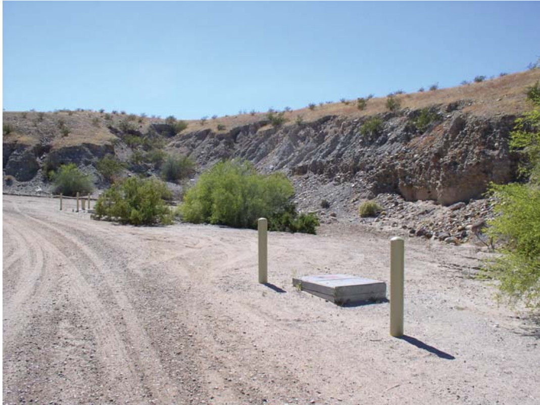
Typical injection well vault with bollards
