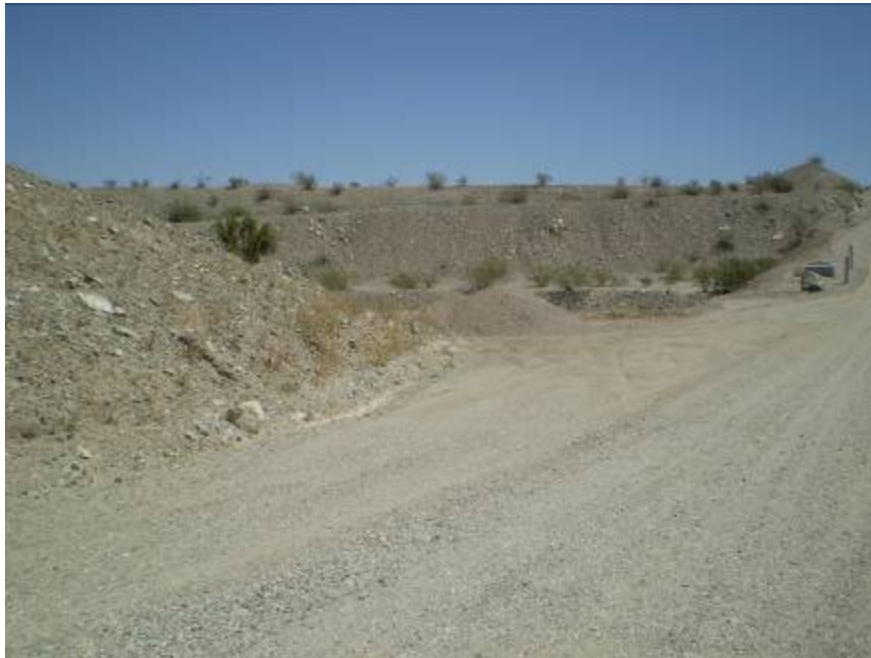
Soil stockpile north of MW-25 - view to east
