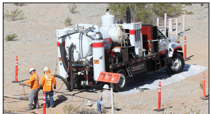
Workers utilize a hydro-vac to conduct soil investigation activities.
