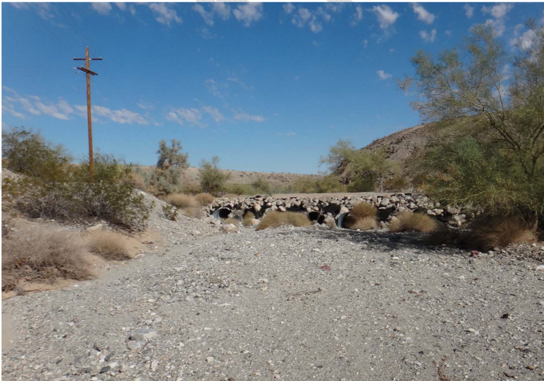
View looking downstream of existing crossing CMPs. From PG&E.
