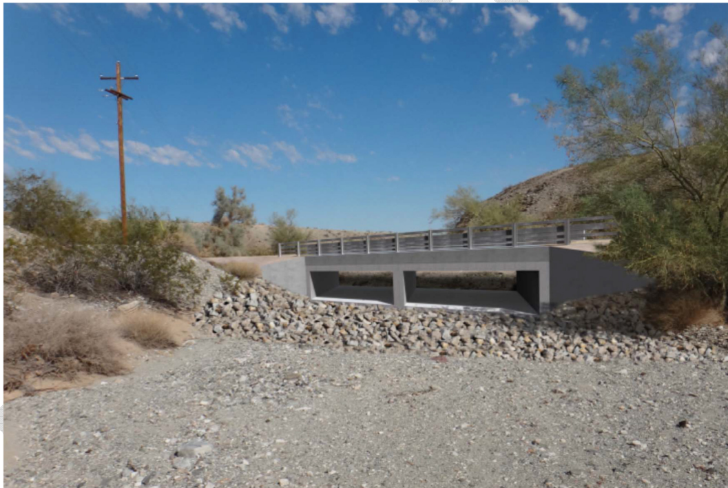
Visual simulation of a proposed box culvert / bridge replacement for crossing on Bat Cave Wash. Image from PG&E.
