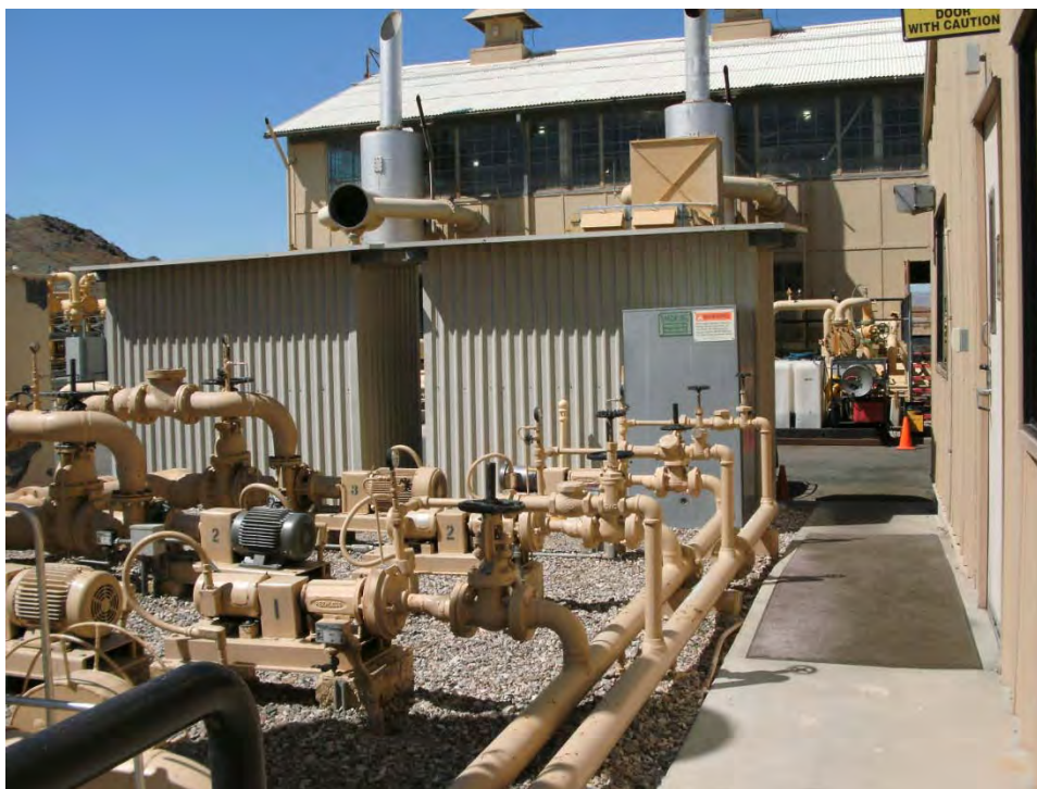
Photograph 23: AOC 15 Auxiliary Jacket Cooling Water Pumps, looking west
