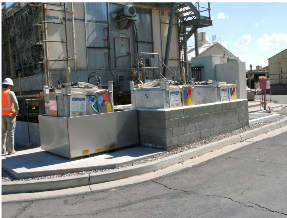
Photograph 4: AOC 5 Cooling Tower A, south side, showing sulfuric acid tanks
