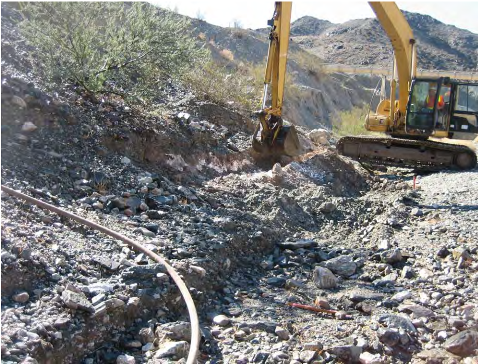
Photograph 22: Horizontal lens of white powder in small observation trench located between trenching locations SWMU1-WP-6a and SWMU1-WP-7
