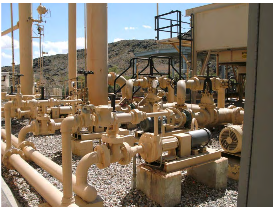
Photograph 24: AOC 15 Auxiliary Jacket Cooling Water Pumps, looking southeast
