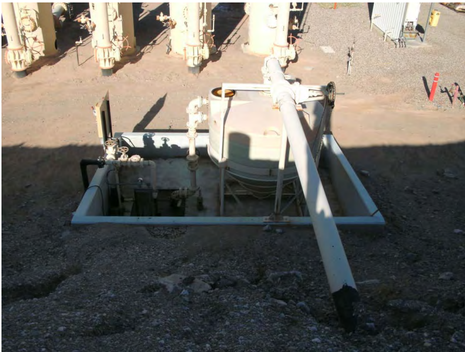
Photograph 50: AOC 24 Grit Tank, looking down from upper yard; likely location of AOC 24 potential American Petroleum Institute (API) separator
