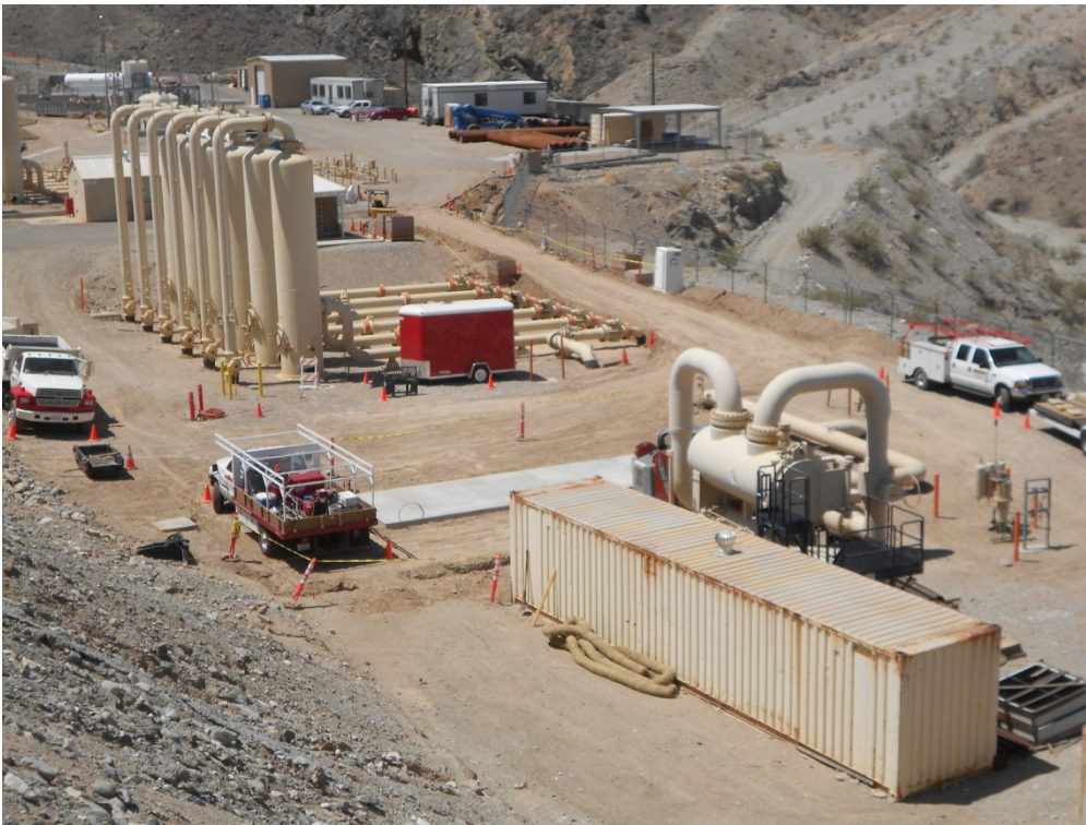
Photograph 50: View of AOC 24, Stained Area and Former API Oil/Water Separator, looking southwest from upper yard
