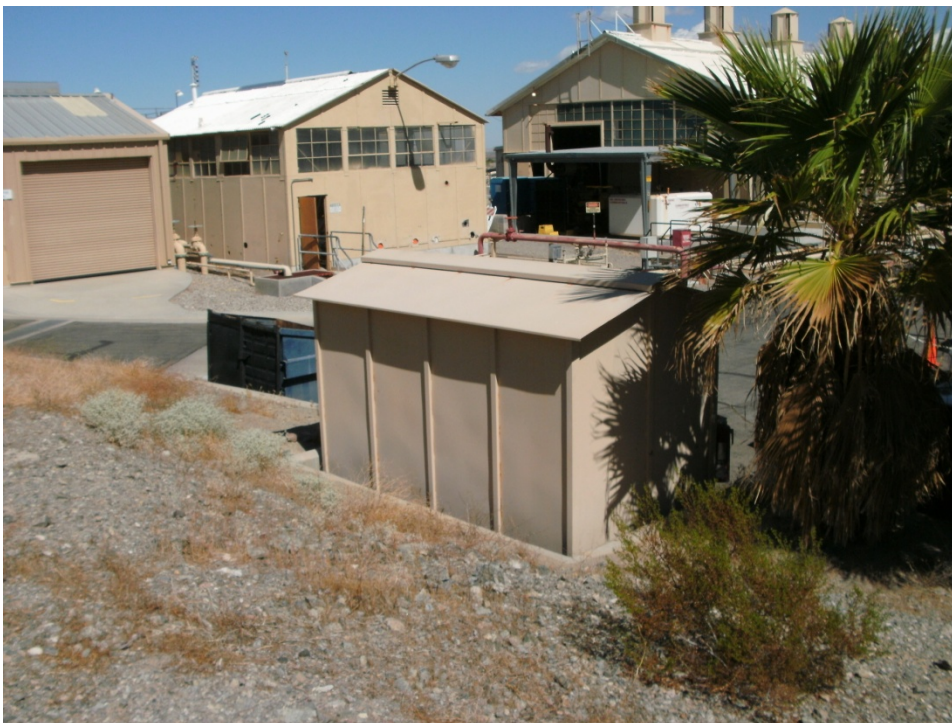
Photograph 14: AOC 8 Paint Locker, south side, looking northwest toward AOC 23, Former Water Conditioning Building
