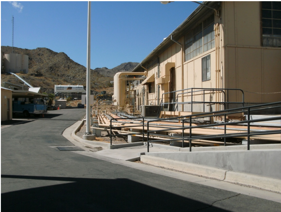
Photograph 54: AOC 25 Compressor and Generator Engine Basements, Auxiliary Building, east side, looking south
