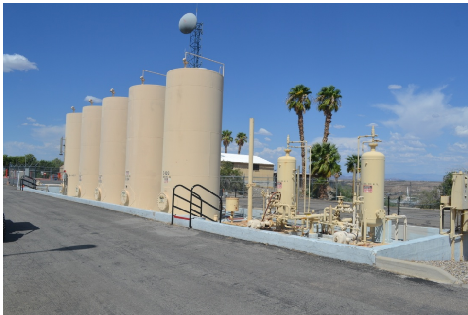
Photograph 64: AOC 32 Oil Storage Tanks and Waste Oil Sump, looking northeast from Control Building
