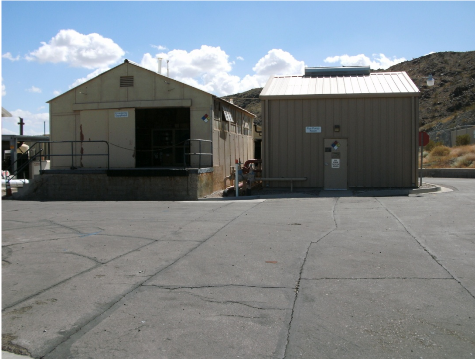
Photograph 47: AOC 23, Former Water Conditioning Building, west side, and Fire Pump Building, looking east
