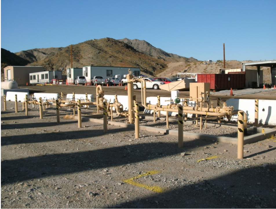
Photograph 61: View toward former Oily Water Treatment System, SWMU 5, SWMU 6, SWMU 9, and AOC 21 area from valve nest west of south scrubbers, looking southwest
