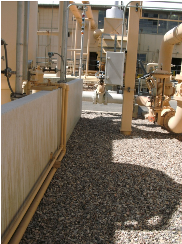
Photograph 28: AOC 19, Former Cooling Liquid Mixing Area and Former Hotwell, showing unpaved area north of former hotwell, by temporary compressor engine oil holding tanks
