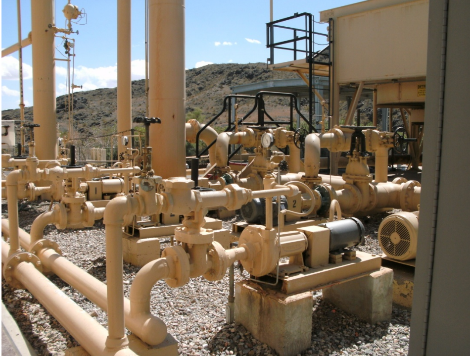
Photograph 25: AOC 15, Auxiliary Jacket Cooling Water Pumps, looking southeast from SCADA cabinets on west side of unit
