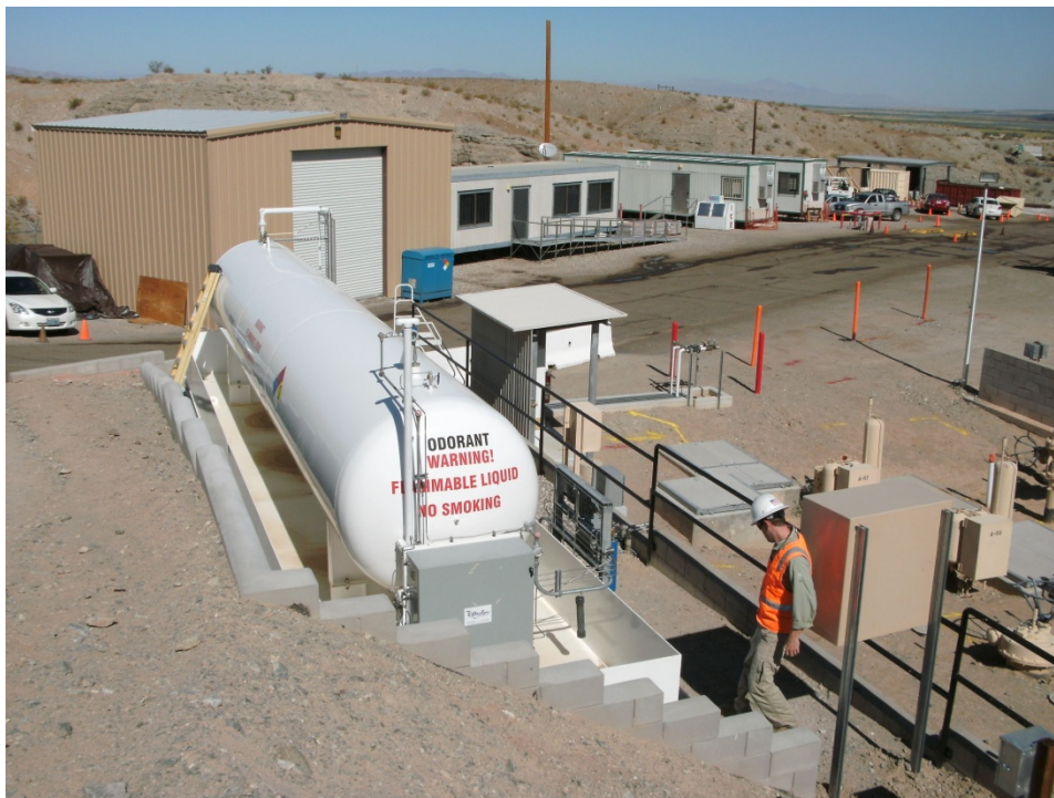
Photograph 60: View of former Oily Water Treatment System, SWMU 5, SWMU 6, SWMU 9, and AOC 21 area from New Odorant Tank, looking northwest
