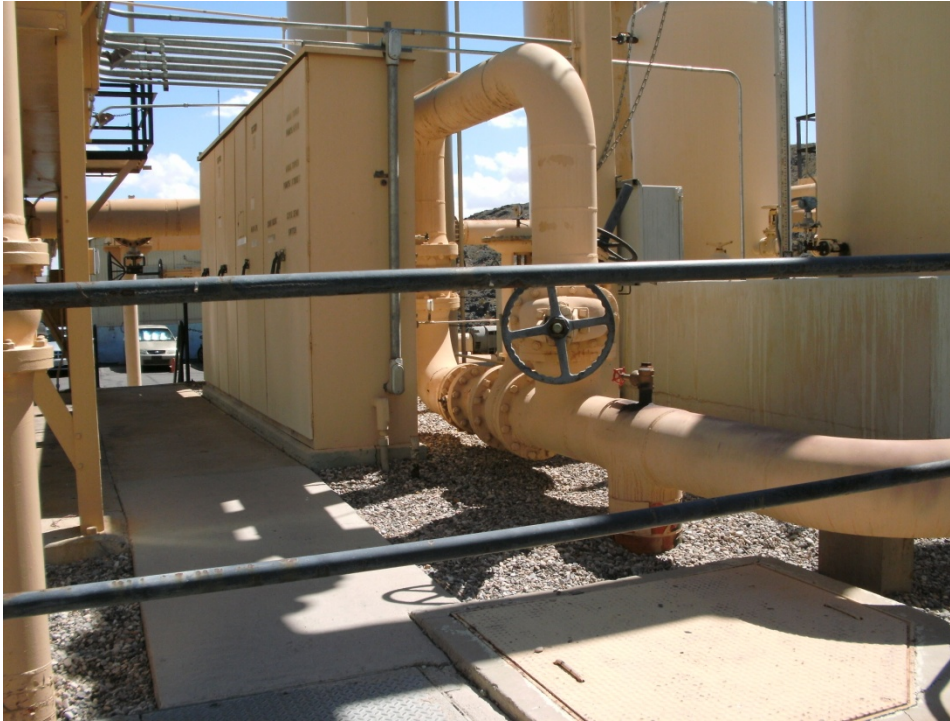
Photograph 29: AOC 19, Former Cooling Liquid Mixing Area and Former Hotwell, northwest corner looking east-southeast
