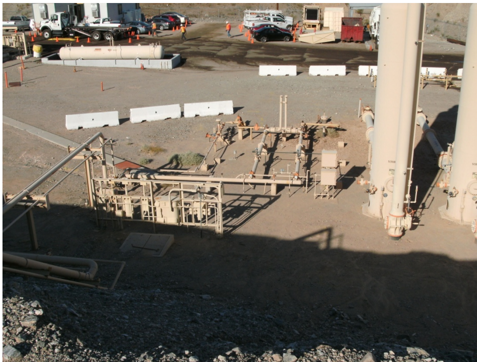
Photograph 59: AOC 26, Former Scrubber Oil Sump, view into area of former sump, showing piping and other access constraints
