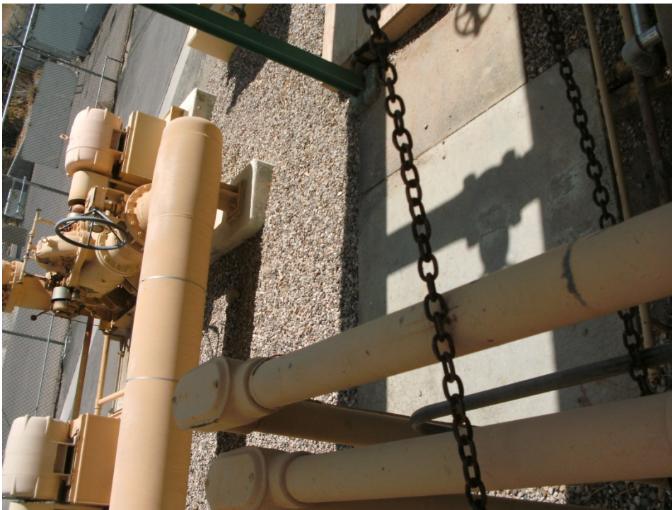
Photograph 30: AOC 19, Former Cooling Liquid Mixing Area and Former Hotwell, Concrete pad area looking down and southeast from former hotwell area
