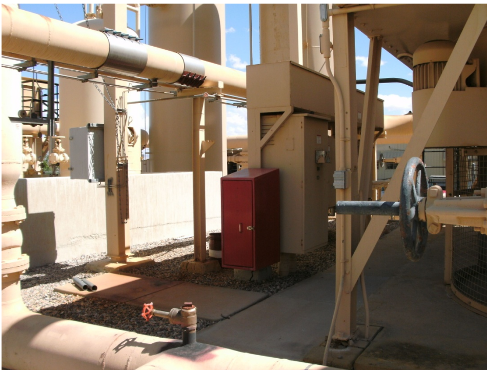
Photograph 38: AOC 19, Former Cooling Liquid Mixing Area and Former Hotwell, south side, looking northeast
