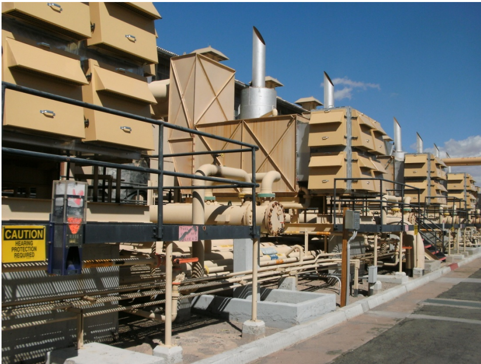
Photograph 52: AOC 25, Compressor and Generator Engine Basements, east side of Compressor Building looking north, showing paved and unpaved areas under piping
