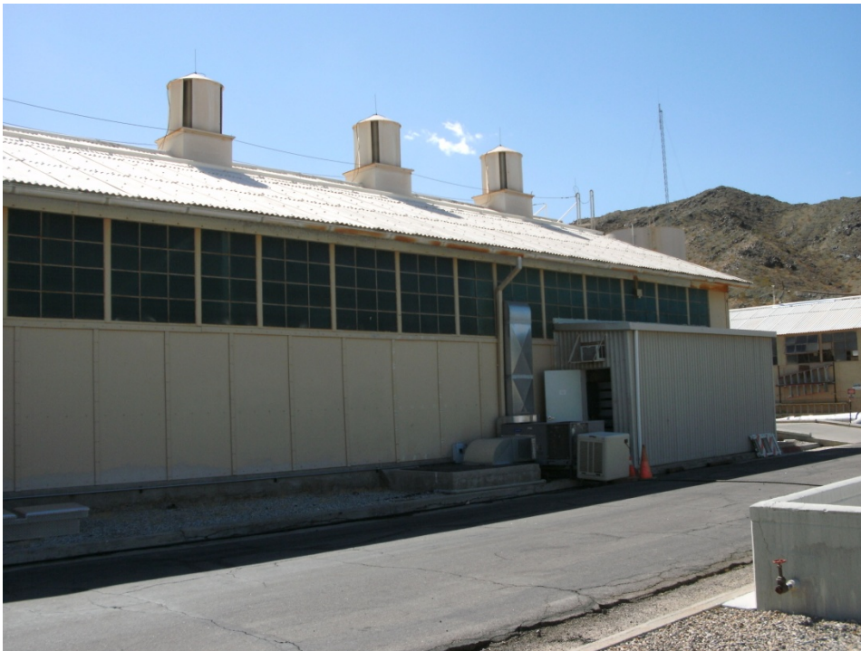
Photograph 56: AOC 25 Compressor and Generator Engine Basements, Auxiliary Building, west side, southern half, looking south-southeast
