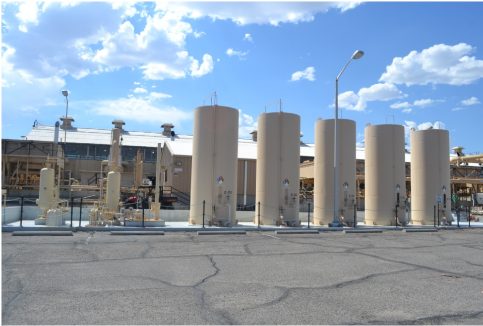
Photograph 65: AOC 32 Oil Storage Tanks and Waste Oil Sump, looking west from Visitor Parking Lot
