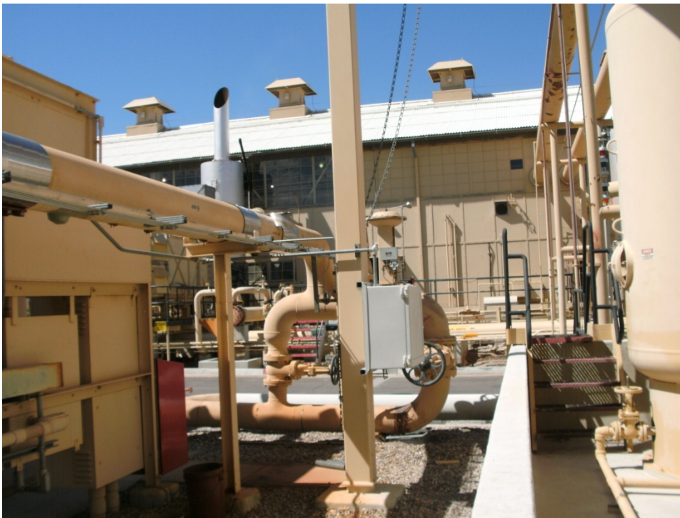
Photograph 42: AOC 19, Former Cooling Liquid Mixing Area and Former Hotwell, south side, looking west
