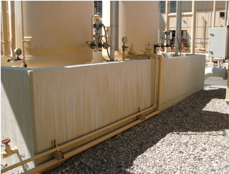
Photograph 37: AOC 19, Former Cooling Liquid Mixing Area and Former Hotwell, north side, looking west-southwest
