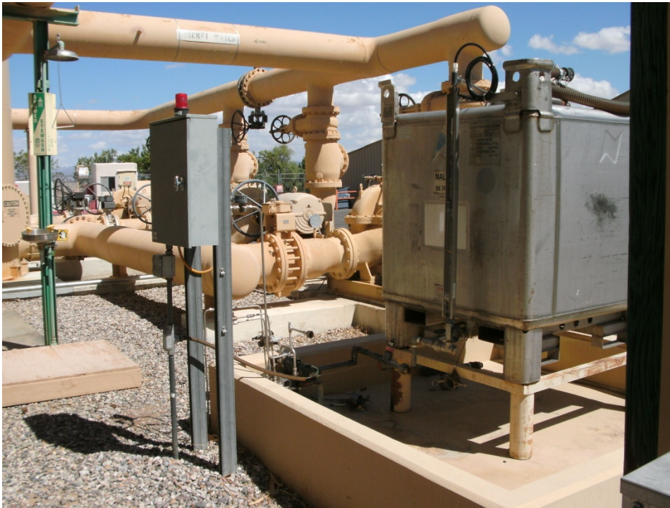
Photograph 35: AOC 19, Former Cooling Liquid Mixing Area and Former Hotwell, east side, looking north, showing utilities and access
