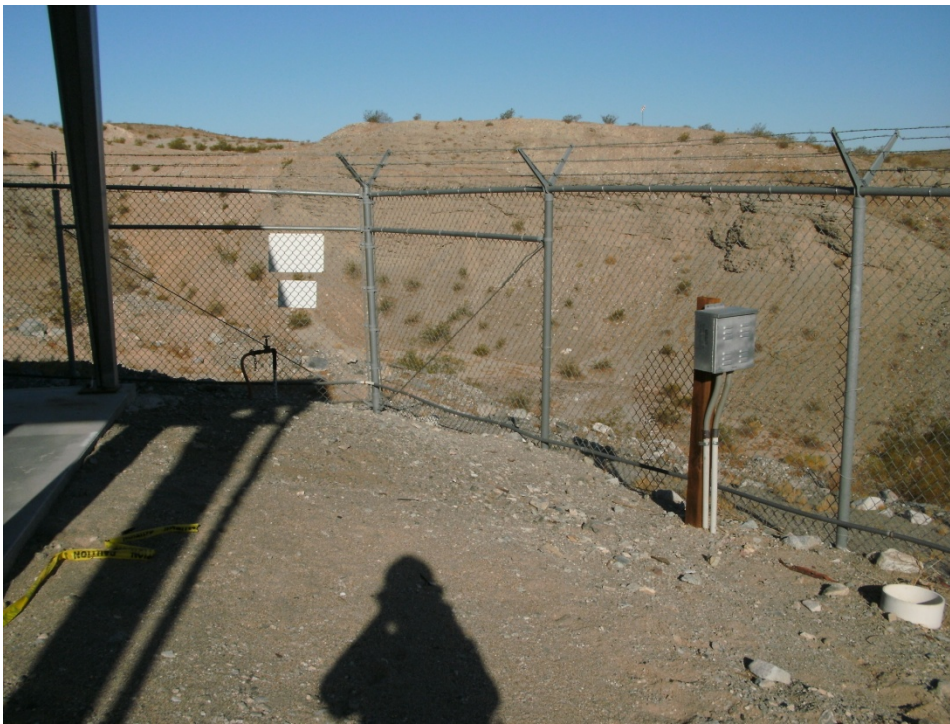
Photograph 26: AOC 16, Sandblast Shelter, Utilities along fence line north of unit
