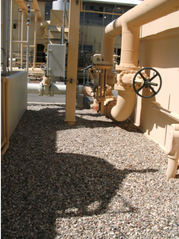
Photograph 31: AOC 19, Former Cooling Liquid Mixing Area and Former Hotwell, unpaved area north of former hotwell, second view
