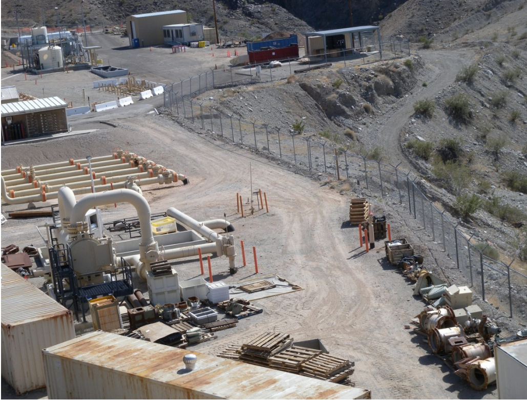
Photograph 63: Overview of lower yard, showing western portion of lower yard, looking southwest from upper yard
