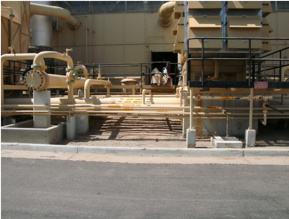
Photograph 15: AOC 13, Unpaved Areas at the Compressor Station, example of unpaved area on east side of Compressor Building
