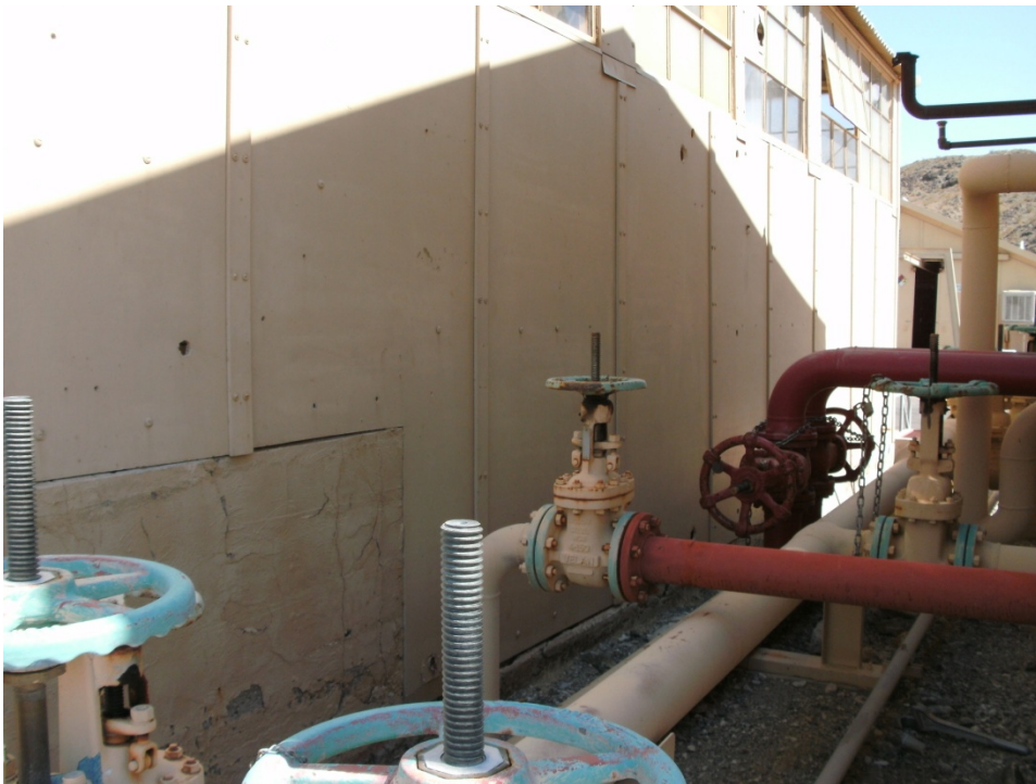
Photograph 48: AOC 23, Former Water Conditioning Building, Close-up of Foundation of Water Conditioning Building and adjacent utilities, looking northeast
