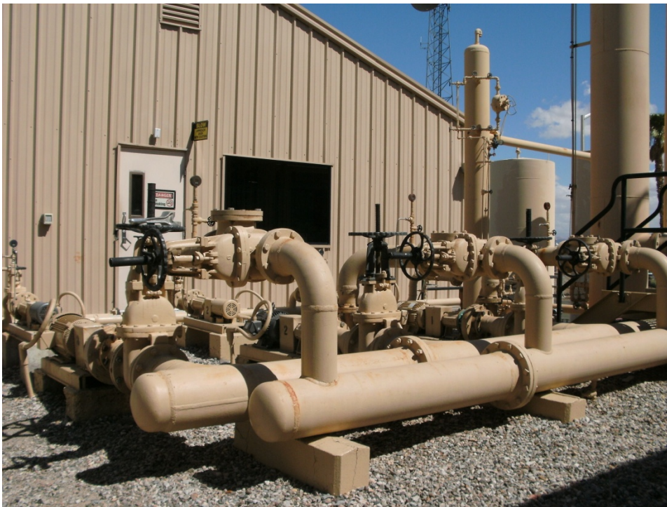
Photograph 20: AOC 15 Auxiliary Jacket Cooling Water Pumps, looking north, Control Building in Background
