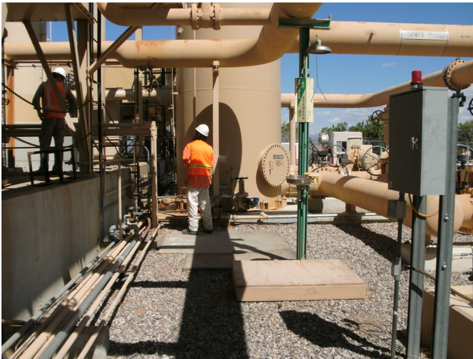
Photograph 34: AOC 19, Former Cooling Liquid Mixing Area and Former Hotwell, east side, looking north, showing utilities, raised foundation in former hotwell area and access
