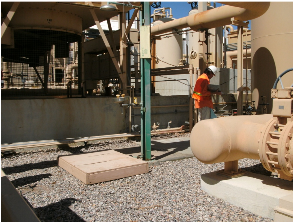
Photograph 36: AOC 19, Former Cooling Liquid Mixing Area and Former Hotwell, east side, looking northwest, showing utilities, raised foundation in former hotwell area, and access
