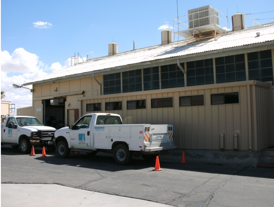
Photograph 55: AOC 25, Compressor and Generator Engine Basements, Auxiliary Building, west side, northern portion, looking northeast
