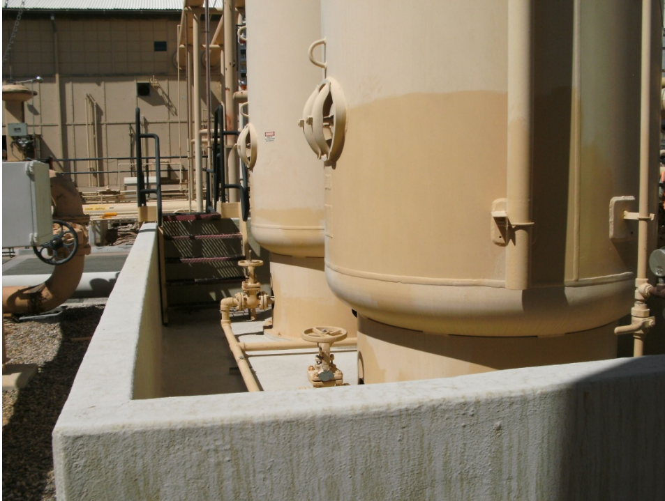
Photograph 39: AOC 19, Former Cooling Liquid Mixing Area and Former Hotwell, south side, looking west, showing part of inside of containment for temporary compressor engine oil holding tanks
