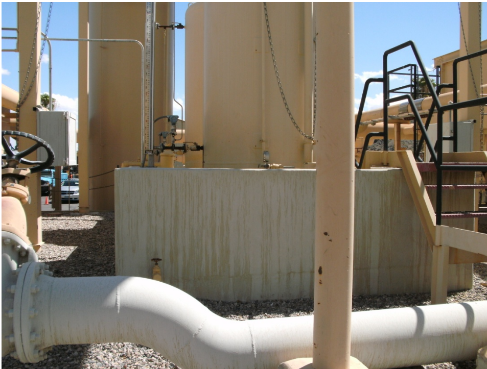
Photograph 32: AOC 19, Former Cooling Liquid Mixing Area and Former Hotwell, west side, looking east
