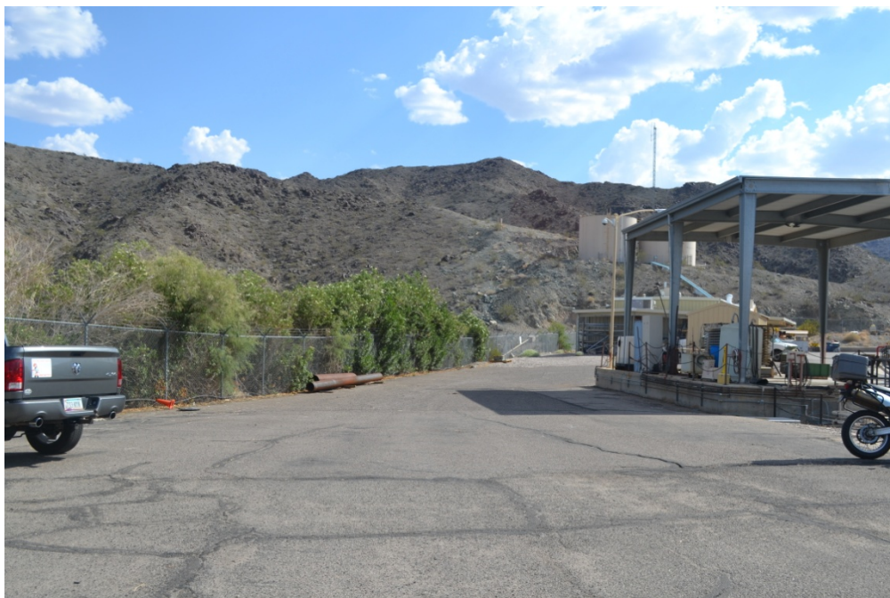
Photograph 67: AOC 33, Potential Former Burn Area, looking south from north portion of Visitor Parking lot
