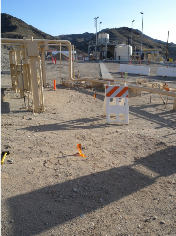
Photograph 57: AOC 26, Former Scrubber Oil Sump, showing area of former excavation
