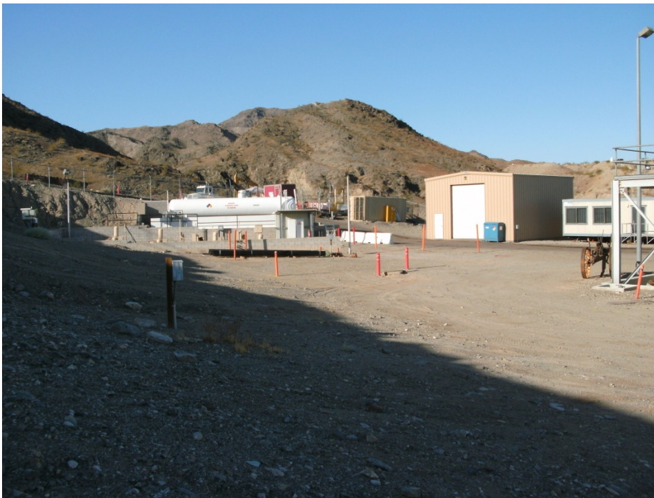
Photograph 16: AOC 13, Unpaved Areas at the Compressor Station, showing miscellaneous utilities, southeast portion of lower yard
