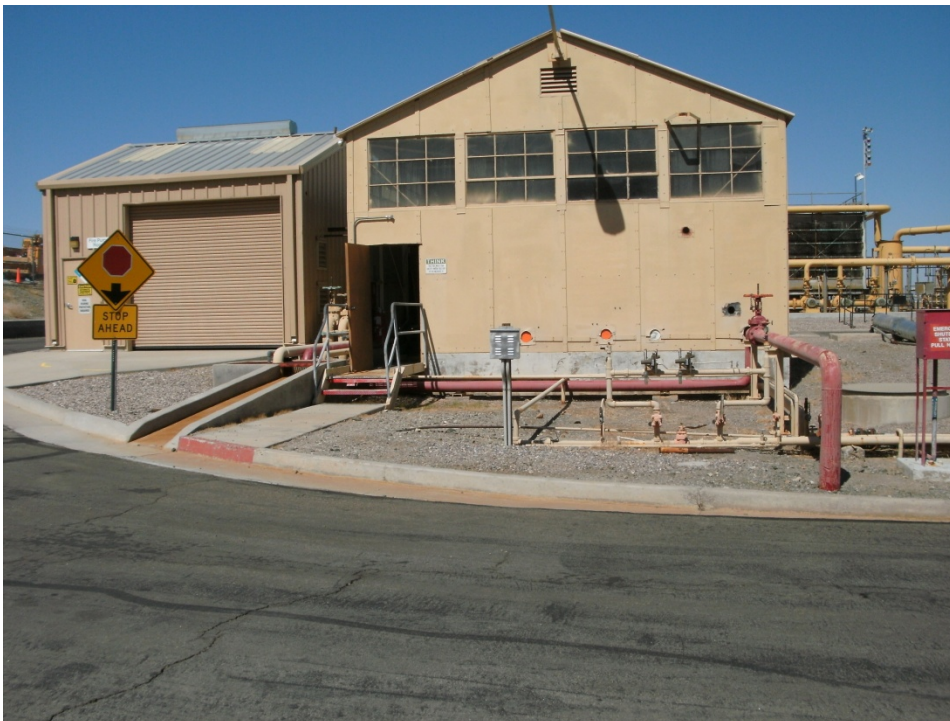
Photograph 46: AOC 23, Former Water Conditioning Building, east side, and Fire Pump Building, looking west
