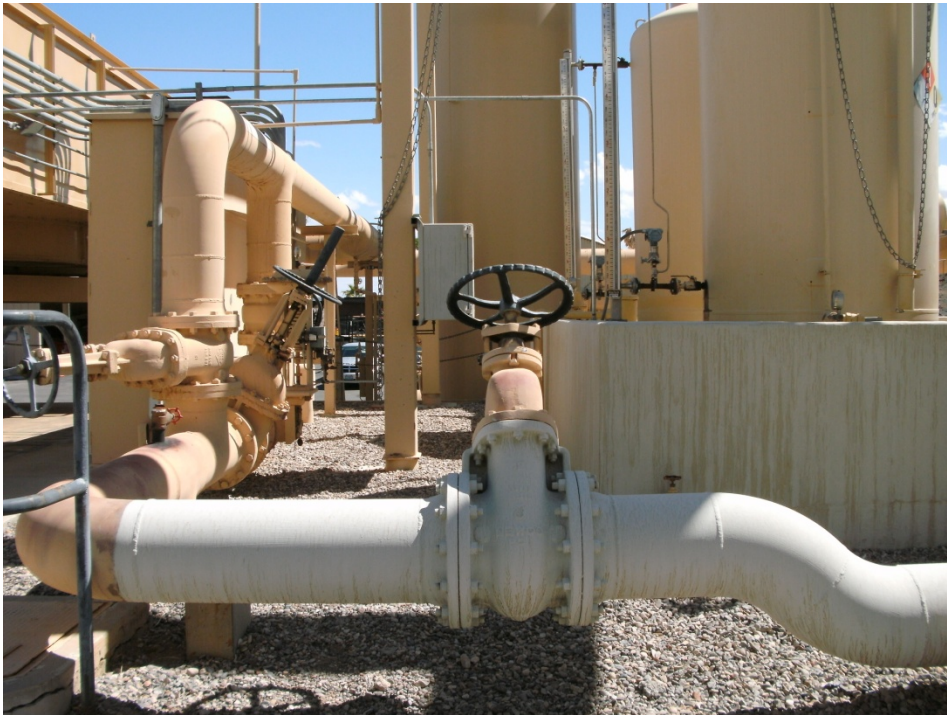
Photograph 41: AOC 19, Former Cooling Liquid Mixing Area and Former Hotwell, west side, looking east, showing access on north side of former hotwell area
