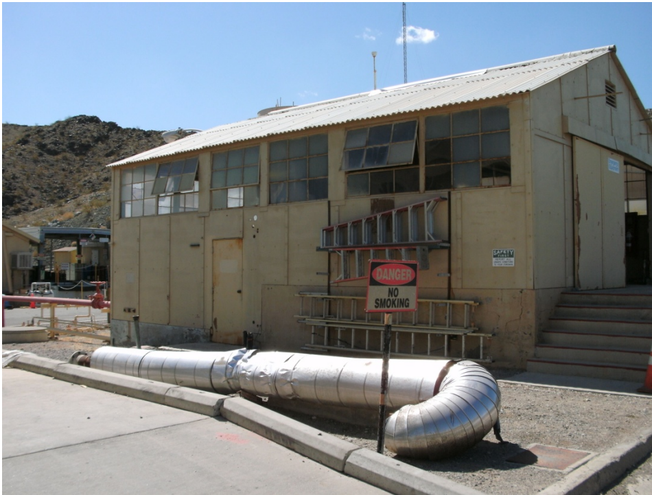
Photograph 45: AOC 23, Former Water Conditioning Building, north side, looking southeast, showing variable foundation heights
