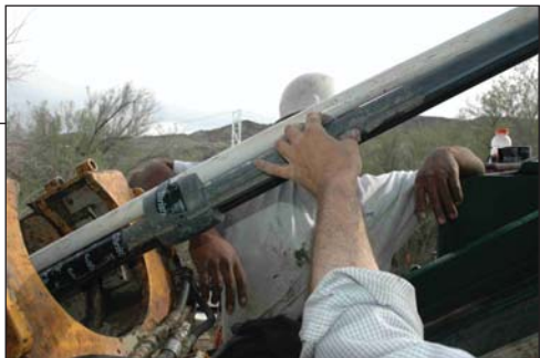
Centralizer with bundled tremie pipe and sounding conduit. Sample tubing recess is being packed with bentonite.
