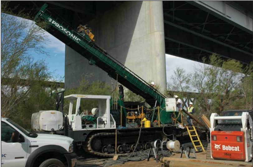
Rotosonic drill rig set up on an angle.
