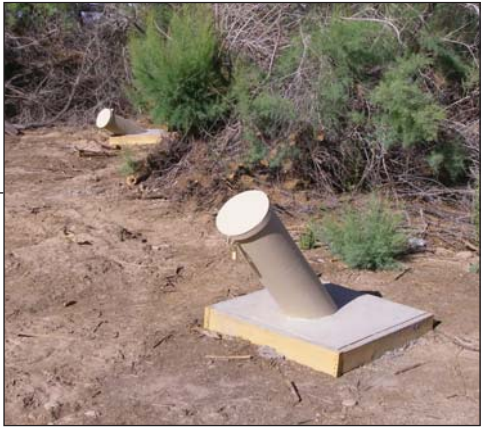
Completed wellheads MW-52 (near) and MW-53 (far).
