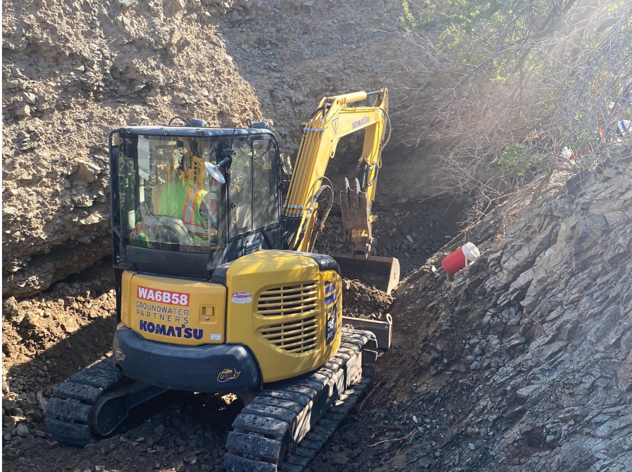
AOC 4 Gabion: Removal of Soil with Mini-Sized Excavator, September 15, 2021
