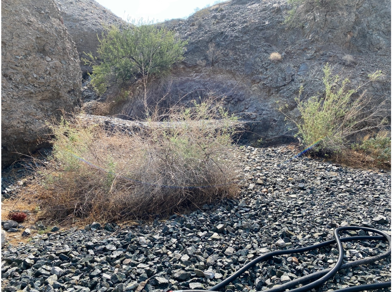
AOC 4 Gabion: Restored Work Area, September 22, 2021
