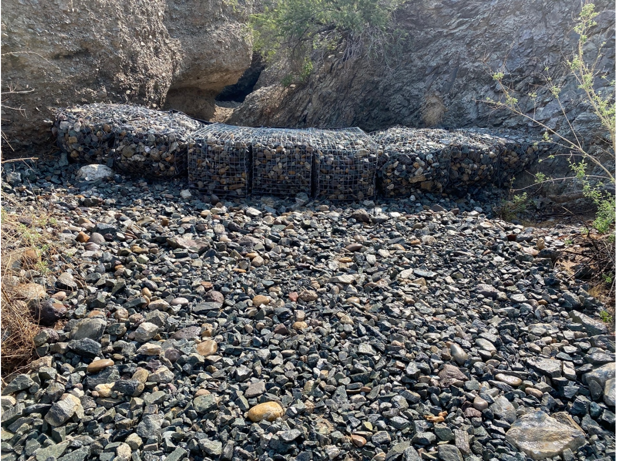
AOC 4 Gabion: Rebuilt Gabion with New Metal Cages, September 22, 2021
