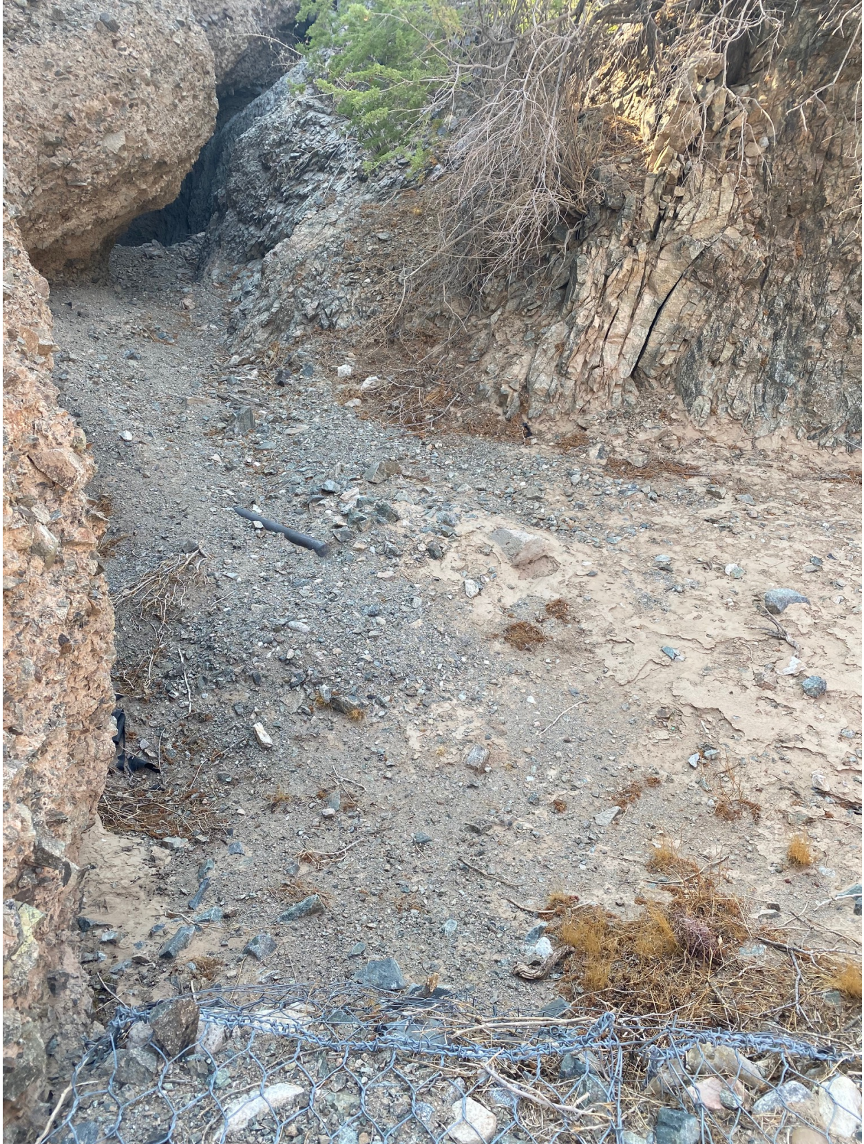
AOC 4 Gabion: June 17, 2021
