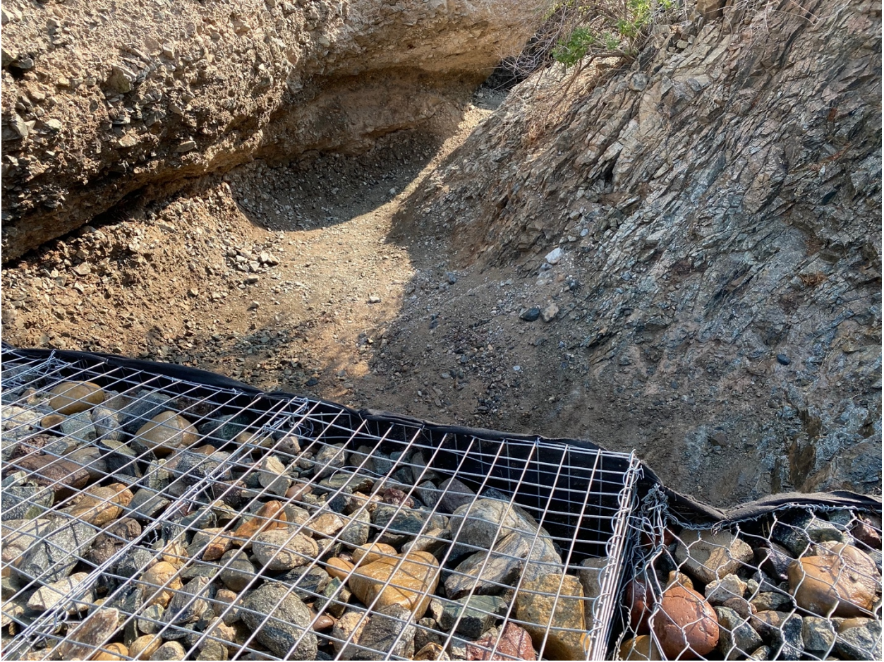
AOC 4 Gabion: Completed Excavation, September 21, 2021
