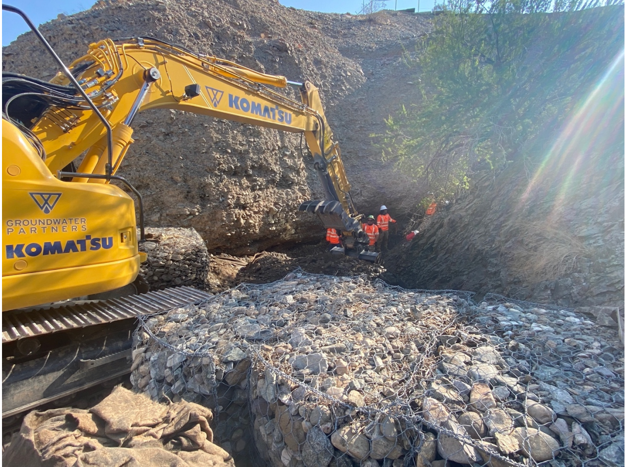
AOC 4 Gabion: Removal of Gabion with Mid-Sized Excavator, September 14, 2021
