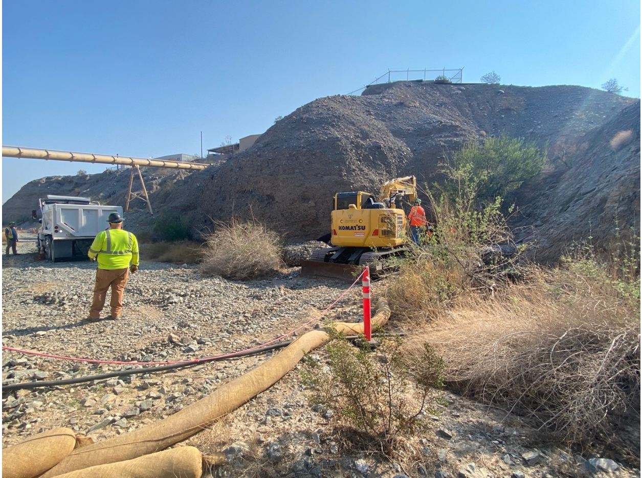
AOC 4 Gabion: Mobilization, September 13, 2021
