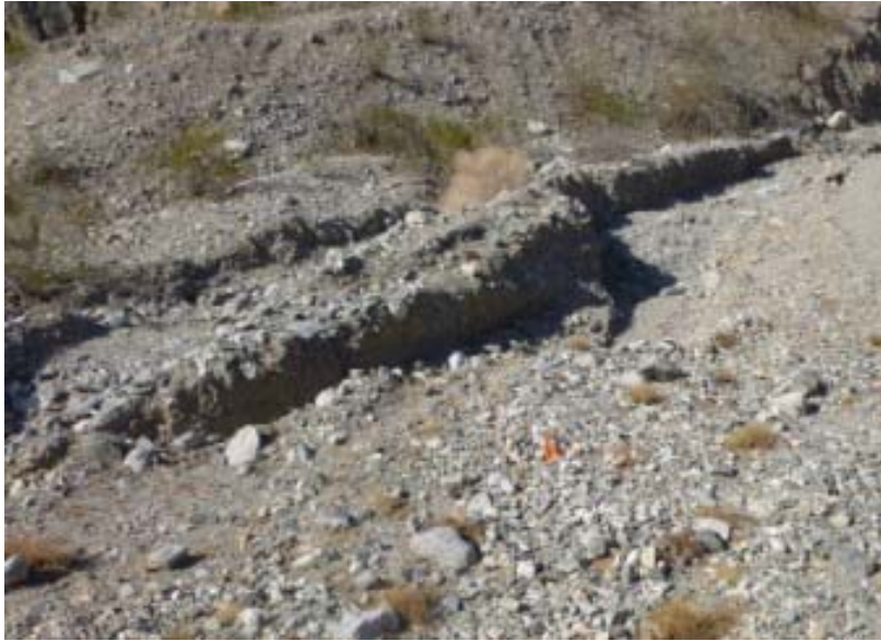
EXHIBIT 3.5-3 SEVERE EROSION OBSERVED ON ROAD, WEST OF FRESHWATER INJECTION WELL FW-2 Groundwater Remedy Basis of Design Report/Pre-Final (90%) Design PG&E Topock Compressor Station, Needles, California
