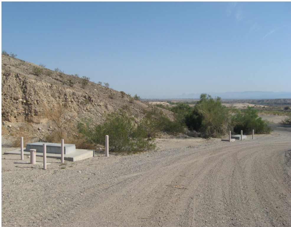
PHOTOGRAPH 10 Valve Vaults along Extraction and Brine Pipelines, Typical
