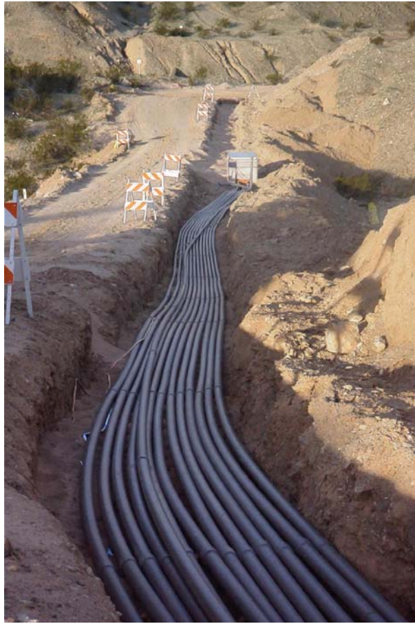
PHOTOGRAPH 9 Underground Extraction and Brine Pipelines and Conduits
