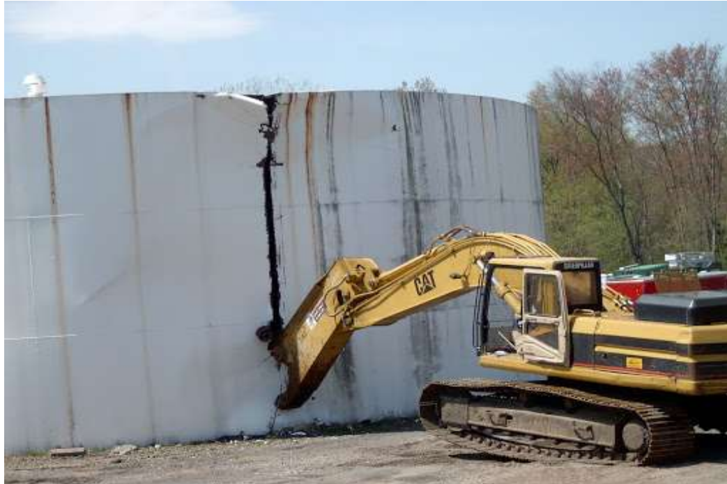
FIGURE 4-21 Typical excavator using shear attachment
