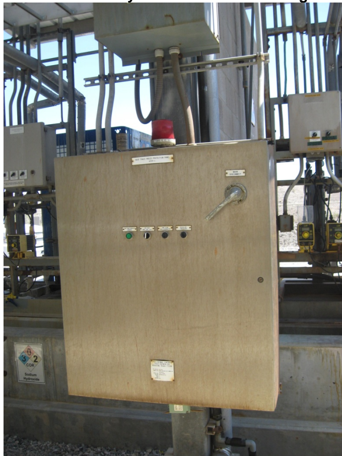
PHOTOGRAPH 46 Heat Trace Panel in Front of Chemical Storage Area
