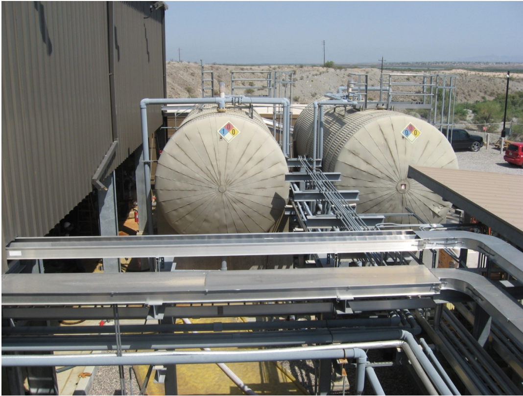
PHOTOGRAPH 37 Raw Water Storage Tank (Left) and Treated Water Storage Tank (Right)
