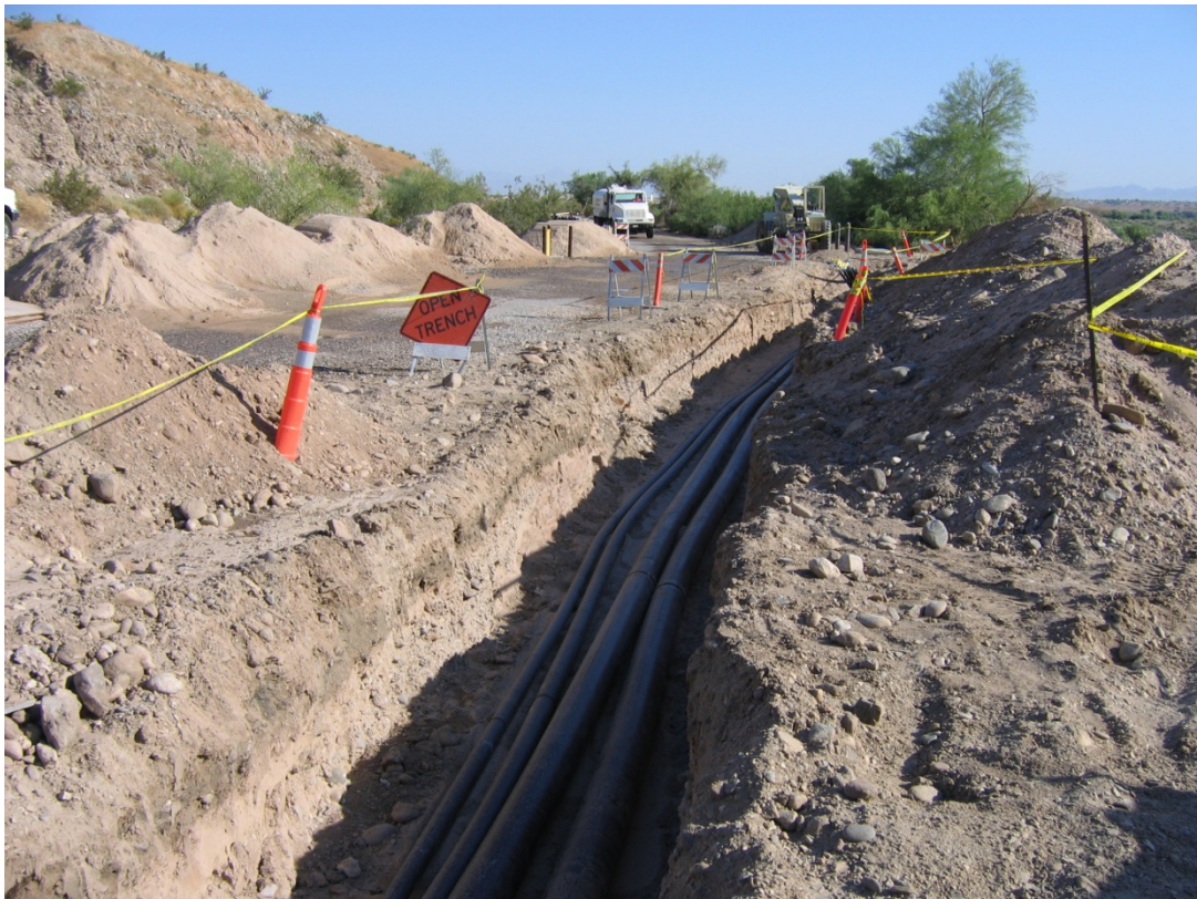
PHOTOGRAPH 8 Underground Double Contained Extraction Pipelines and Brine Pipes
