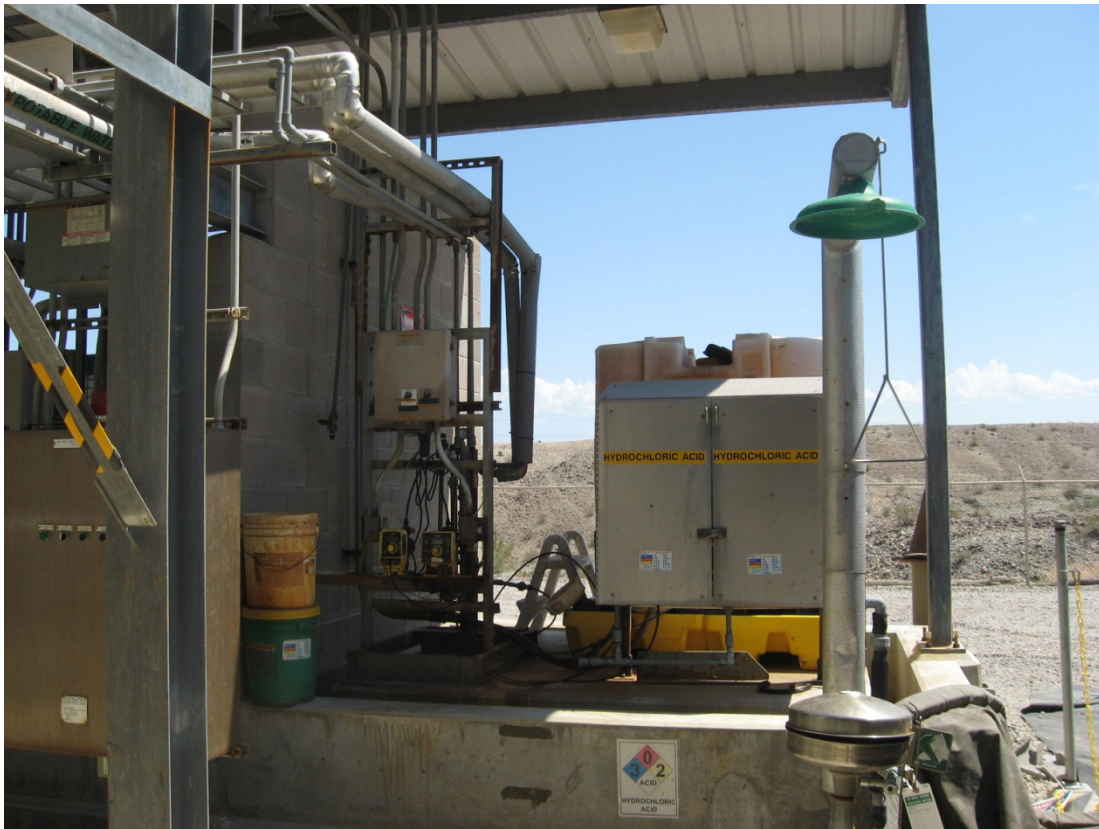
PHOTOGRAPH 43 Hydrochloric Acid System in Chemical Storage Area
