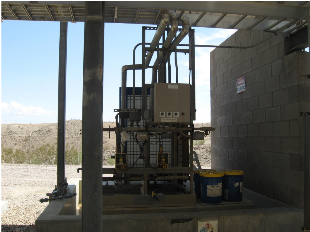
PHOTOGRAPH 44 Sodium Hydroxide System in Chemical Storage Area
