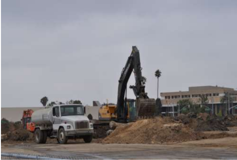
FIGURE 4-4 Typical water truck (left) and typical excavator with thumb attachment (right)
