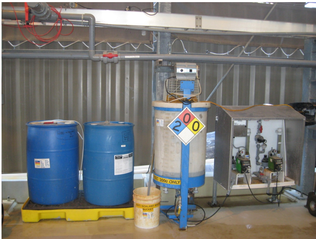
PHOTOGRAPH 48 Anti-scalant System Located Near Primary RO System
