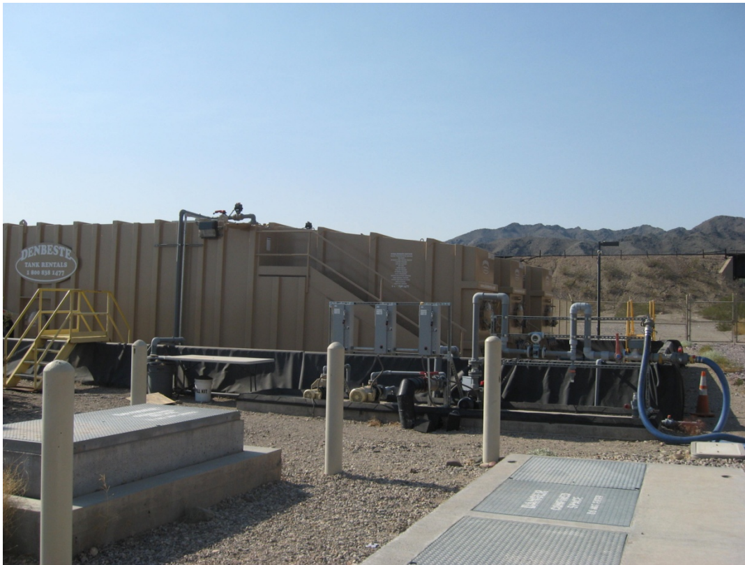
PHOTOGRAPH 62 Brine Storage & Loading System on MW-20 Bench Facility
