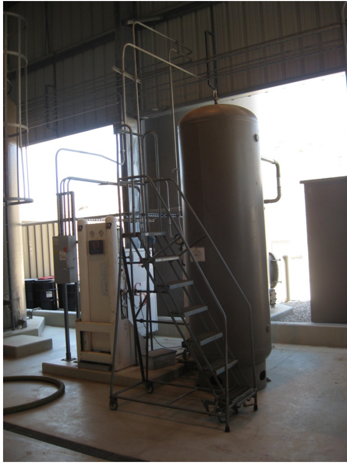
PHOTOGRAPH 41 Air Compressor and Dryer
