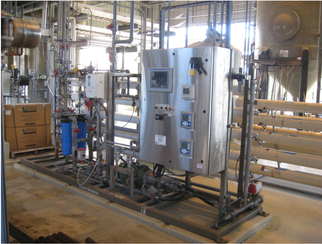
PHOTOGRAPH 31 Secondary RO System
