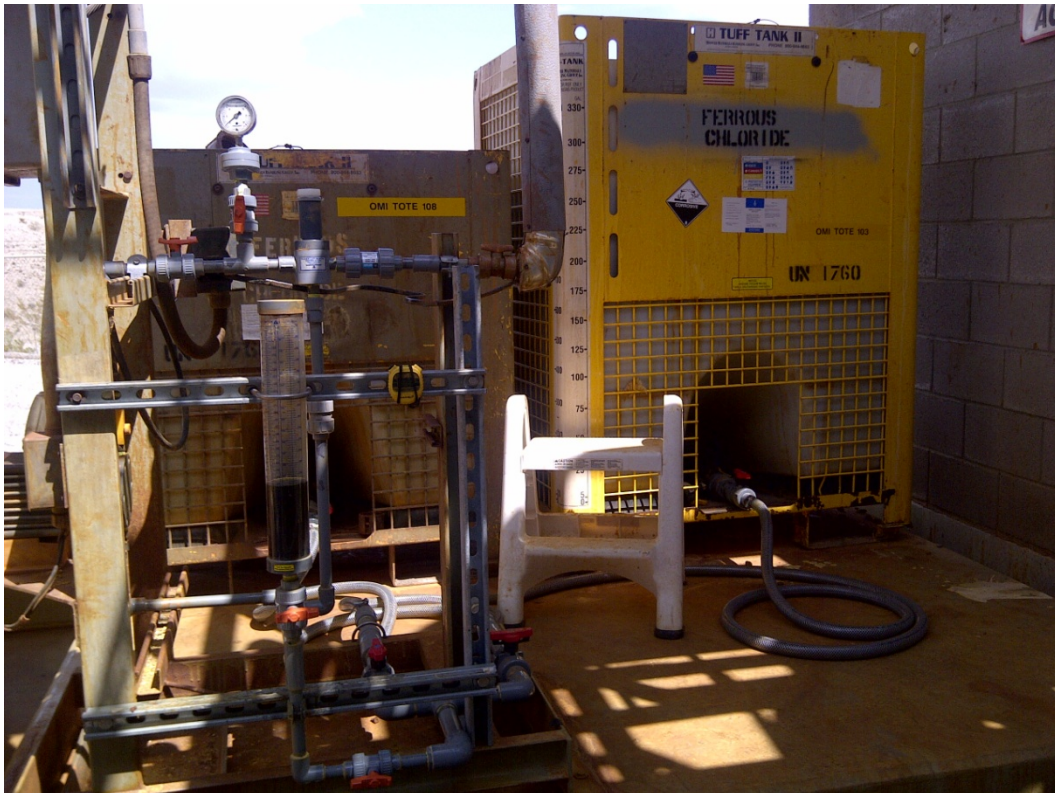
PHOTOGRAPH 45 Ferrous Chloride System in Chemical Storage Area
