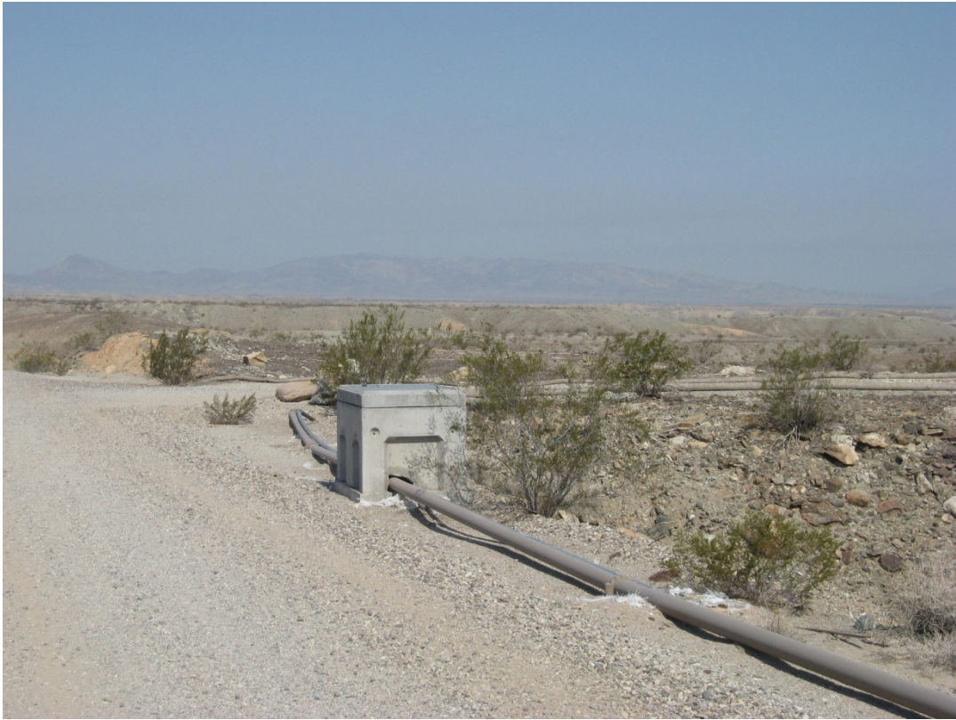
PHOTOGRAPH 57 Valve Vault Along Above Ground Injection Pipeline
