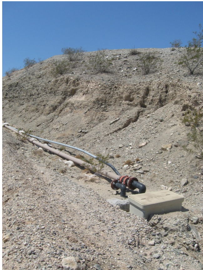
PHOTOGRAPH 56 Above Ground Injection Pipeline and Conduit
