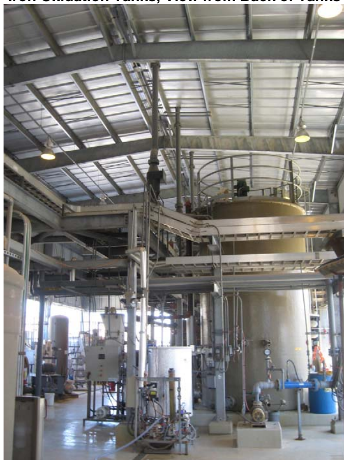
PHOTOGRAPH 20 Iron Oxidation Tank T-301C Side View
