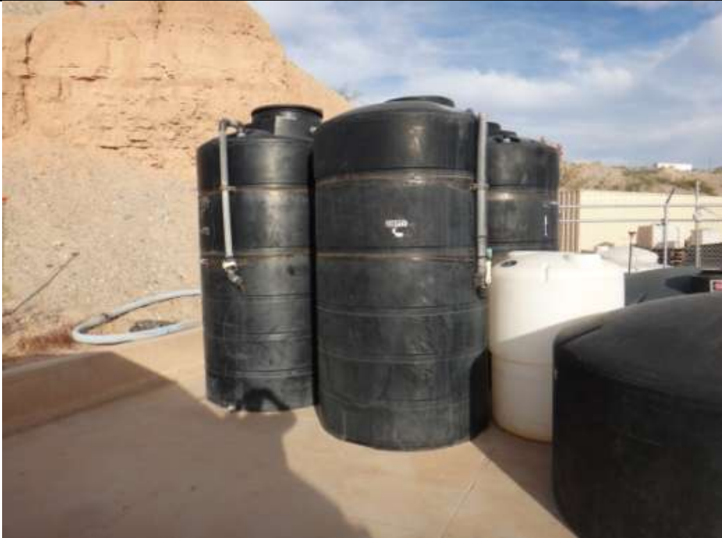
FIGURE 4-22 Typical water storage tanks (for dust control)
