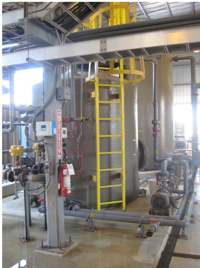
PHOTOGRAPH 32 RO Permeate Tank
