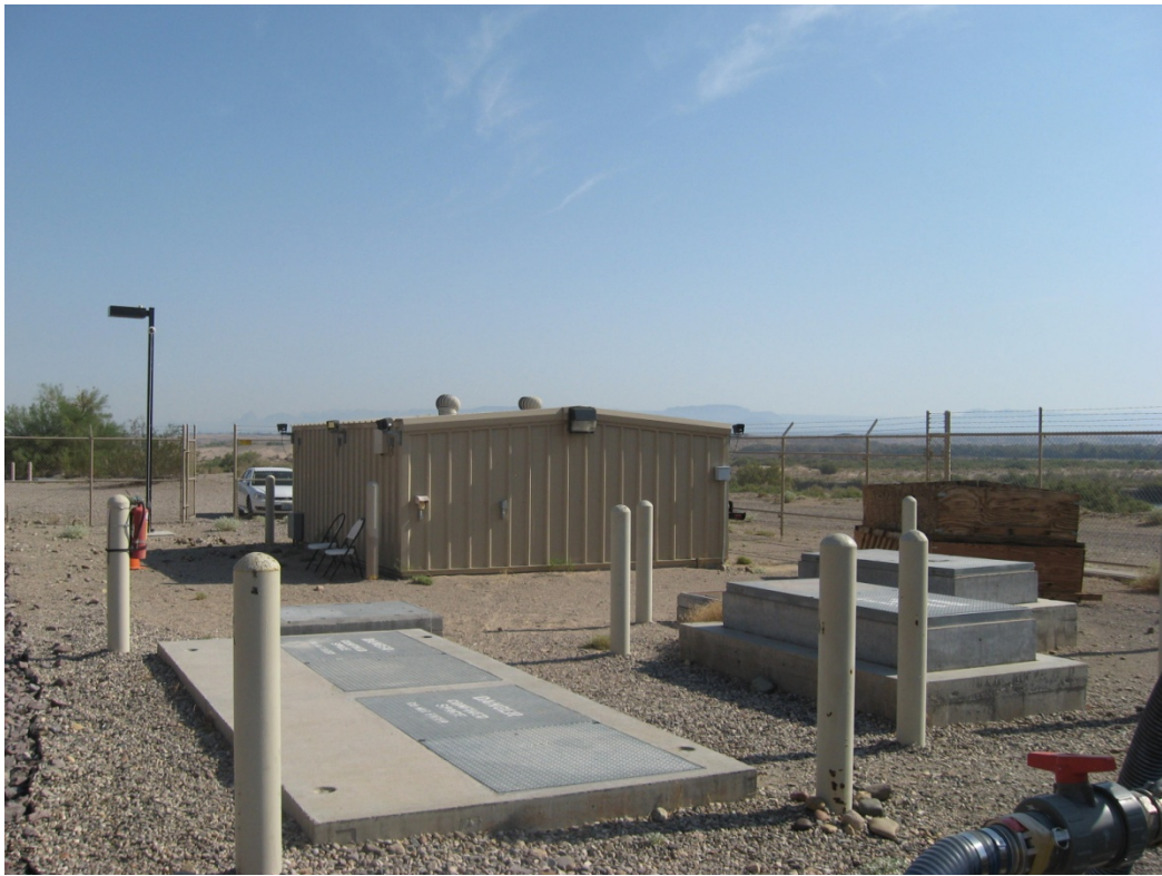
PHOTOGRAPH 2 Extraction Well Vaults Over TW-2S, TW-2D, & TW-3D and Valve Vault #1 on MW-20 Bench Facility
