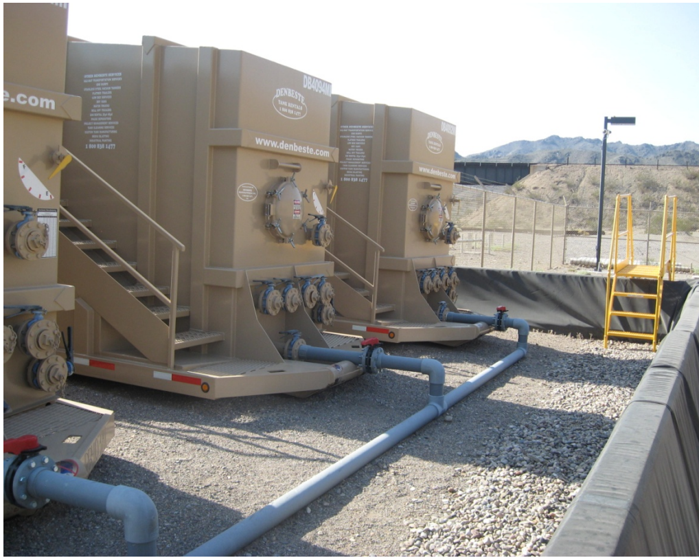
PHOTOGRAPH 63 Brine Storage and Loading System Secondary Containment
