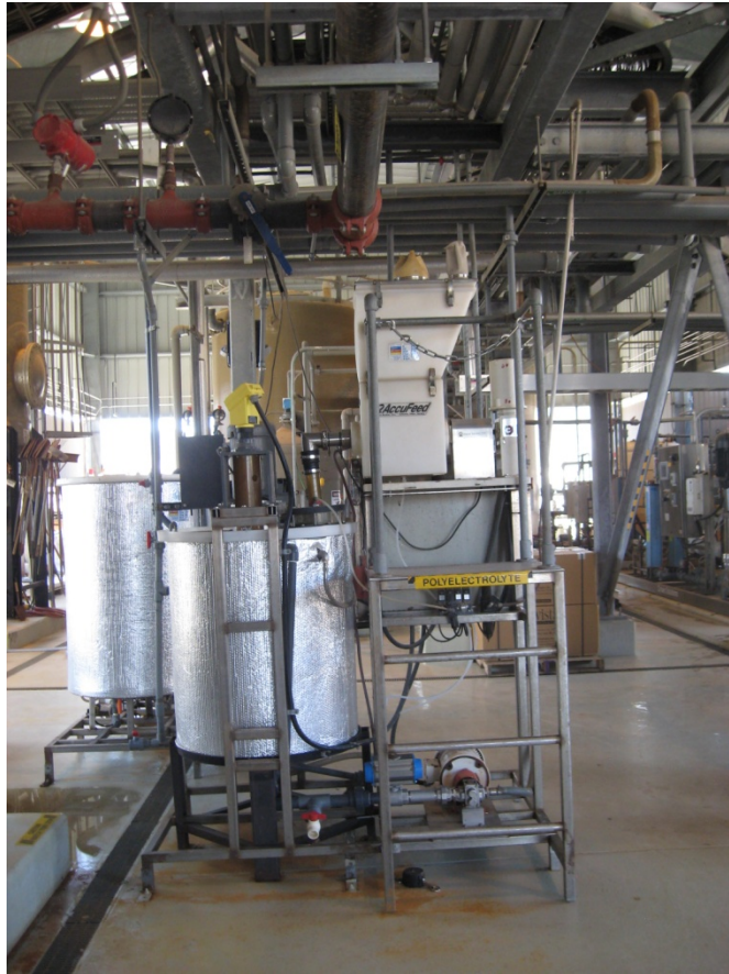
PHOTOGRAPH 47 Polymer System Located Near Iron Oxidation Tanks
